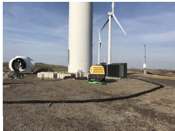
Photo 2: Typical work area with generator over temporary spill control containment.
