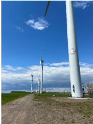
View looking northerly along access road.
