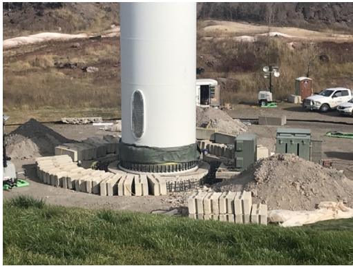
Photo 1: Typical Pre-Excavated Tower foundation with concrete block sidewalls.
