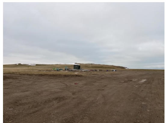
View of restored cap area of contractor trailer and equipment laydown area.
