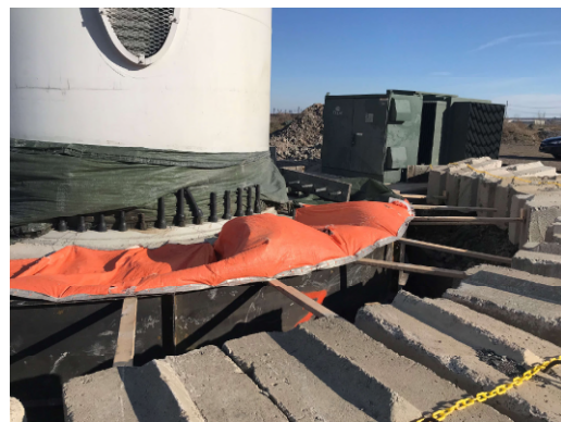
Photo 4: Turbine 5 with recently poured concrete within formwork.
