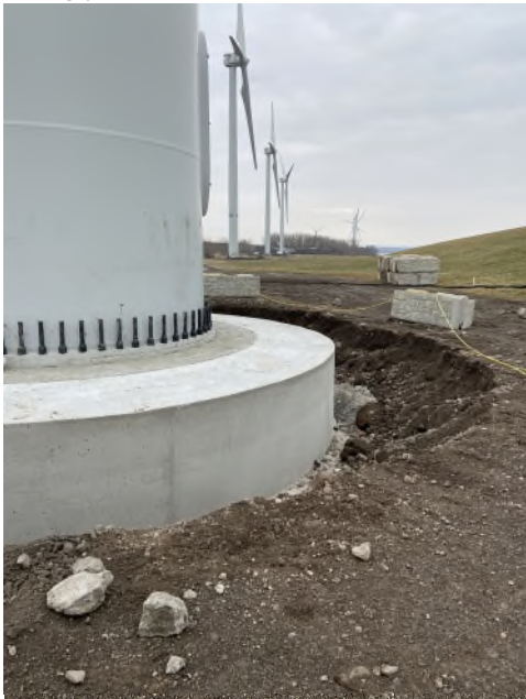
Photo 3: Turbine 4 with new poured foundation.
