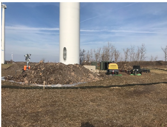
Typical view of foundation retrofit work area. Note erosion control wattle.
