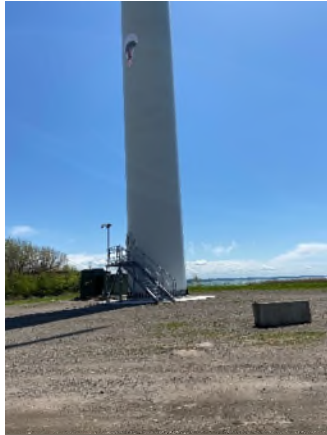
View of Turbine 1.
