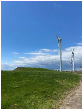
Typical view of grass covered cap.
