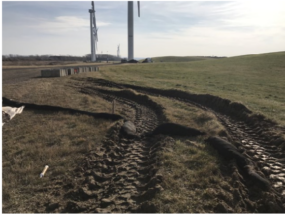
Photo 3: Typical rutting observed near Turbine 5. No wood chip demarcation material was observed.
