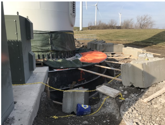
Photo 5: Turbine 6 with recently installed concrete and associated formwork.
