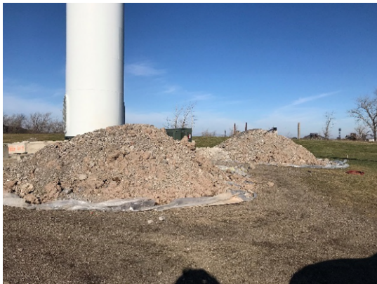
View of excavation spoil stockpile on plastic during foundation retrofit.
