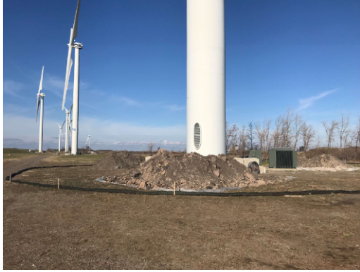
Photo 1: Typical Turbine work location with stockpile soil inside erosion control wattle.
