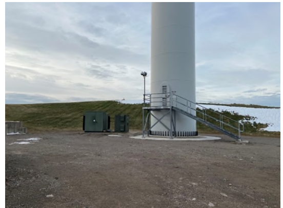
View of typical foundation retrofit area restoration.
