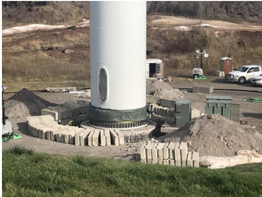
View of Turbine 8 foundation retrofit.
