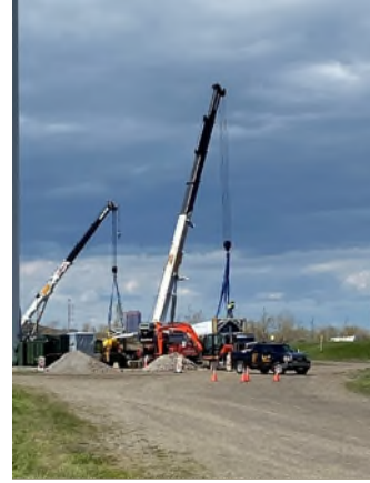
View of turbine blade unloading for upcoming repowering work.
