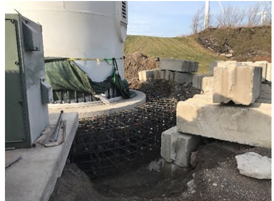
View of typical foundation retrofit rebar.
