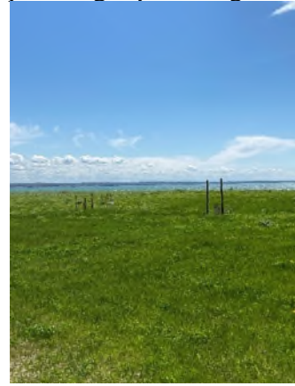
View of groundwater monitoring wells within grass covered cap area.
