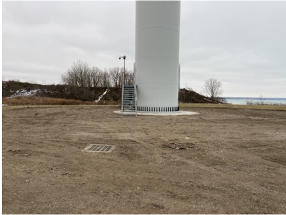
Photo 1: Completed Turbine 1 work location.
