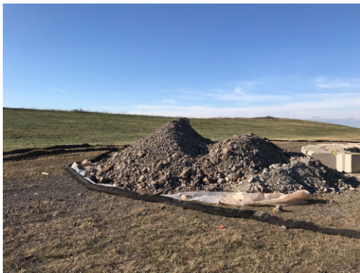
Photo 3: Typical foundation spoils on top of plastic sheeting.
