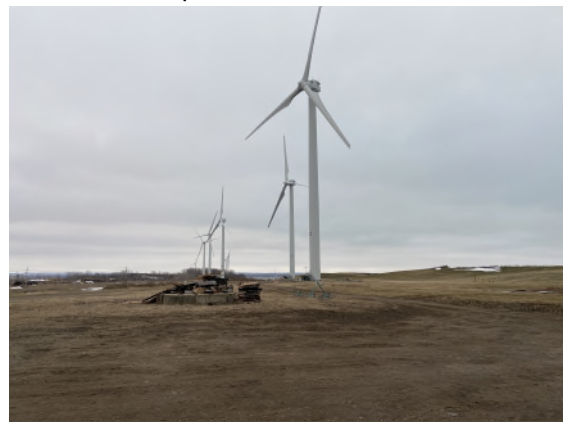
Photo 4: Former construction trailer area.
