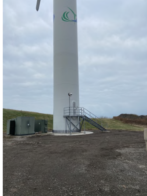
Photo 2: Turbine 8 foundation completed, backfilled and regraded.
