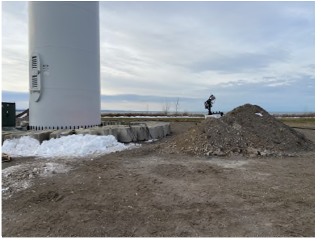
Photo 1: Turbine 1 work location with spoil pile.
