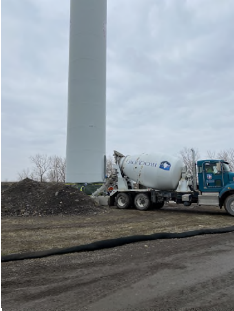
Photo 1: Turbine 2 work location with concrete being poured. Note erosion control wattle.
