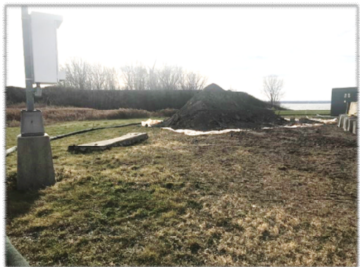
Photo 5: Excavation spoil on plastic, surrounded by erosion control wattle.
