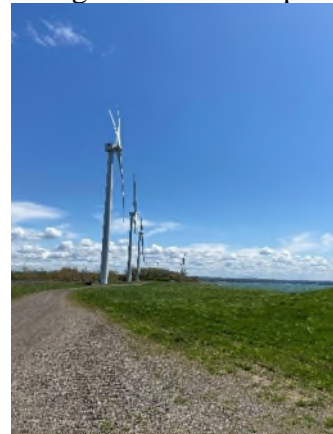
Southerly looking view of access road and grass covered cap.
