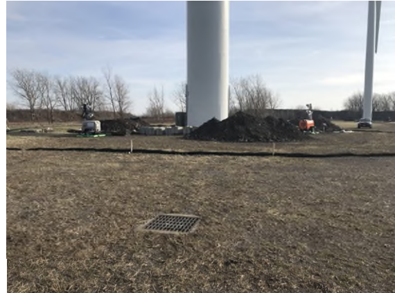
Photo 4: Typical storm drain catch basin located outside of designated work area.
