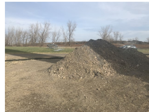
Photo 6: Excavation spoil not on plastic but surrounded by erosion control wattle.
