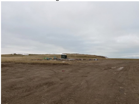
Photo 5: Former equipment laydown area.
