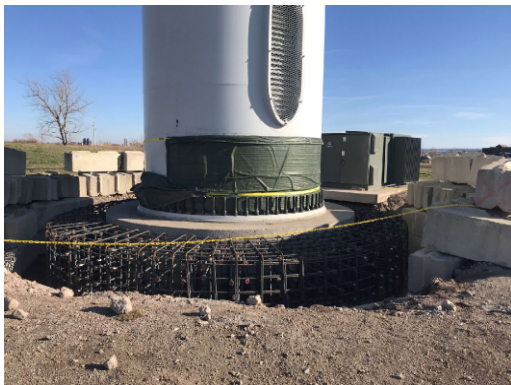
Photo 5: Turbine 6 with installed rebar ready for concrete pour.
