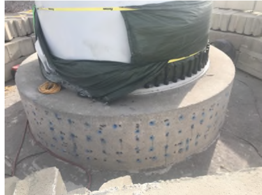
Photo 2: Typical foundation with drilled holes for steel dowel installation.
