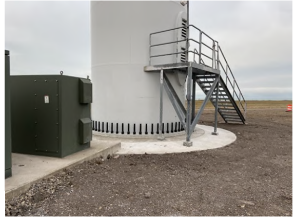
Photo 2: Completed Turbine 2 work location.
