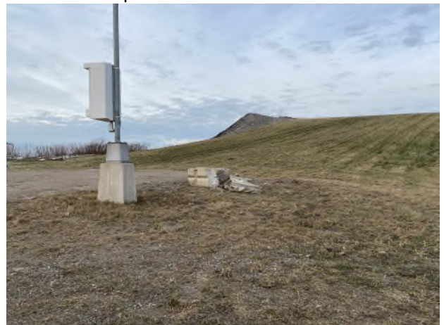
Photo 6: Former concrete slab requiring removal.
