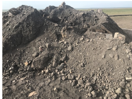
Photo 4: Excavation Spoil pile with fine and course grained Site fill material (brick, slag, etc.).
