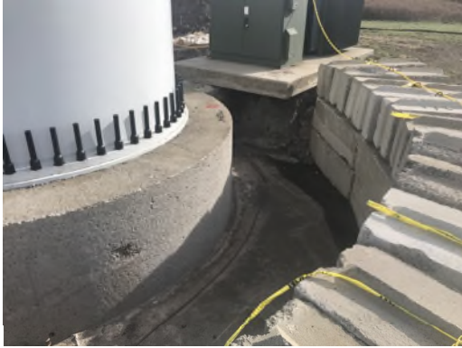
Photo 1: Typical Pre-Excavated Tower foundation with concrete block sidewalls.
