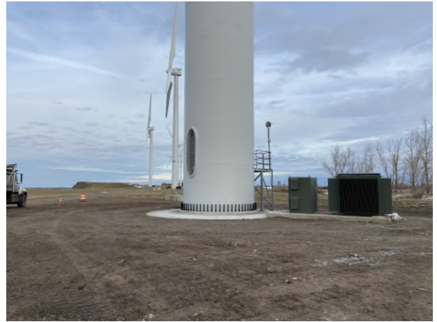
Photo 2: Turbine 2 completed and regraded.
