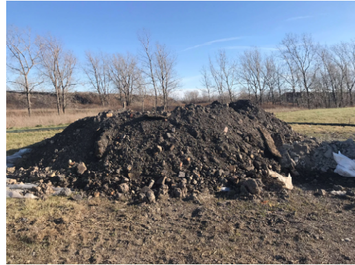
Photo 2: Typical foundation spoils on top of plastic sheeting.
