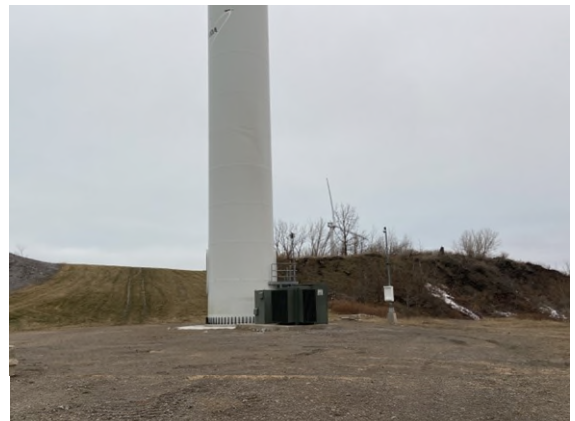
Photo 6: Completed Turbine 7 work area.
