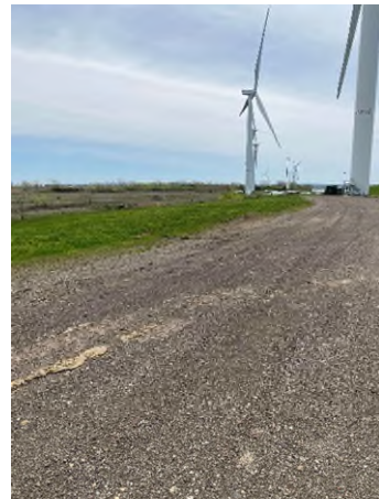
View looking southerly along access road.
