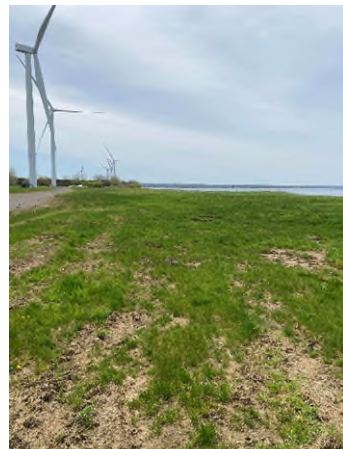
View of slight stressed grass cover in former construction staging area.
