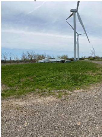
View looking southerly along access road.
