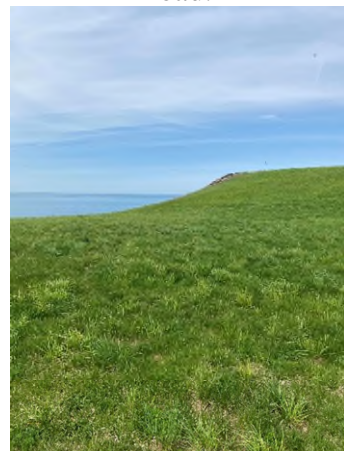
Typical view of grass covered cap looking northwesterly.
