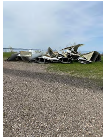
View of cut and stockpiled former turbine blades on ground surface.
