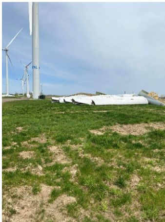
View of former turbine blades cut and stockpiled for removal.
