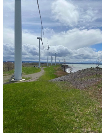
View of grass cover, access road and turbines looking south.
