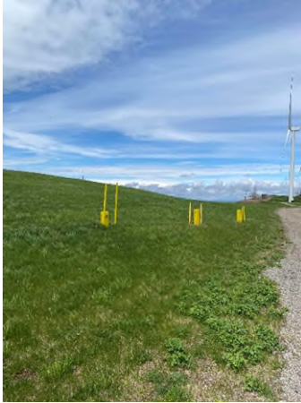
View of grassy cover system looking north.
