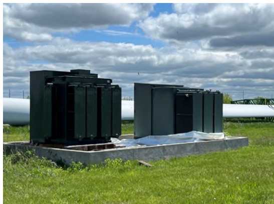
View of spare transformer storage in secondary containment (May 2025)
