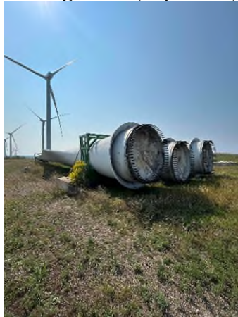
View of former turbine blades staged for removal (Sept 2024)
