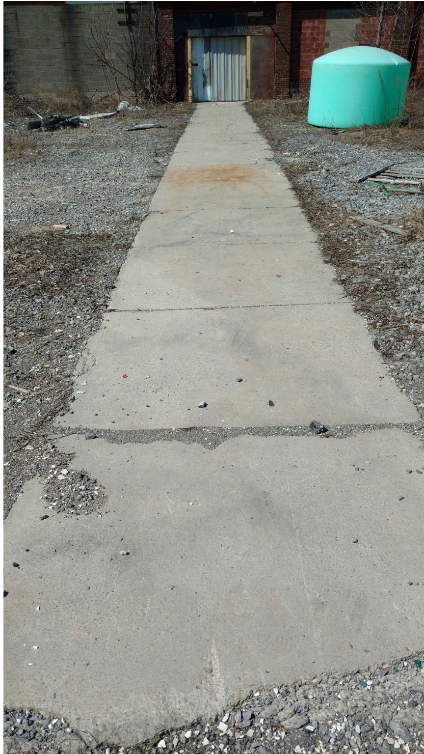
Concrete sidewalk, view toward Harrison Street Warehouse.
