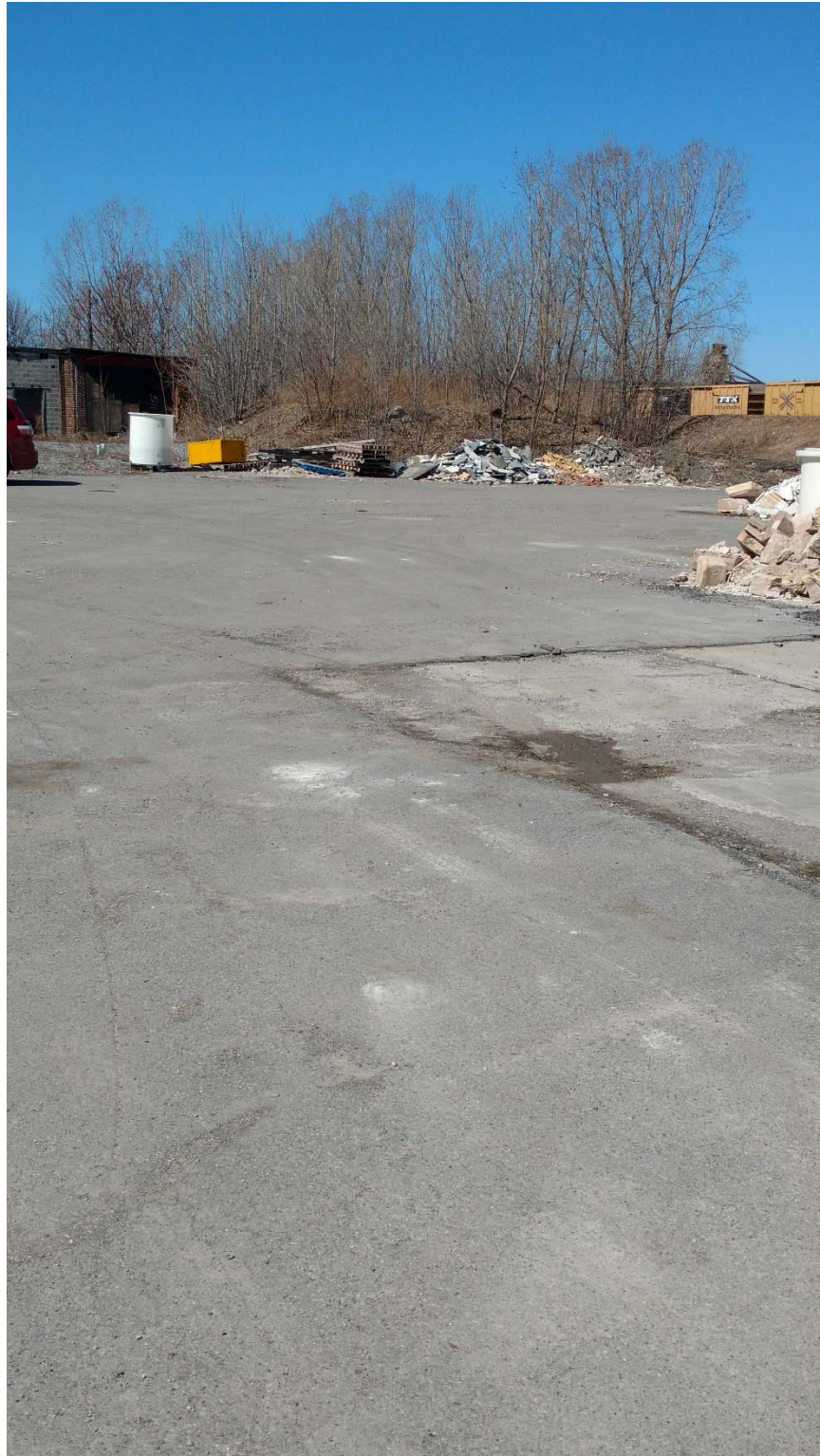
Asphalt cover system, view towards north.
