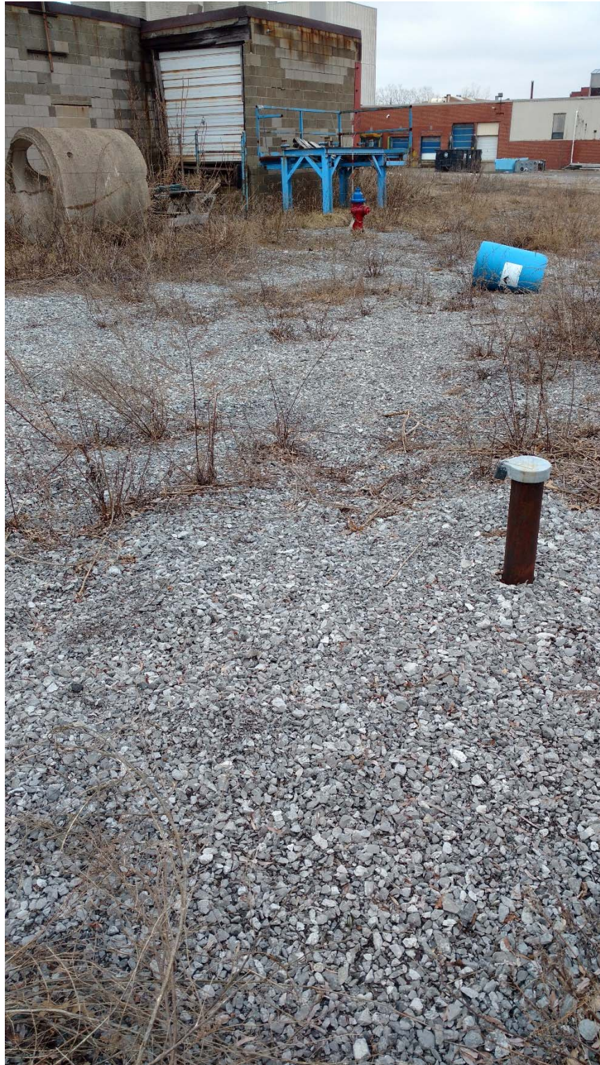
Area D stone cover system, view towards east.
