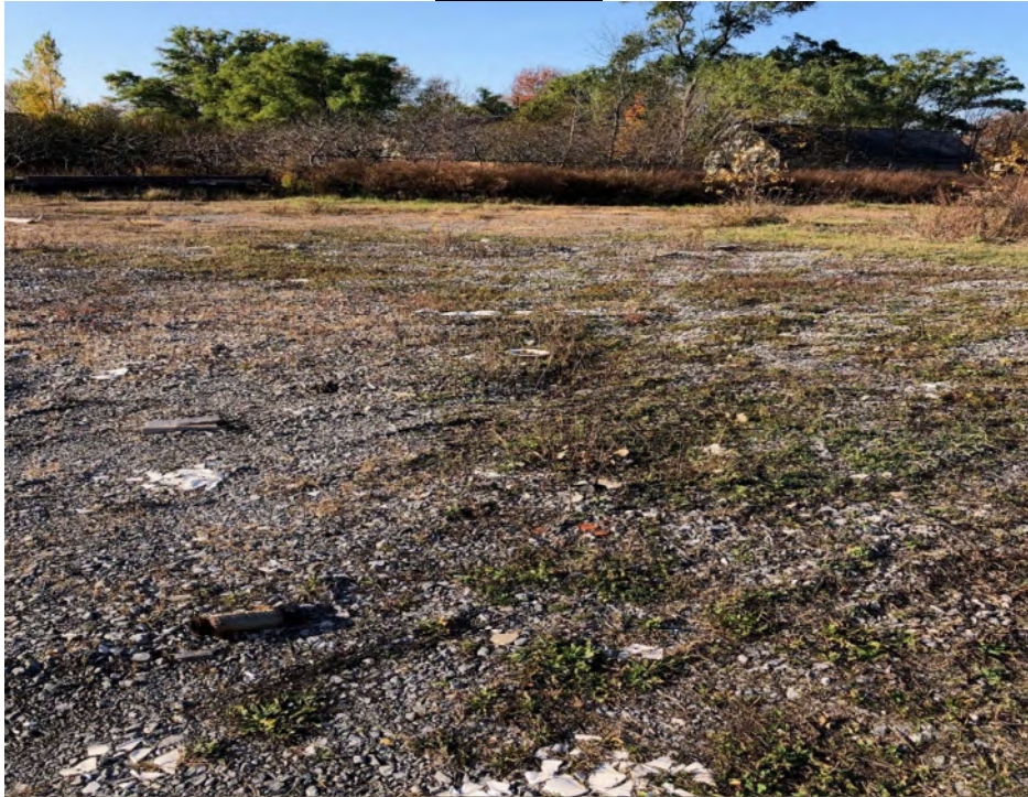
Area C stone cover system, view towards south,
