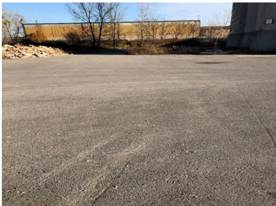
Asphalt cover system, view towards north.
