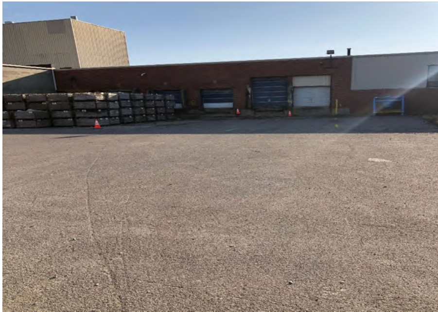
Asphalt cover system, view towards east.
