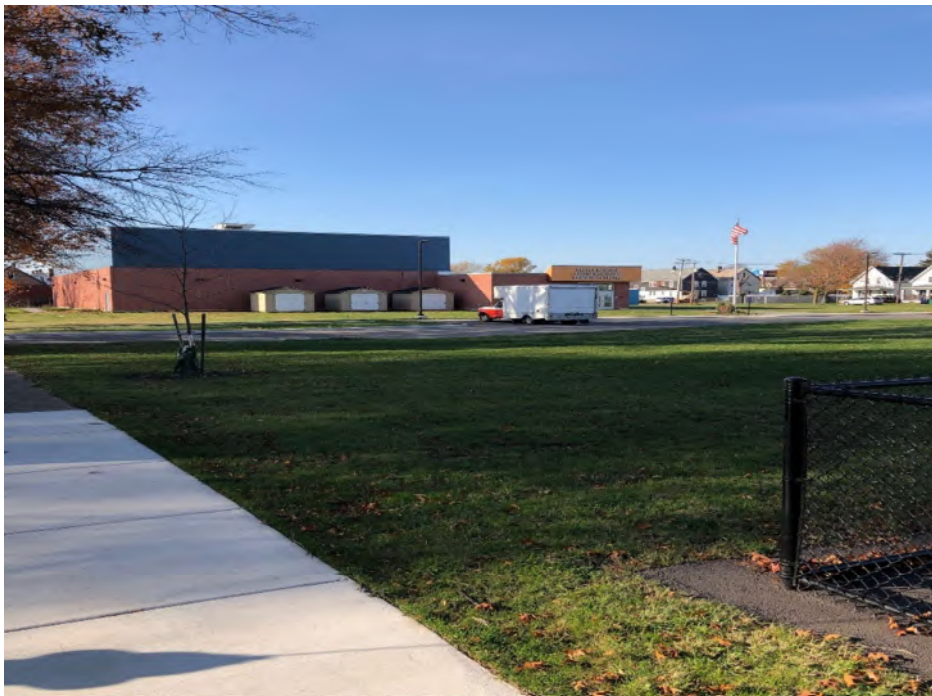
Vicinity of MW-22 and MW-22A that can no longer be located because of Community Center construction, view towards north.
