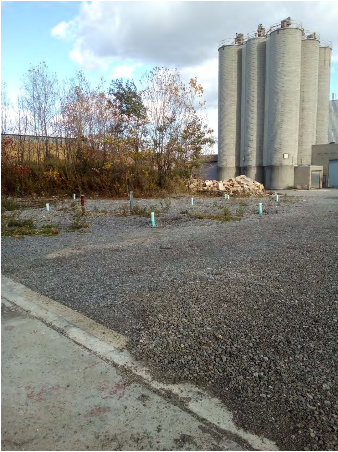
View towards injection gallery and monitoring wells MW-5R and MW-5AR.
