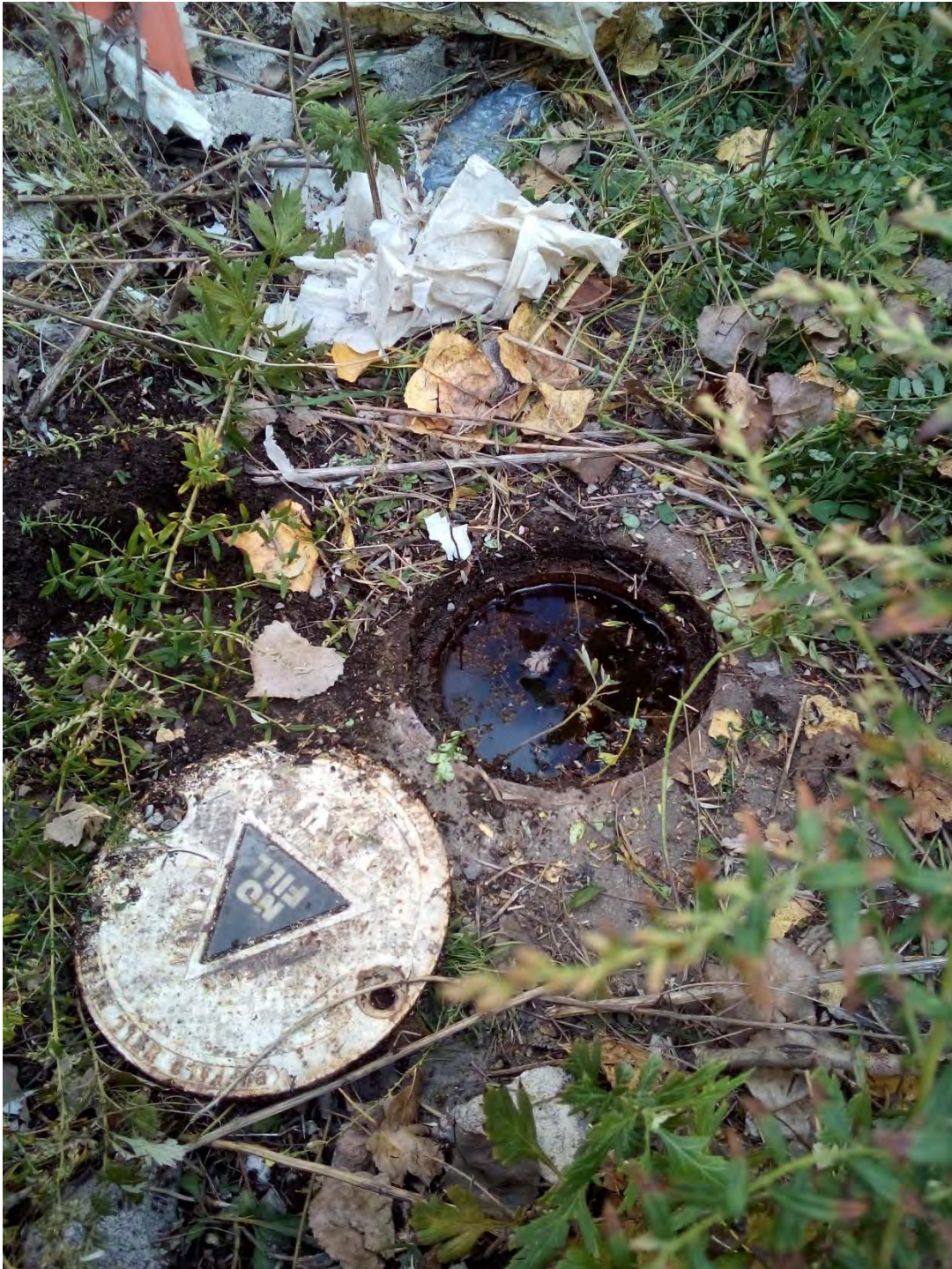
Flooded curb box at monitoring well MW-8.
