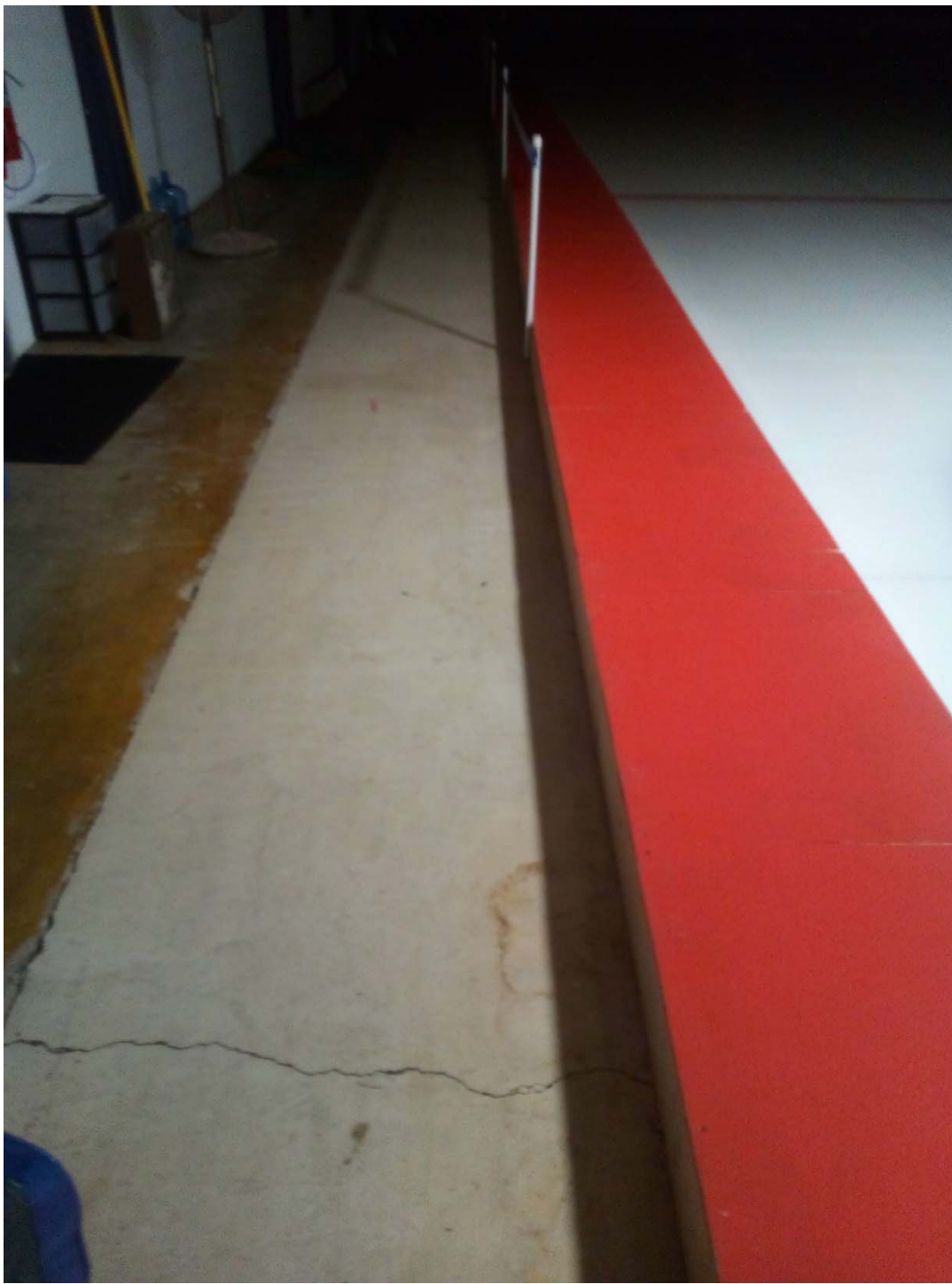
View of floor inside Buffalo Curling Club (ice area – left side).
