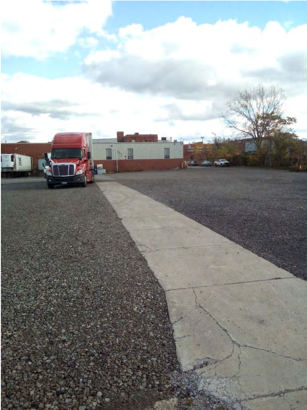
Asphalt cover system, view towards southwest.
