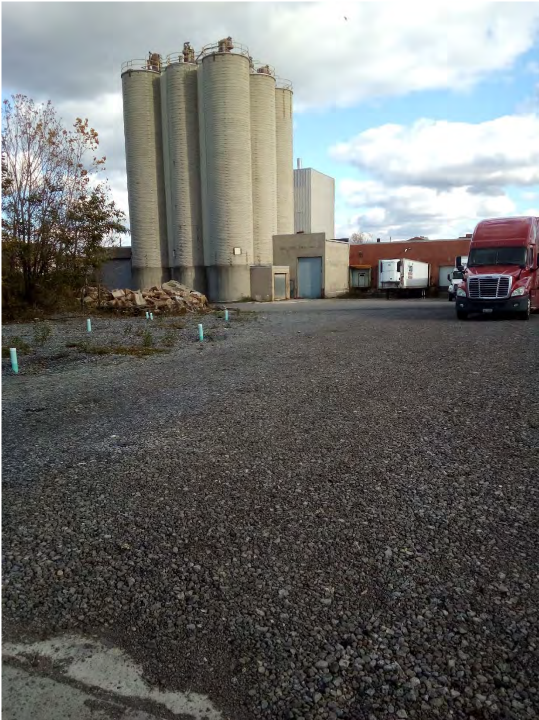
Asphalt cover system, view towards southeast
