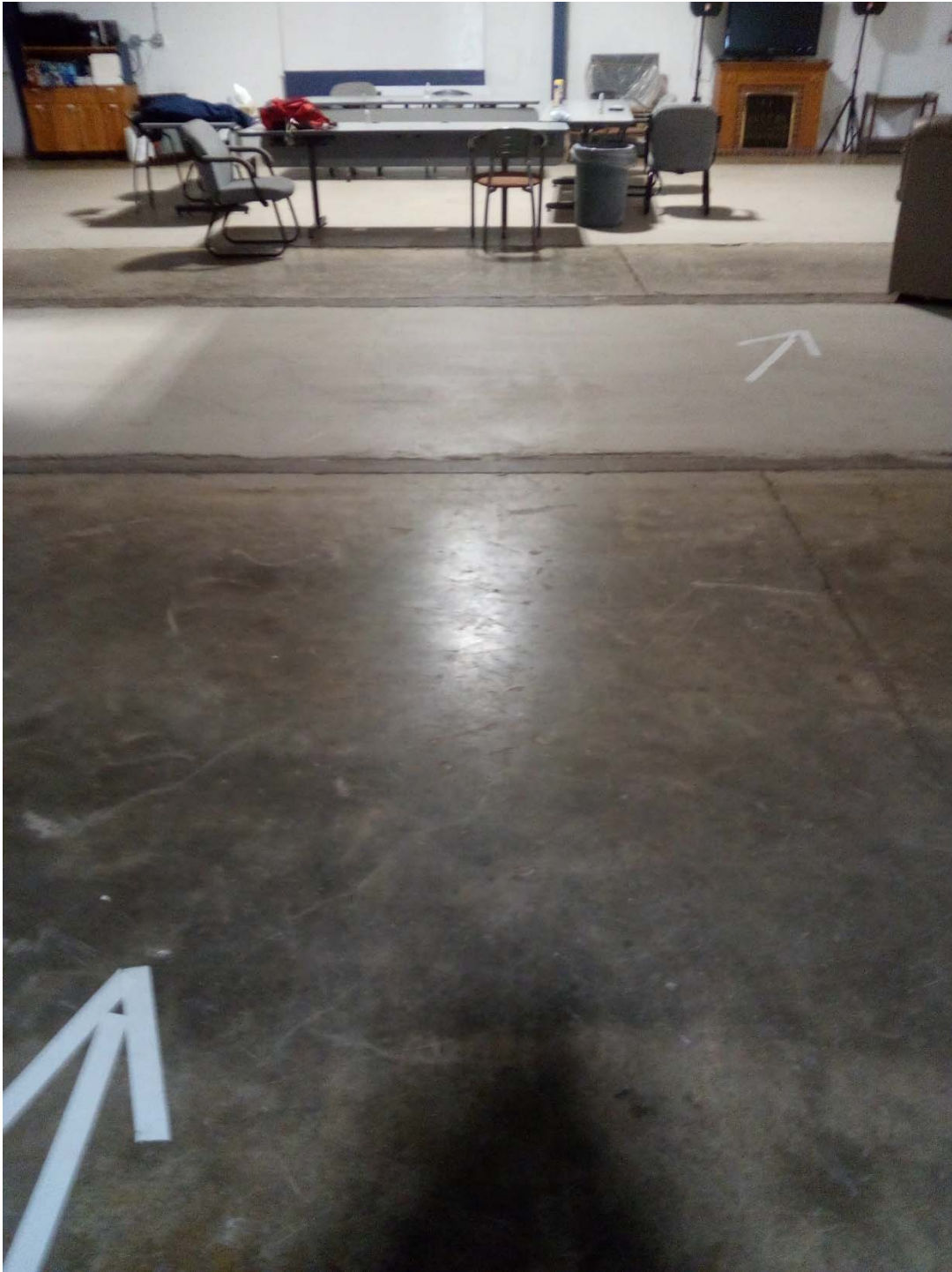
Concrete floor in lounge area of Buffalo Curling Club.
