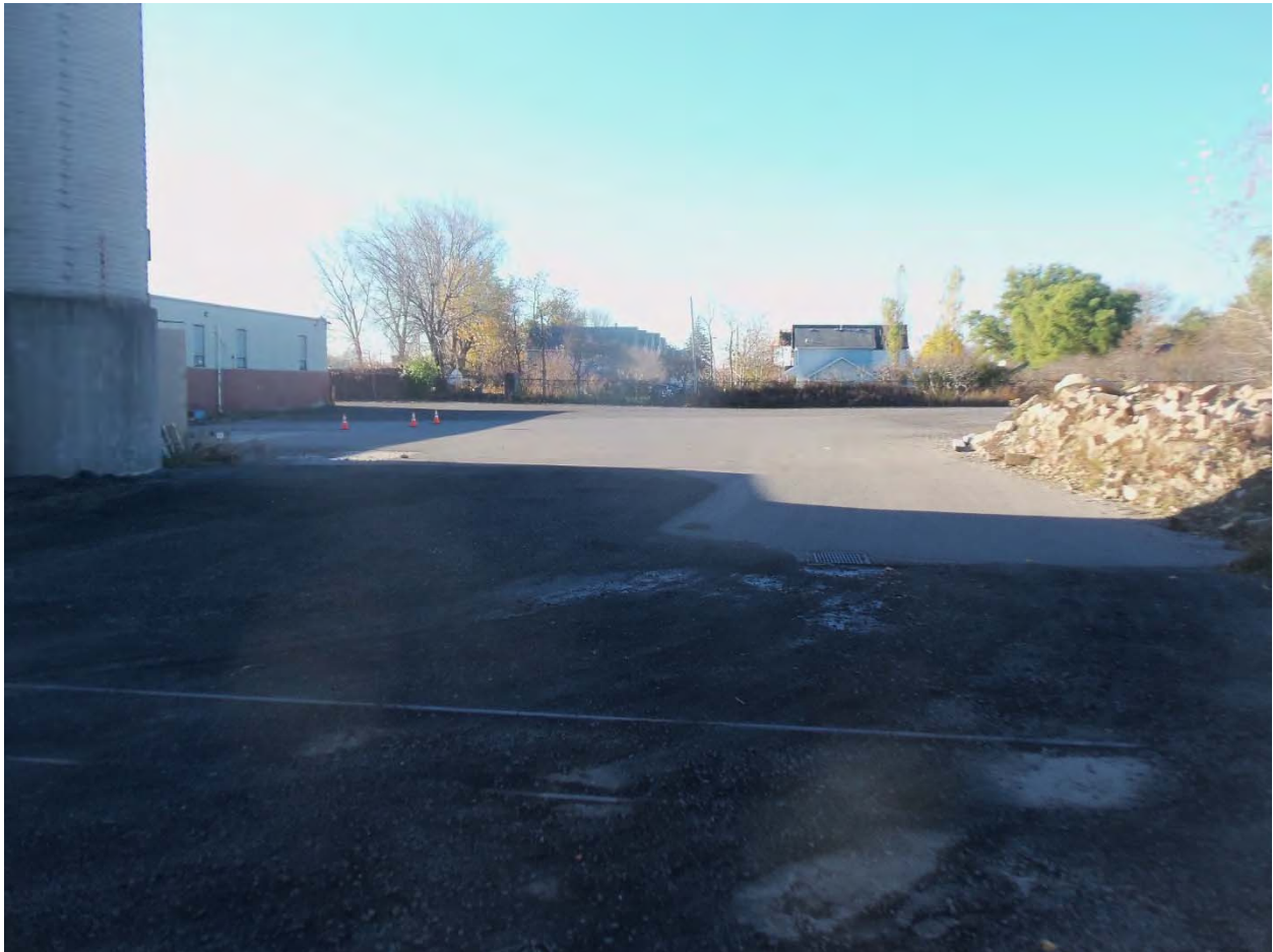
Transition from gravel to asphalt cover system, view towards southwest
