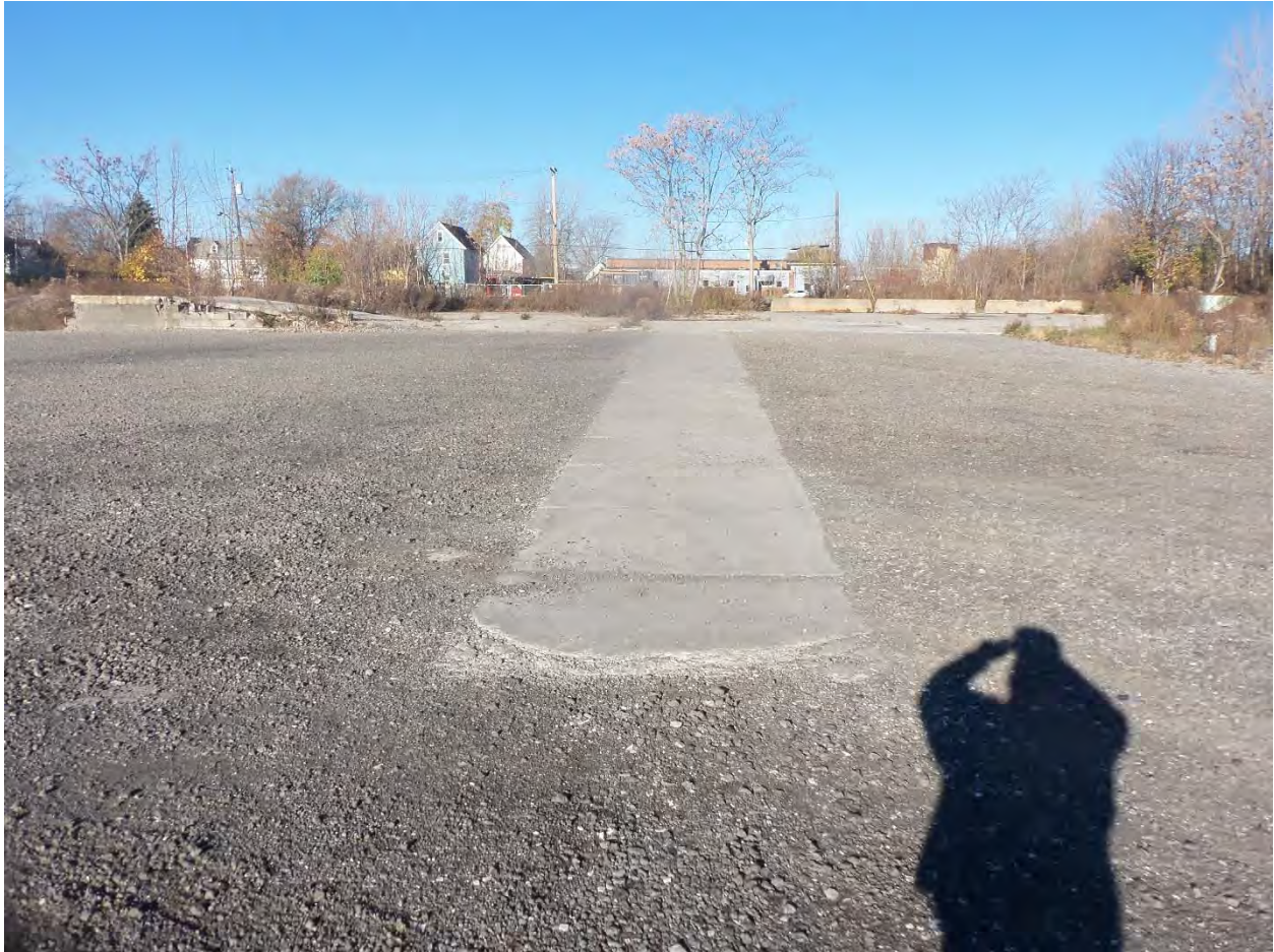
Concrete and stone cover systems, view towards northwest.
