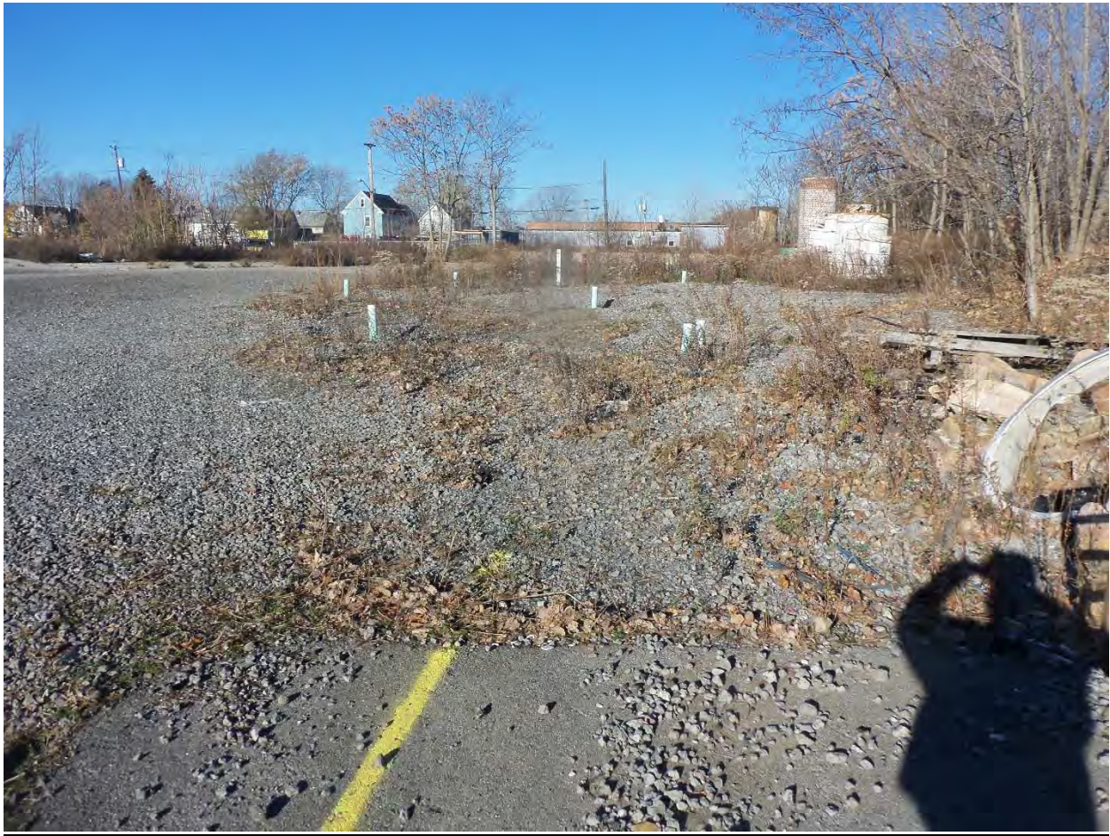
View towards injection gallery, monitoring wells MW-5R and MW-5AR, and concrete floor of former warehouse.
