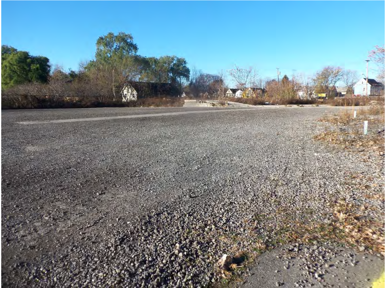
Stone cover system and concrete cover system, view towards southwest.
