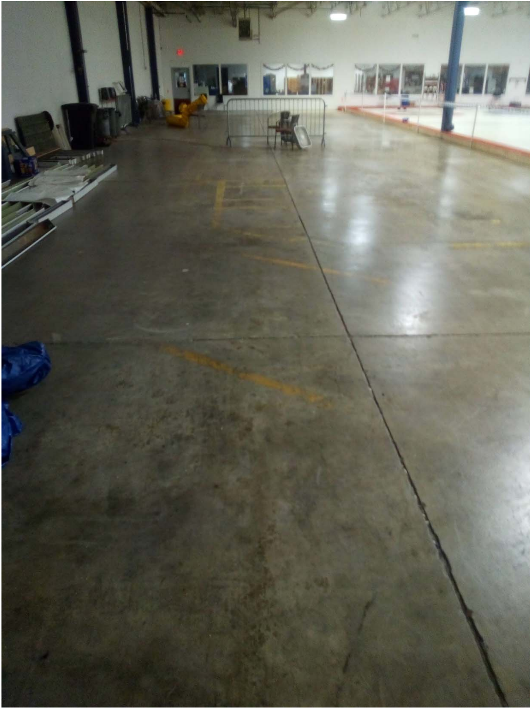
View of floor inside Buffalo Curling Club (ice area – south side).
