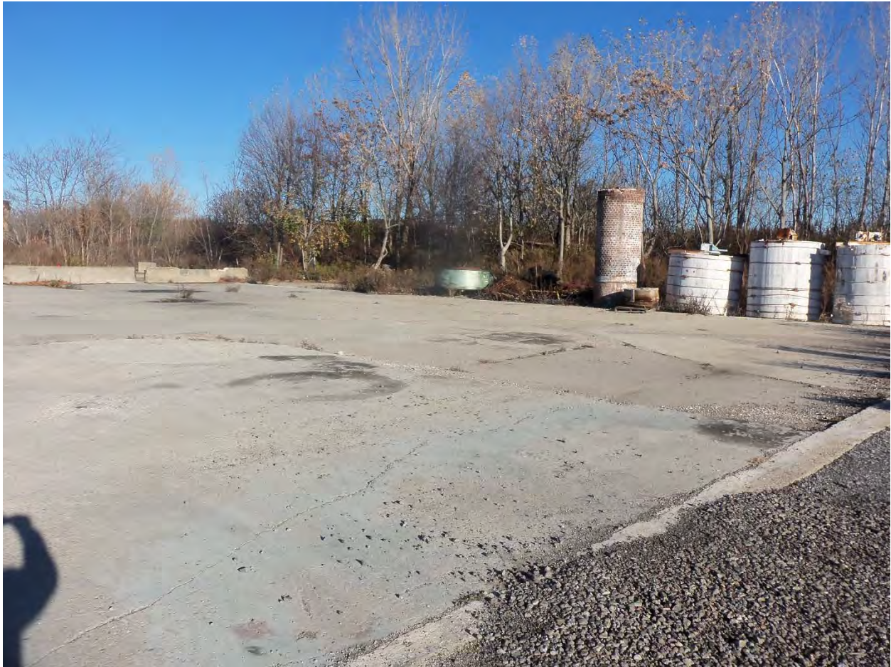
View of concrete floor of former warehouse building.
