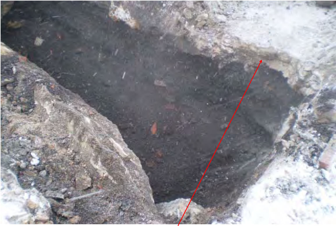
Test Pit 3 looking west standing at northeast corner, 8" thick concrete slab is shown
