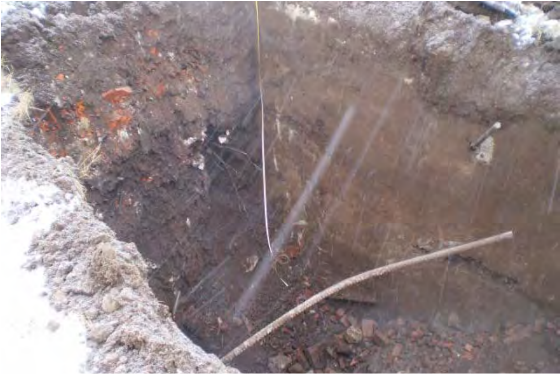
Looking west, concrete foundation wall along western edge of pit. Potential retaining wall tie back in center of picture.
