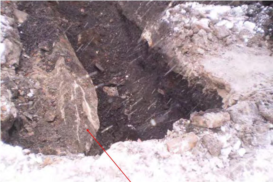
Test Pit 3 looking south, concrete footing on east side of pit, 3.5' thick
