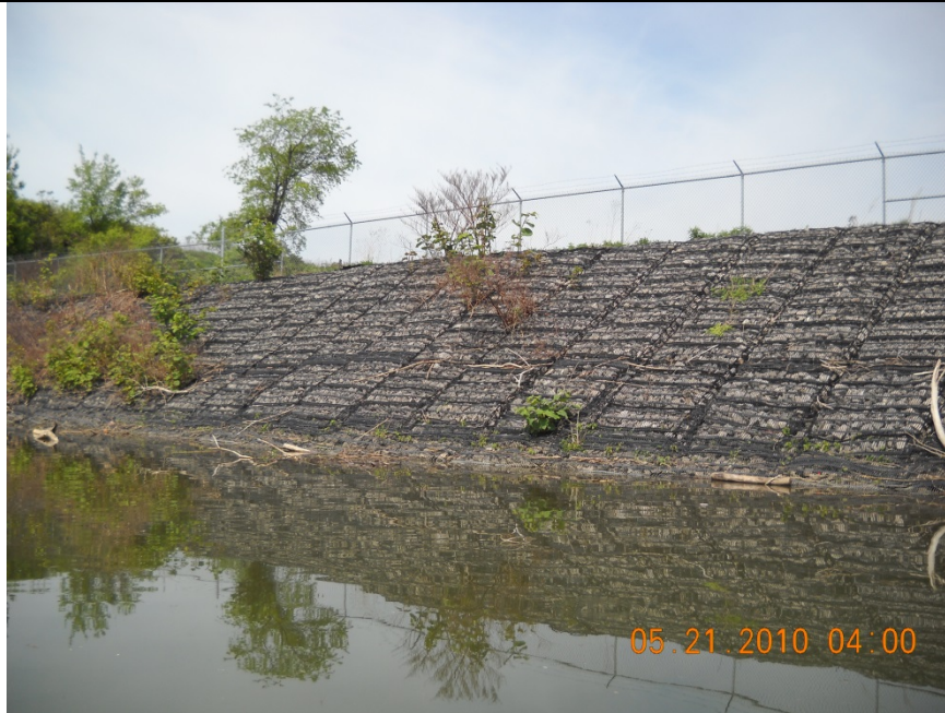
Photo 1: Marine mattress segment at Area A
