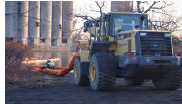
4 Removing turbidity curtain from the river at Ensign St.
