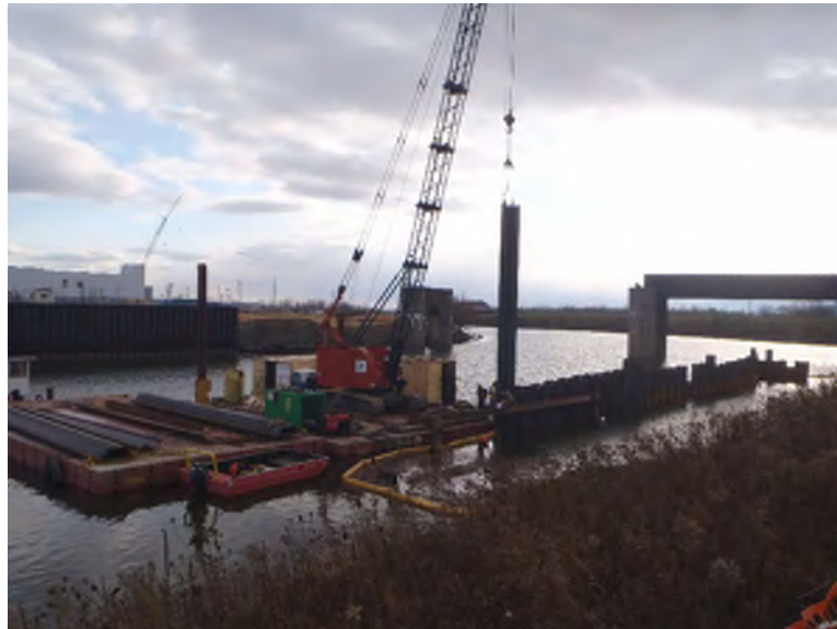
Photograph 2 Knee Wall Installation – DMUs 9 and 10
