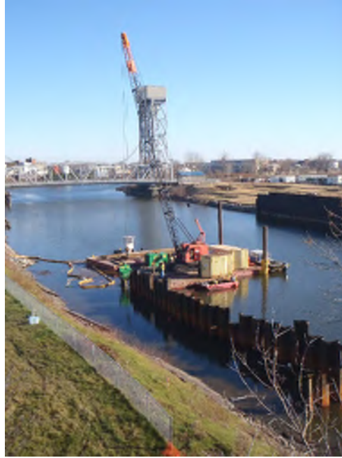
Photograph 1 Knee Wall Installation – DMUs 9 and 10
