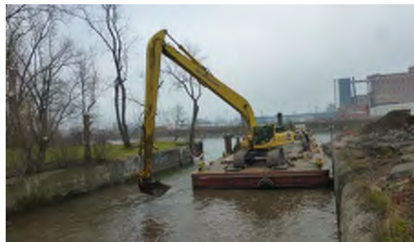
1 Armor stone capping at DMU 44E.
