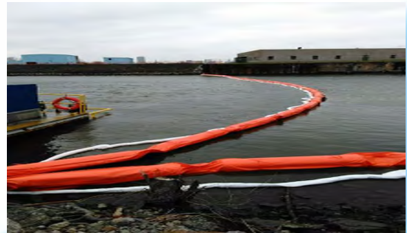
4 Turbidity curtain and oil boom installed upstream of DMU's 9 and 10.
