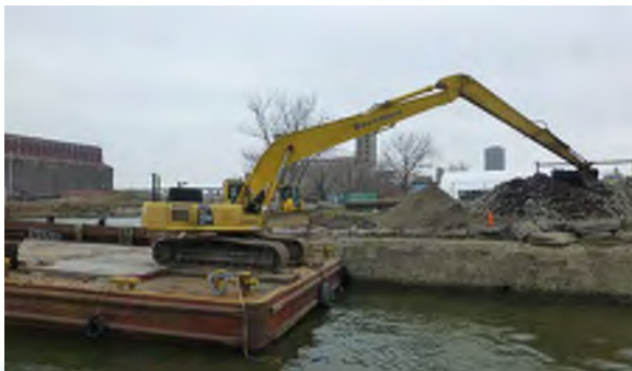
5 Armor stone capping operations at DMU 44E.
