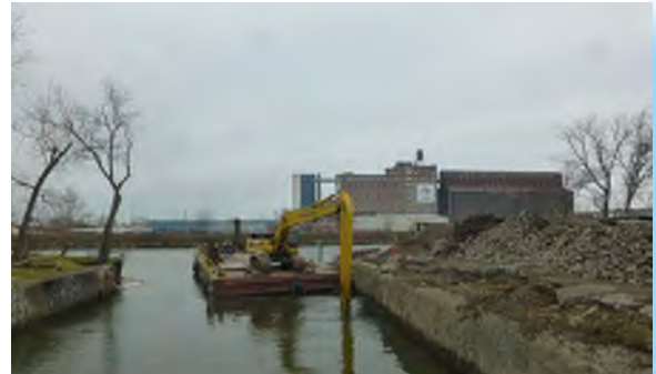
2 Armor stone capping operations at DMU 44E.
