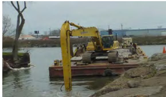
1 Capping operations at DMU 44E.
