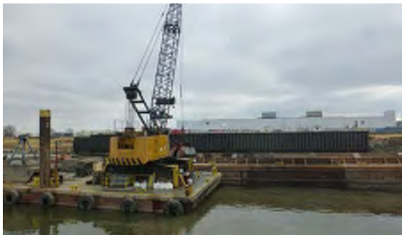
3 Loading dredged material into scow.
