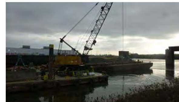
6 Sediment removal in DMU's 9 and 10.
