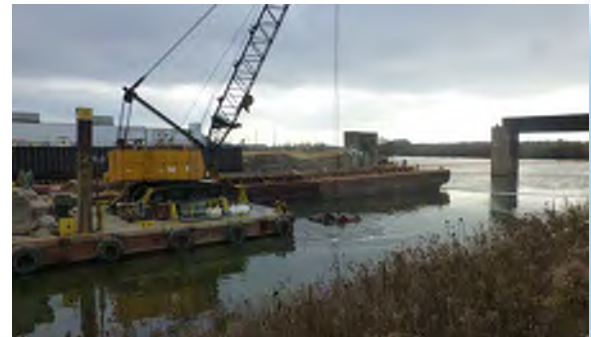
2 Sediment removal in DMU's 9 and 10.
