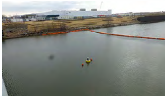
1 Turbidity buoy, curtain, and oil boom in place at DMU's 9 and 10.
