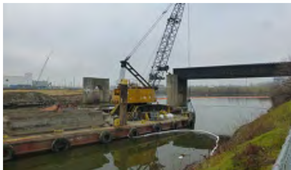
3 Sediment removal operations in DMU's 9 and 10.
