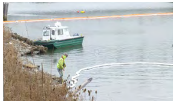
5 Luedtke adjusting oil boom at DMU's 9 and 10.
