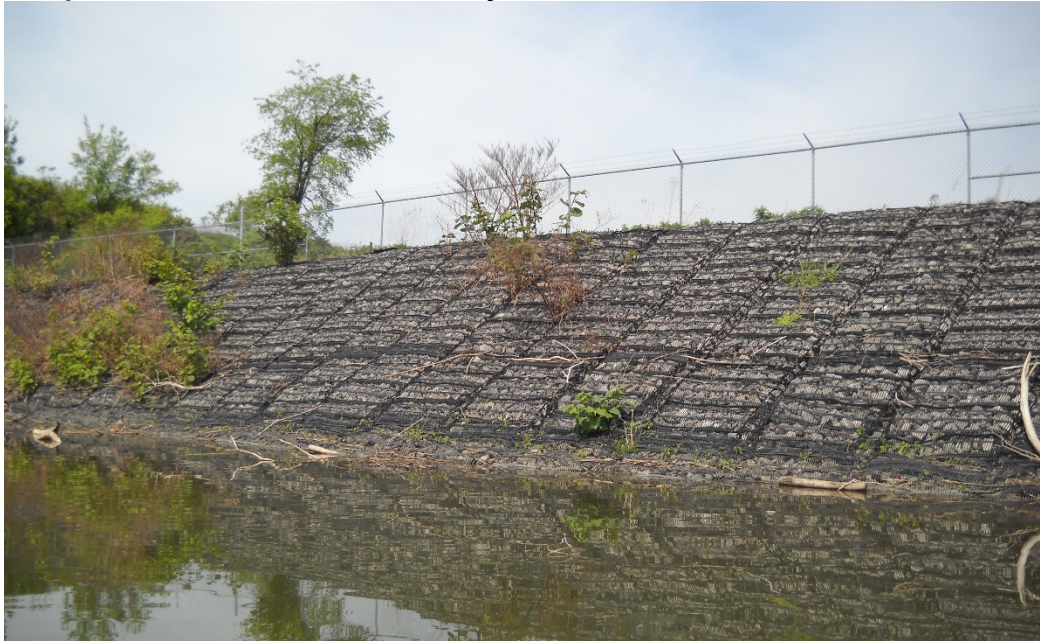
Figure 3 Completed Marine Armor Mattress System
