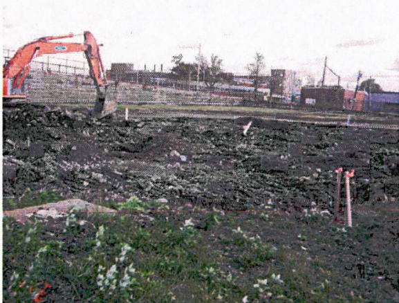
Removal of overburden at C2
