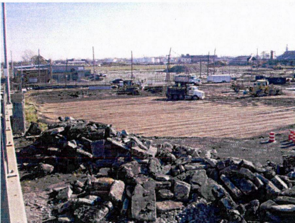
Final backfilling and compaction of C-2 excavation
