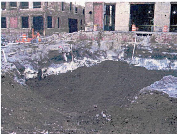
Area C-1 excavation backfill first lift
