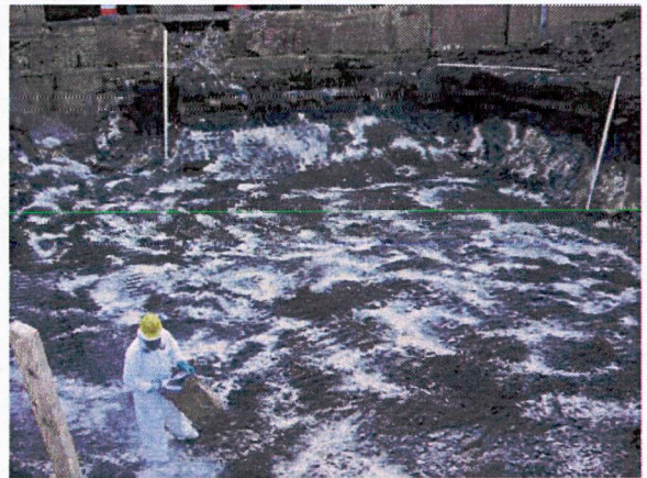
Applying ORC - A to C1
