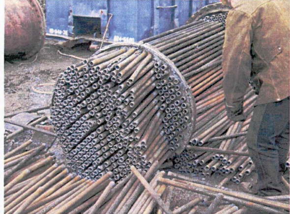
Exchanger tube bundles cut for recycling
