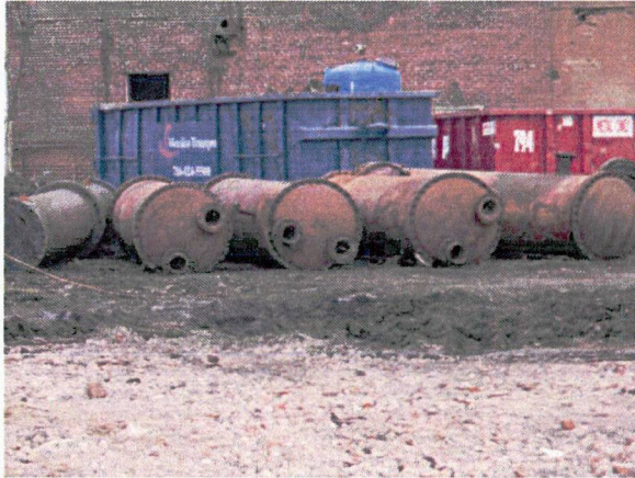
Heat exchangers removed from Area C roof
