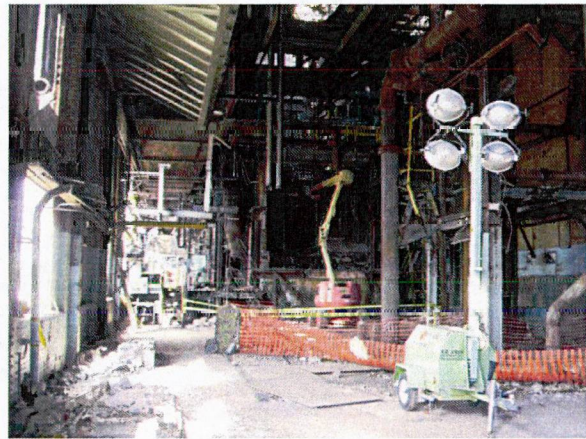
Area C continued boiler removal
