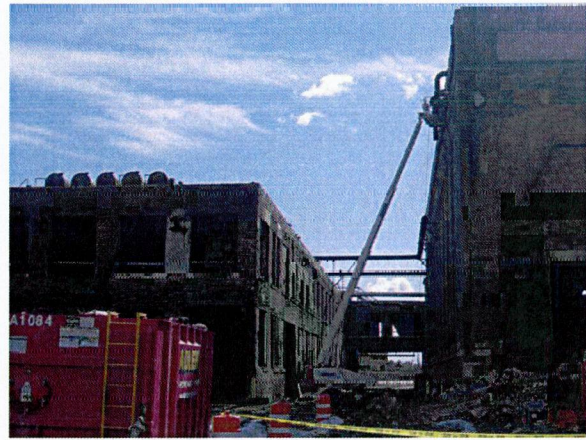
Area C exterior pipe removal
