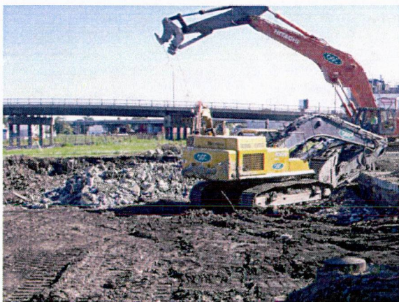
No.6 oil secondary containment demolition
