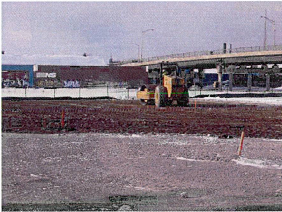
Compaction with drum roller
