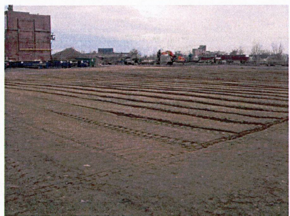
C-2 excavation backfill and compaction complete
