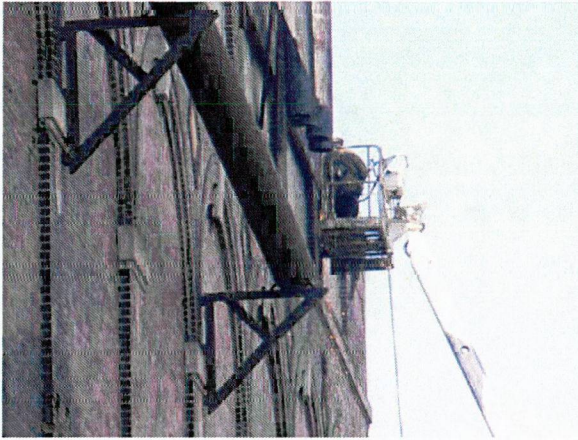
Area C exterior pipe removal
