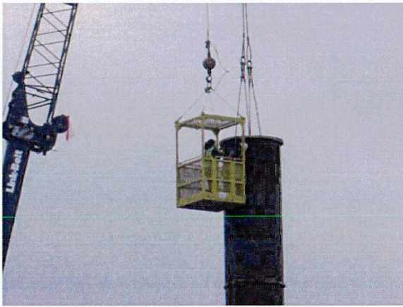
Prepping for stack removal
