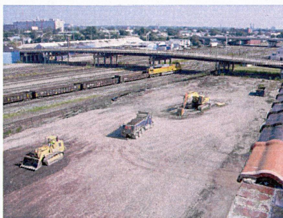
No.6 oil secondary containment final grade
