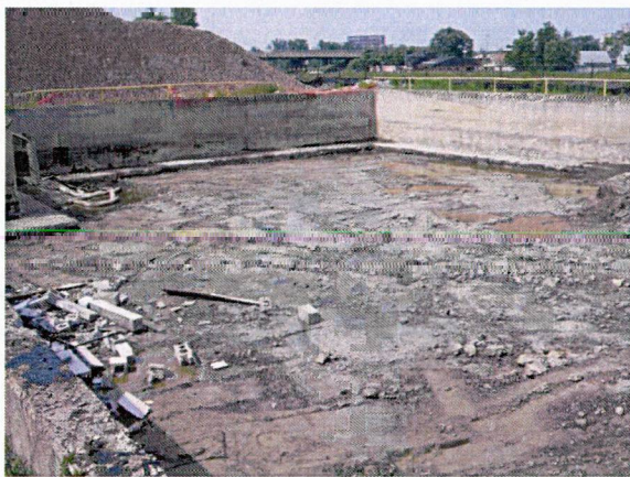
No.6 oil secondary containment remediation
