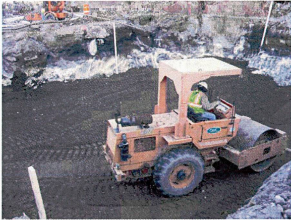
Backfill compaction at C1
