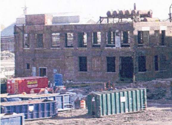
Area C Bldg.223 gut out complete Roof top equipment to be removed by crane
