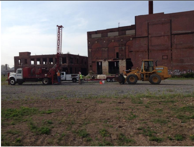
Area C ORC Borehole Installation
