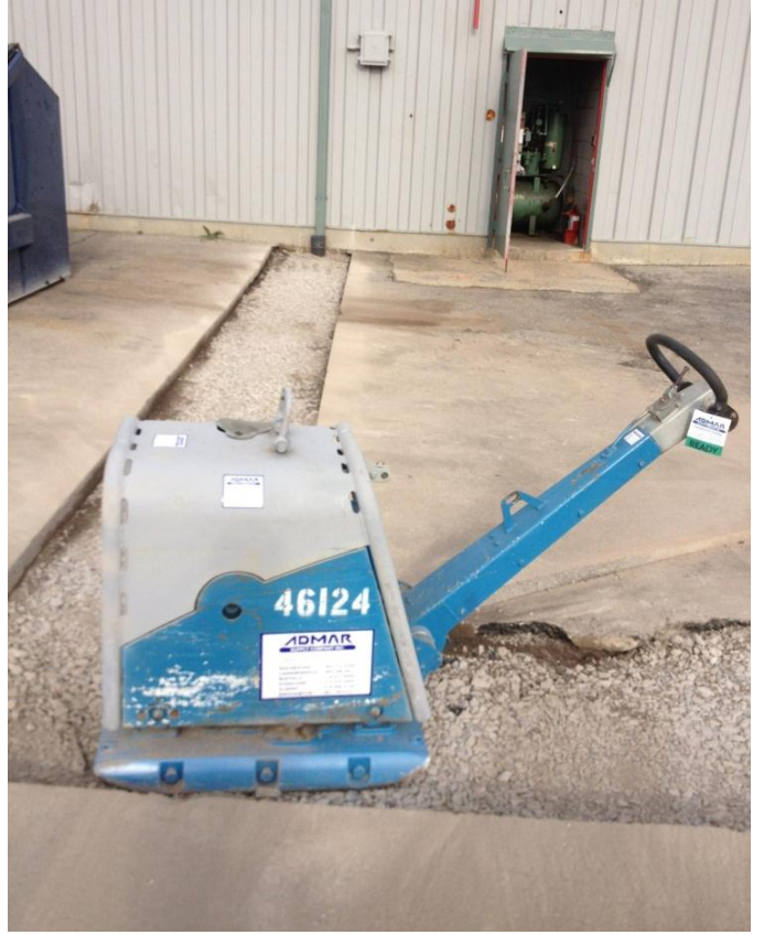
Crusher Run Compaction
