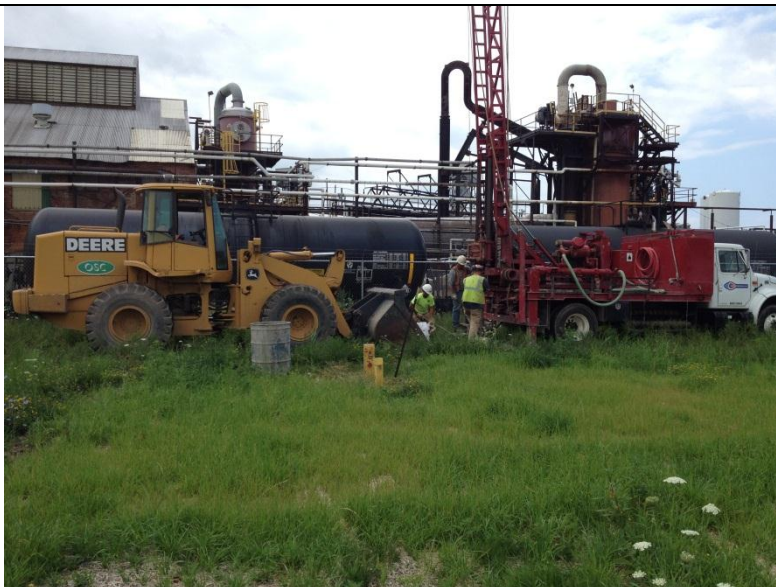
Area E ORC Borehole Installation
