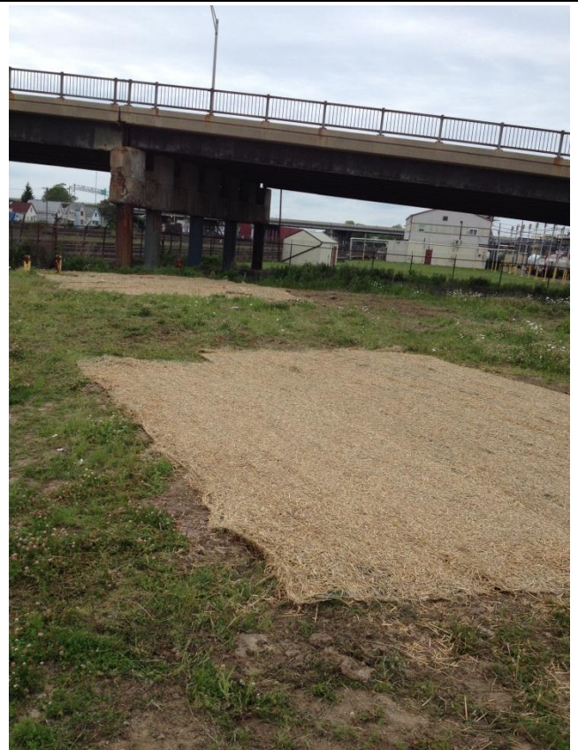
Restoration Near RFI-20
