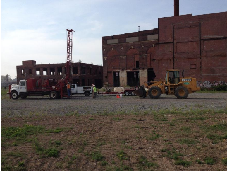
Area C ORC Borehole Installation
