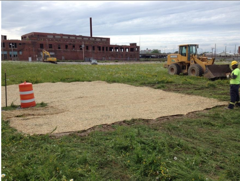
Restoration Near RFI-32
