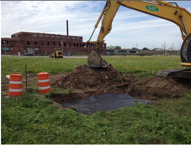
Cover System Fabric Replacement
