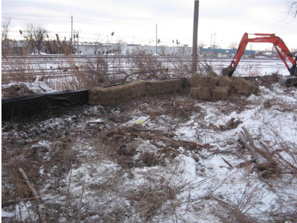
Photograph 5: 2/8/10: Looking southwest, Grid 13 hay bales/silt fence being placed
