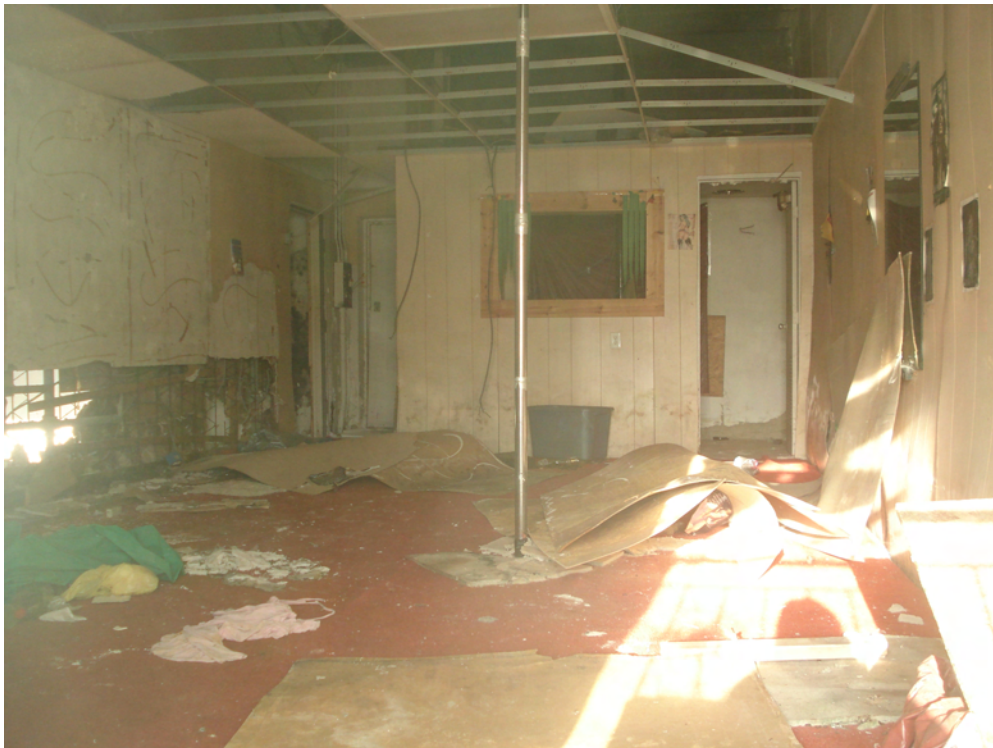
Interior of tenant space in Building 3
