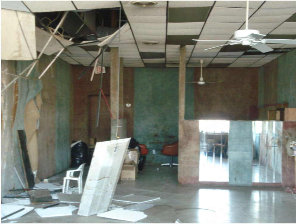
Interior of tenant space in Building 1
