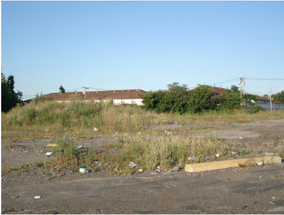
Area of fill stockpile in northeastern corner of Site
