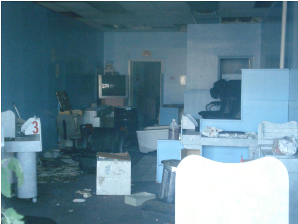
Interior of tenant space in Building 1
