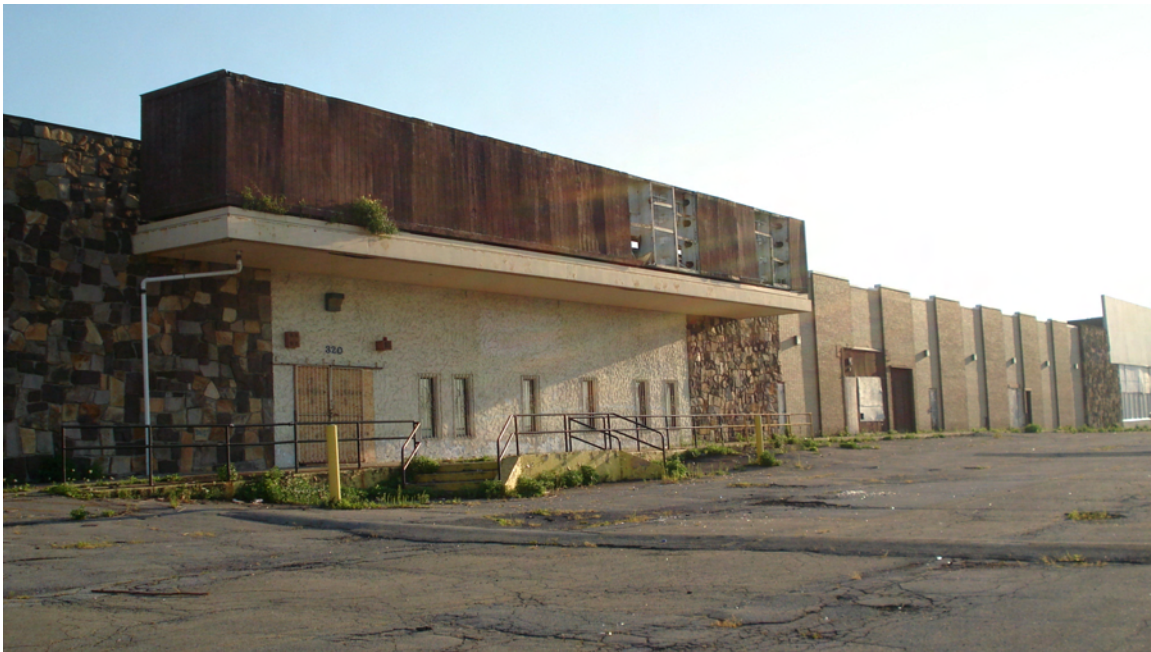
Building 4 looking south
