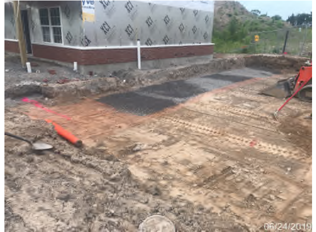
Installation of demarcation layer in green space area looking southeast
