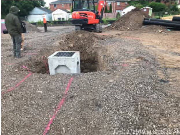
Storm water catch basin looking north
