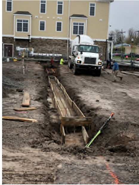
Foundation footer forms looking west
