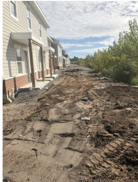
Backfill of gas utility line looking east
