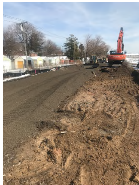
Backfill of storm sewer line looking east
