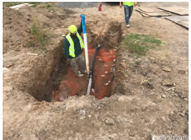
Installation of demarcation layer in gas utility trench looking west
