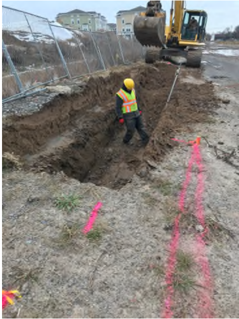
Excavation for building foundation looking west
