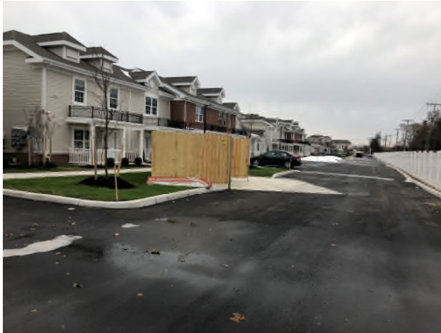
Finishe Townhouses looking west
