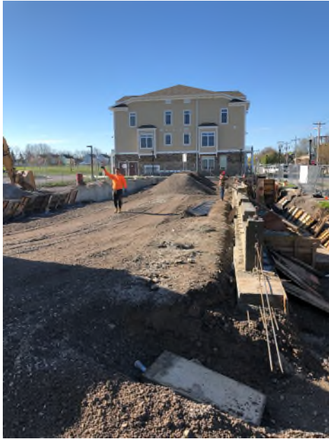
Backfill in building foundation looking west
