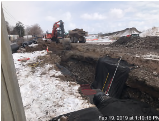
Excavation for storm sewer line looking southeast
