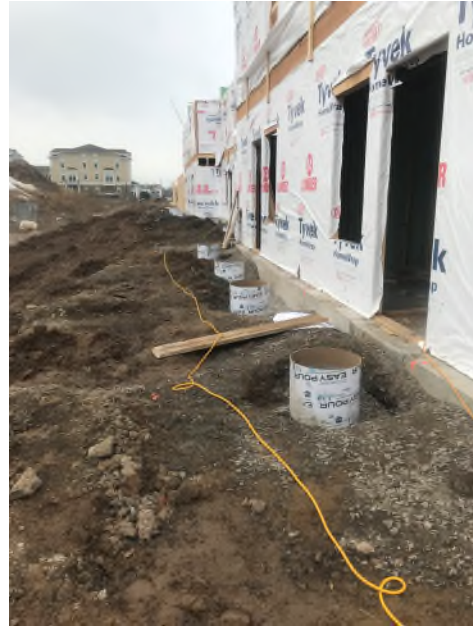
Installation of concrete piers looking west
