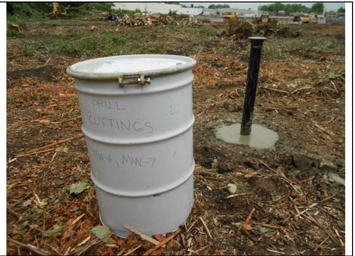
2. View of MW-6 after concrete pad has been poured
