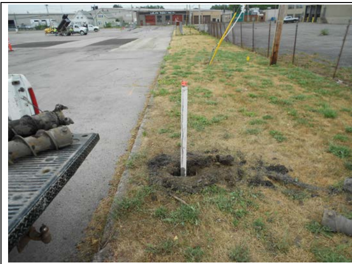
7. View of Monitoring Well MW-3 after riser is installed
