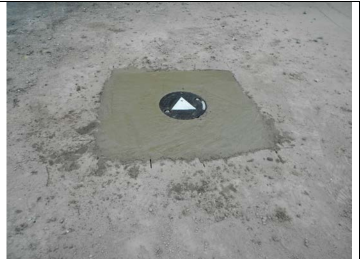
4. After riser is cut, the inner ring is placed and concrete poured
