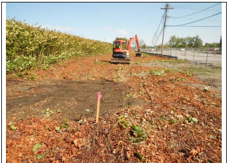
12. TS-14: each test pit is left as level as it was before the dig
