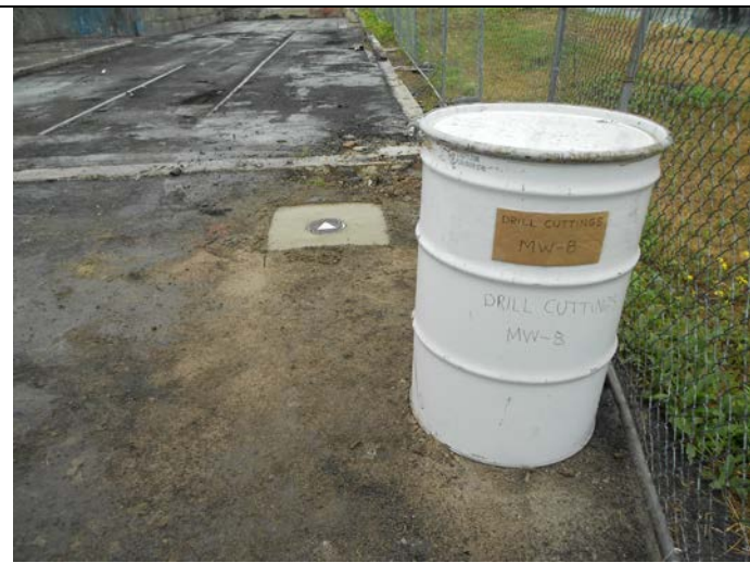
5. View of MW-8 after installation is complete
