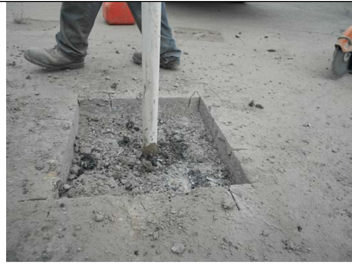
3. The asphalt is removed around MW-5 riser
