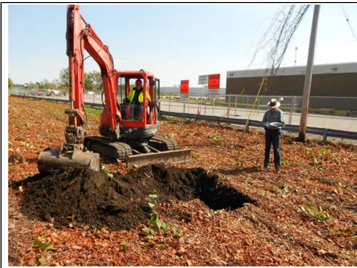
13. Starting to dig Test Pit TS-5
