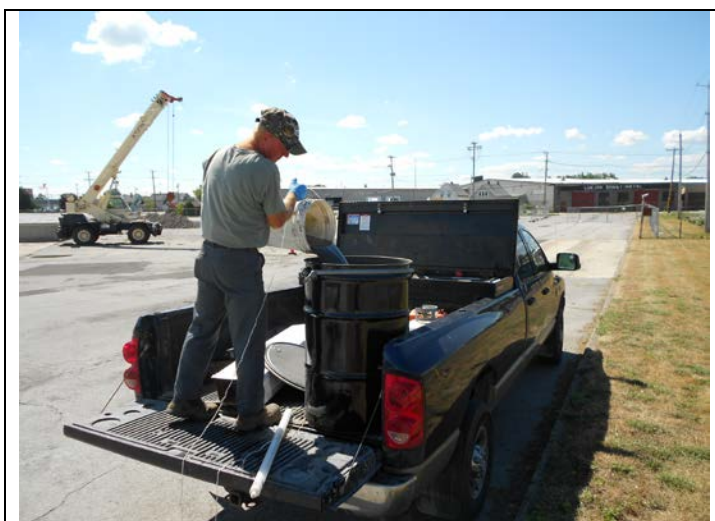
12. The well develop water is then contained
