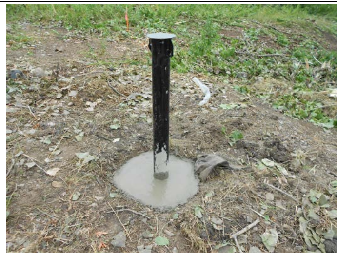
1. View of MW-7 after concrete pad has been poured
