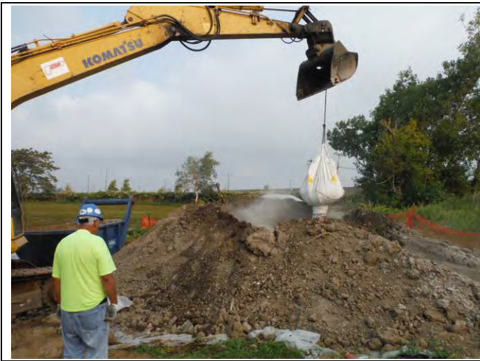
1. View of cement being mixed with excavated soil at TS-9
