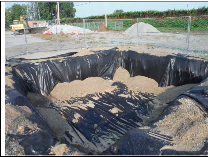
1. View of GS-21 lined with plastic and ready to be filled with approved backfill soil
