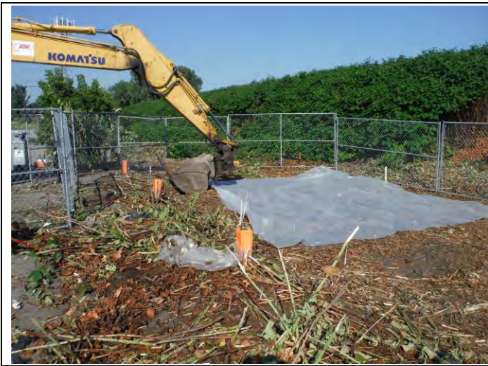
1. Before a hot spot is excavated, plastic is put down for the excavated material
