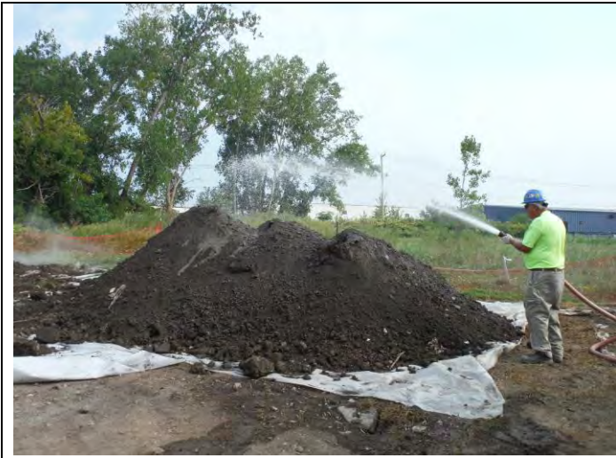
3. Water is added during and after the mixing to achieve the correct moisture content
