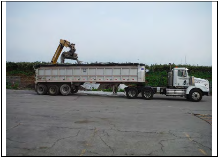
2. View of Tractor Trailer Dump Truck being loaded with excavated material from TS-5
