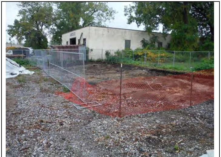
4. View of GS-19 after widening in an attempt to border on cleaner material
