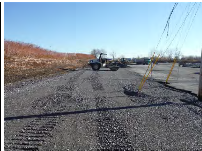
5. After the gravel is graded, it is tamped down with a roller
