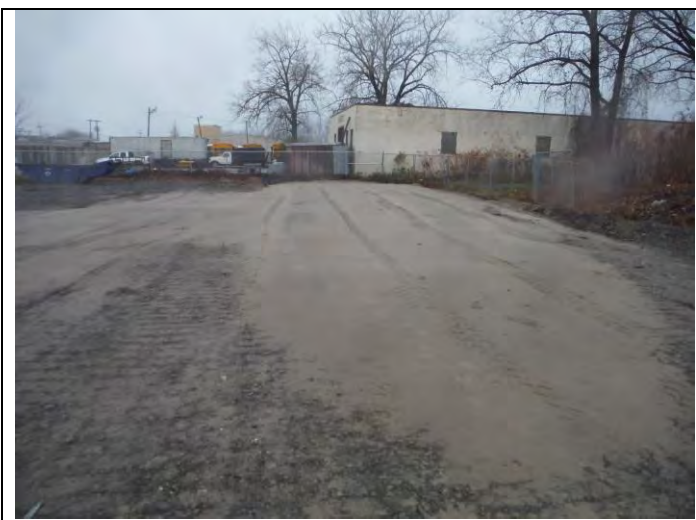
3. GS-19 is approved and gets backfilled
