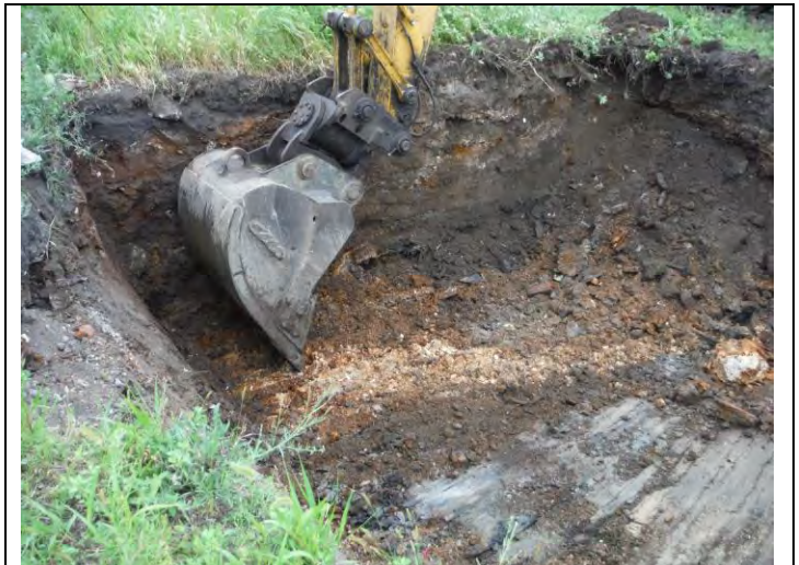
4. View of TS-4 excavation as its west wall is widened another 2' in an attempt to border cleaner material
