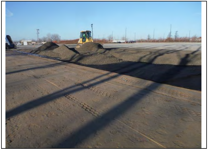
2. Gravel is applied over backfill on the east end
