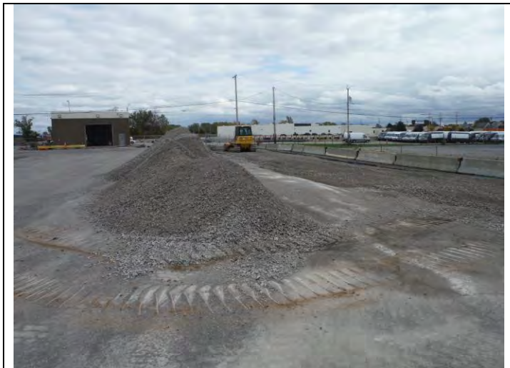
4. Pinto's bulldozer gravels and grades a strip along the south border across from the Cell Tower
