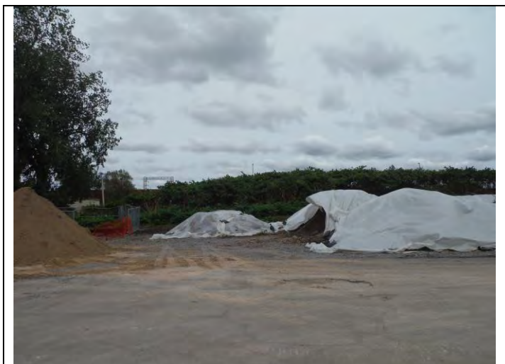
4. View of stockpiled backfill soil and excavated material from GS-19 and Cell Tower material under plastic
