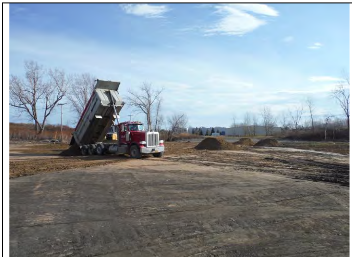
2. Truckloads of clean fill are brought in to raise the grade on the east end of the site
