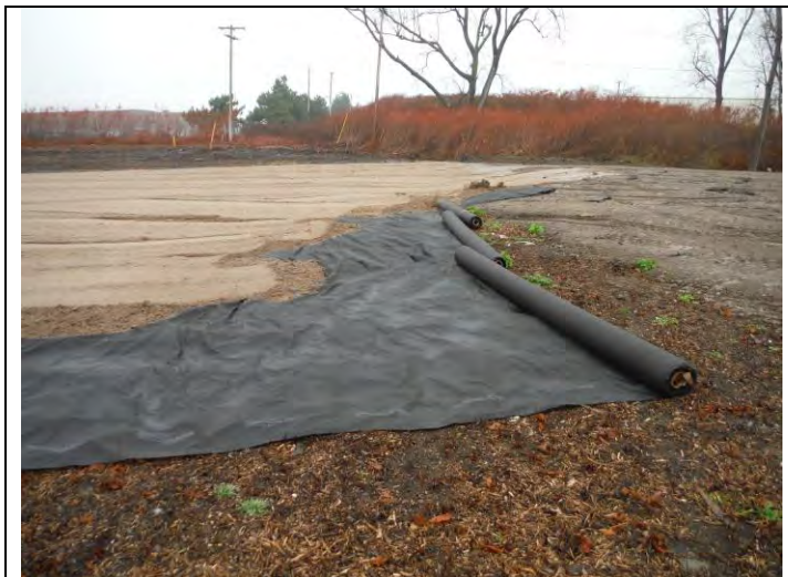
2. View of geotextile and backfill being applied to northeast section of site
