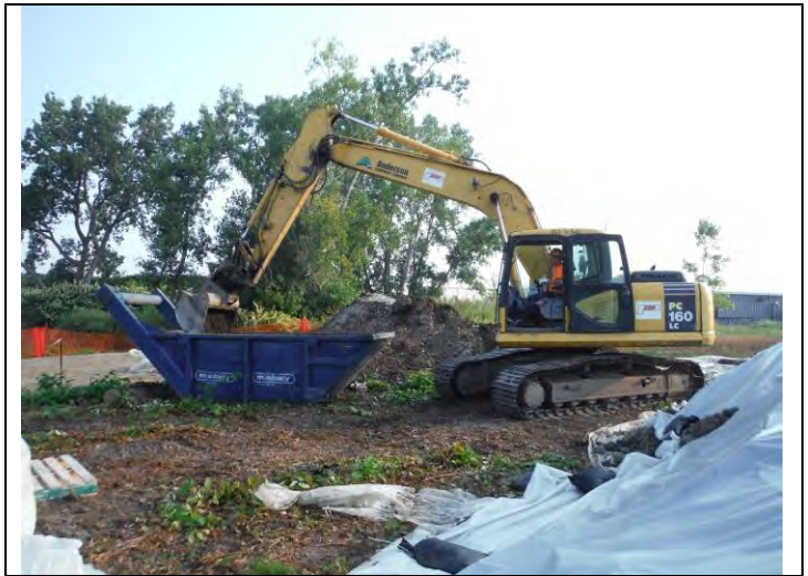
2. After the cement is added to the pile, it is mixed inside the stone vat
