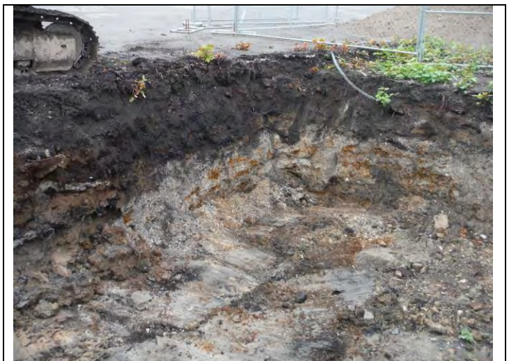
6. View of TS-13 after widening in an attempt to border on cleaner material
