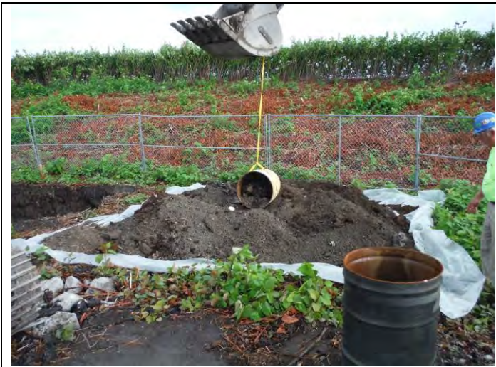
3. The stored drill cuttings in the 55 gal drums were dumped onto the MW-2 excavation pile
