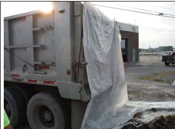
5. Approved excavation piles are loaded into dump trucks for disposal. The plastic sheet keeps the outside of the truck clean.
