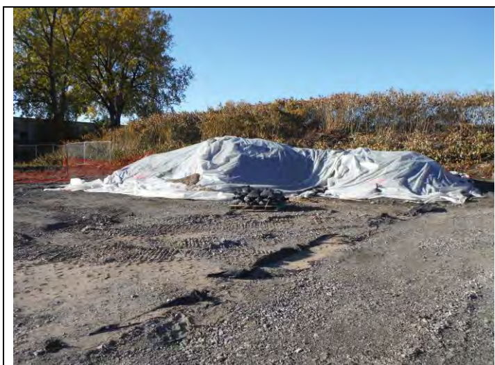
6. . View of TS-15 excavation pile while waiting for disposal approval
