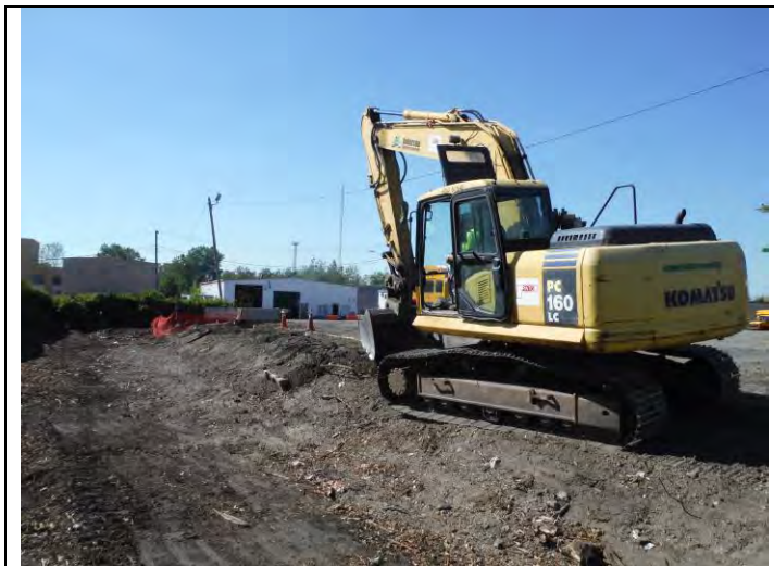
2. View of Pinto's excavator digging test pits at GS-17
