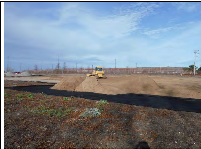
3. The bulldozer spreads backfill over the geotextile fabric
