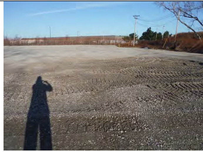
3. The entire northeast section has been graveled and graded
