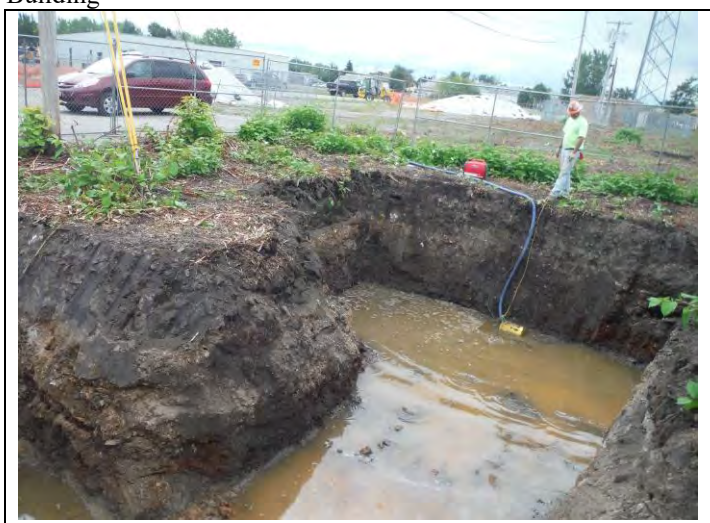
5. View of Pinto crew pumping ground water out of TS-5
