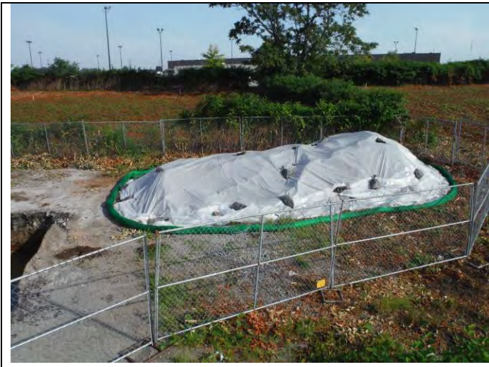
3. All excavated piles are covered with plastic before the end of each day
