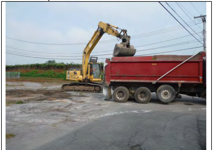
6. View of GS-21 excavated pile being loaded into a tandem dump truck for disposal
