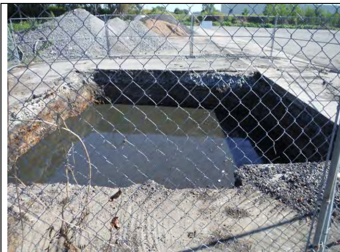
5. GS-30 after being widened and deepened to border with cleaner material
