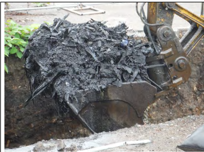
5. View of excavated trash at the bottom of MW-2 as it is deepened again in an attempt to reach cleaner material
