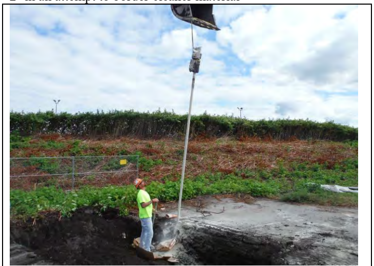
6. View of MW-2 Piezometer Well being decommissioned at MW-2
