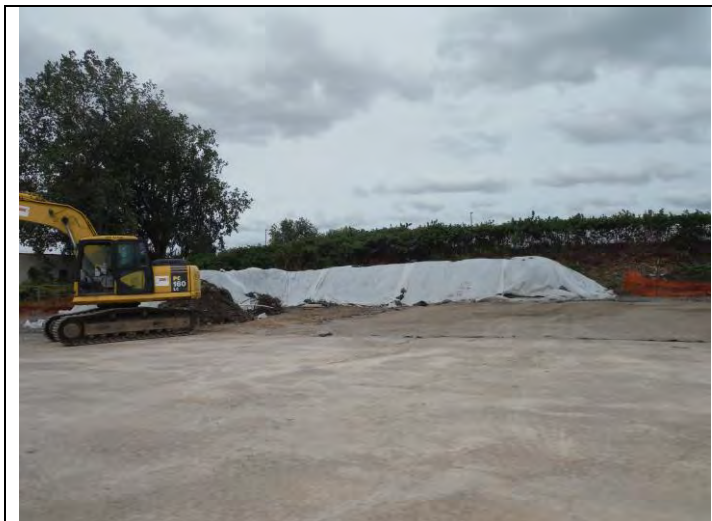
2. View of covered Cell Tower Expansion excavated material
