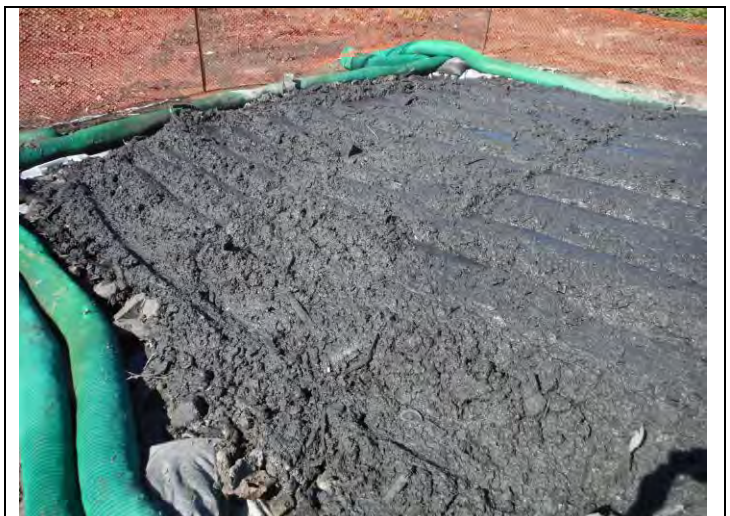
6. View of excavated material from GS-30 drying out on plastic
