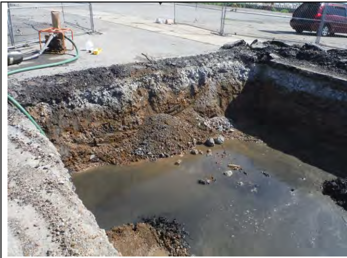
5. View of GS-30 as groundwater is pumped out
