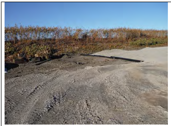
4. Geotextile fabric is put down before the gravel is applied
