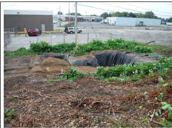
5. View of TS-5 lined with plastic and being backfilled with approved soil
