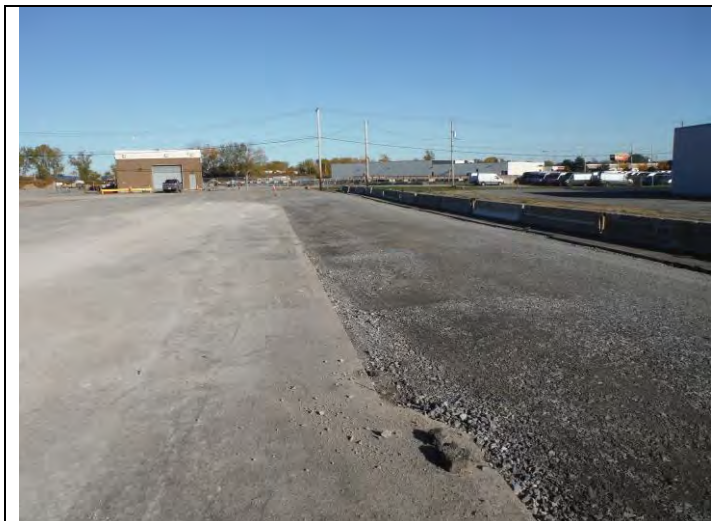
2. View of south section of site after graveling and grading
