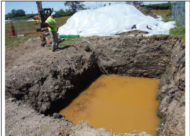
4. View of TS-9 as groundwater is pumped out
