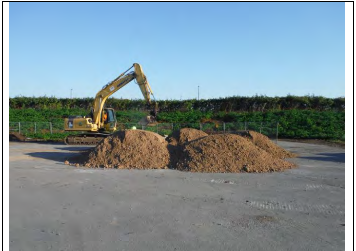
4. Approved backfill material is staged on asphalt
