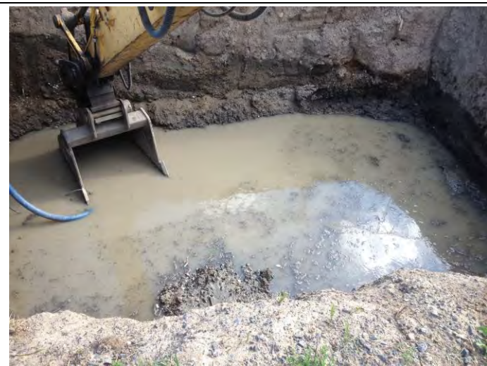
1. Pumping ground water out of TS-9
