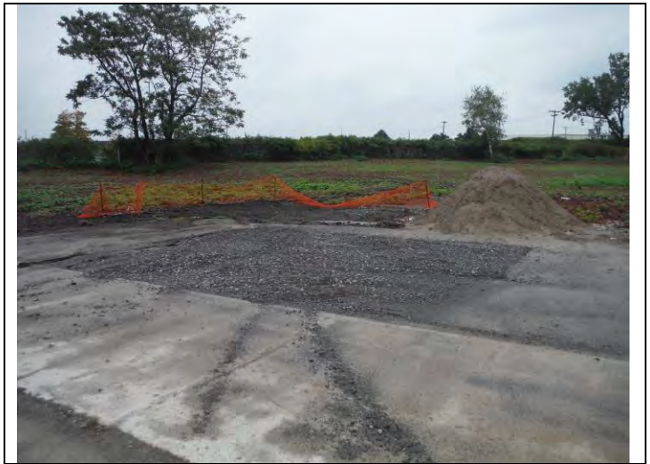
2. View of GS-30 after it has been backfilled and graded
