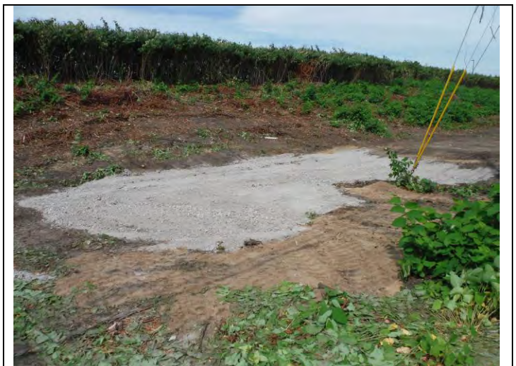
6. View of TS-5 after it is graded off with gravel
