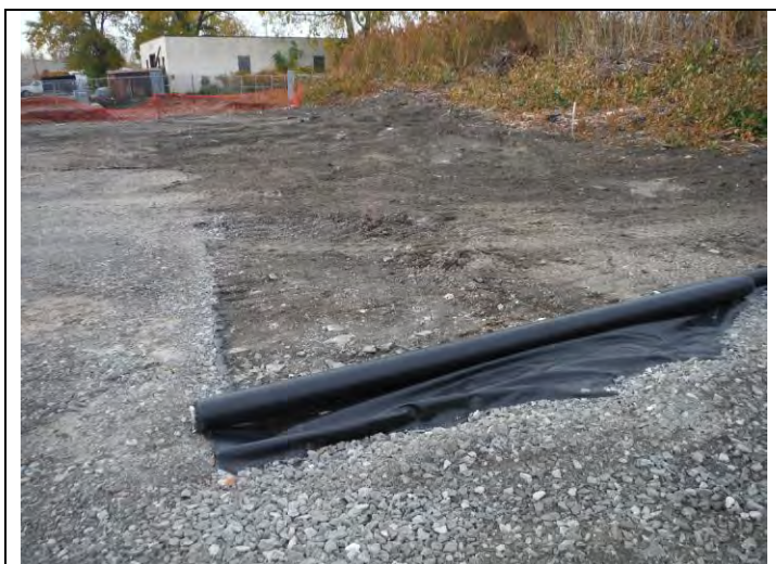
6. Close view of gravel application with the geotextile underlay on the north side of the site
