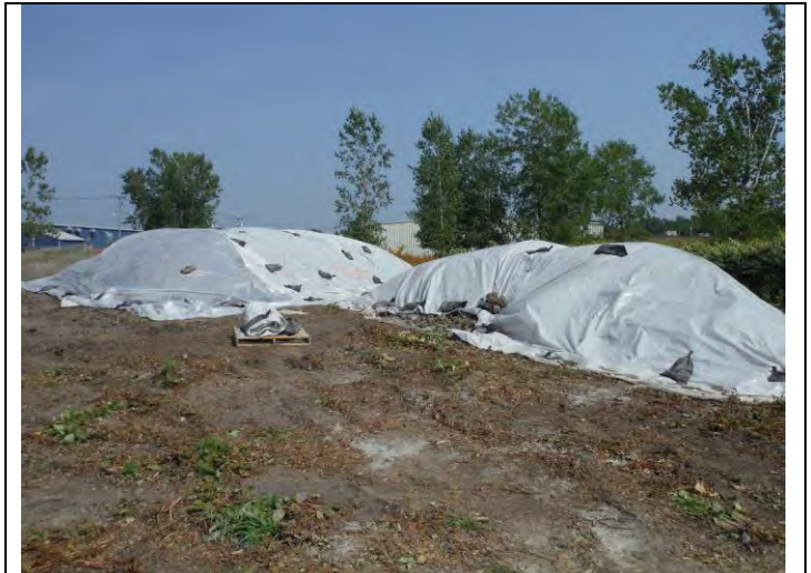
4. Before the end of the day, all mixed excavation piles are covered with plastic
