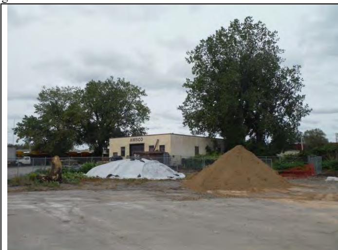
3. View of stockpiled backfill soil and excavated material from GS-19 under plastic
