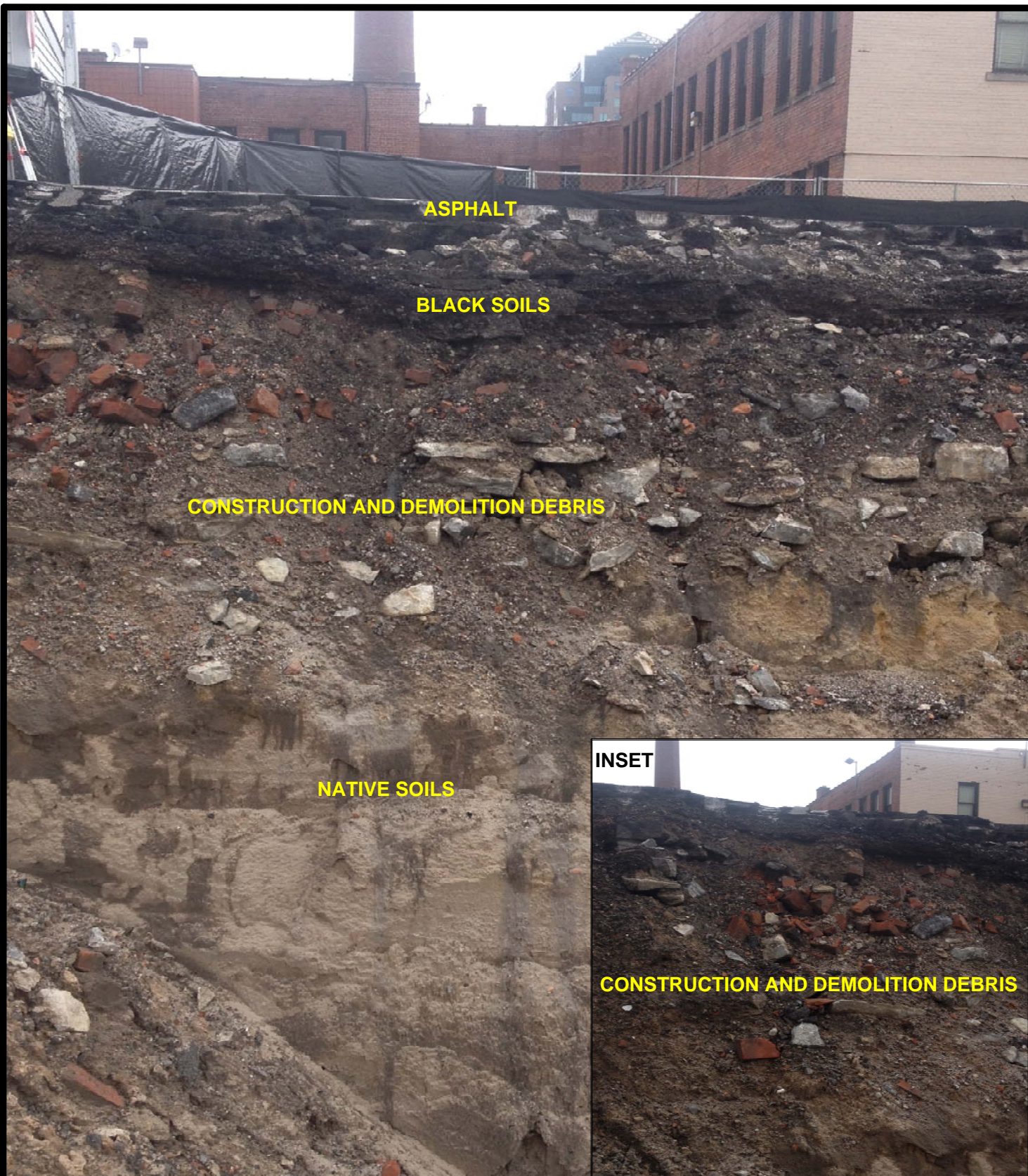
FIGURE 7 HISTORIC FILL MATERIALS EXPOSED ON THE EAST WALL OF THE PETROLEUM-RELATED SOIL EXCAVATION
