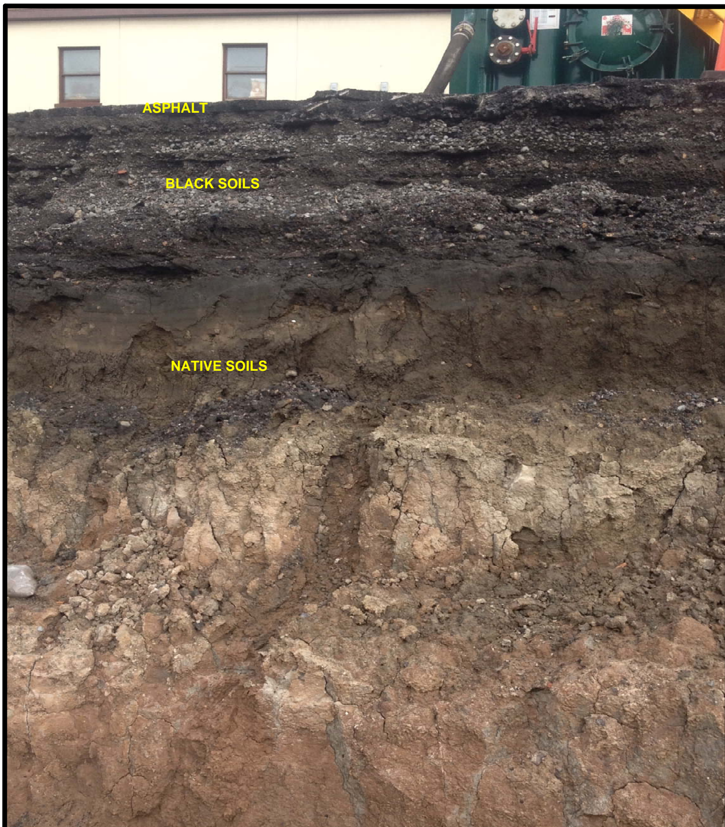
FIGURE 6 HISTORIC FILL MATERIALS EXPOSED ON THE NORTH WALL OF THE PETROLEUM-RELATED SOIL EXCAVATION
