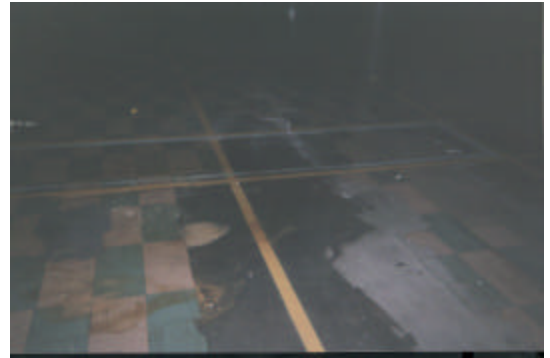
Suspect asbestos containing floor tile on vacant floor
