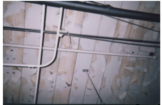
Peeling suspect lead based paint
