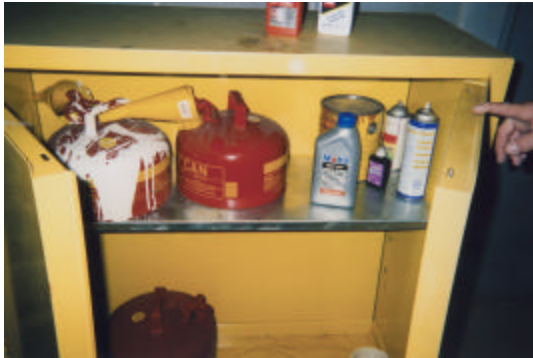
Flammable storage cabinet in boiler room
