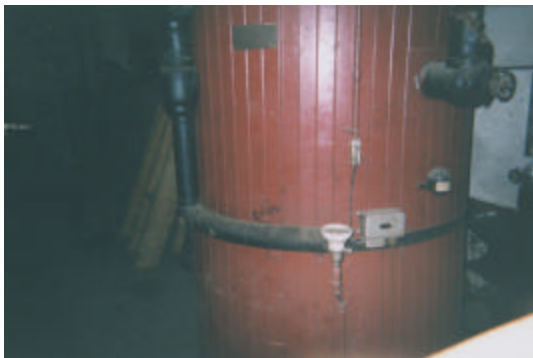
Water storage tank for sprinkler system
