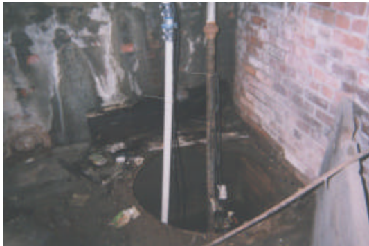
Sump in partial basement area
