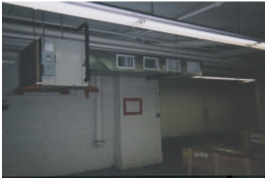
Typical ceiling mounted furnace
