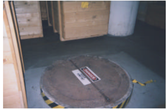
Access area for underground water storage tank for sprinkler system
