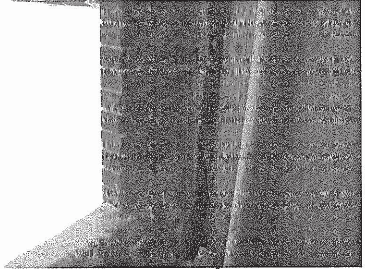
ACM Tar Counterflashing at Interior Support Piers
