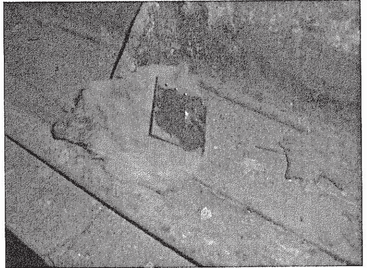
ACM Glue Debris Scattered Throughout Boiler Room
