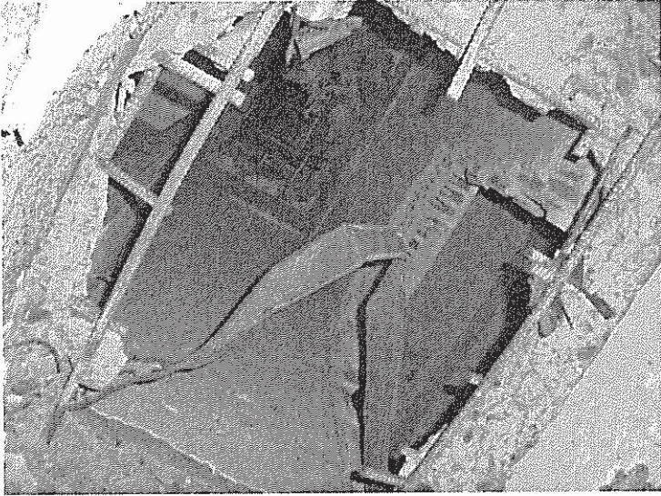
Chute Made by Contractor with ACM Counterflashing Paper Hanging From Rebar
