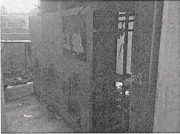
Switchgear Box in the Transformer Room with Bake-Lite Panels in it
