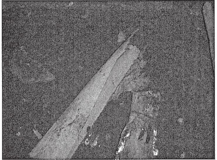
Crawlspace Soil Contaminated with ACM Pipe Insulation
