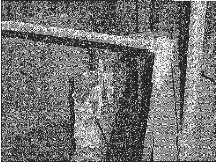
ACM Pipe Insulation Still in Place on Pipes Behind Boiler
