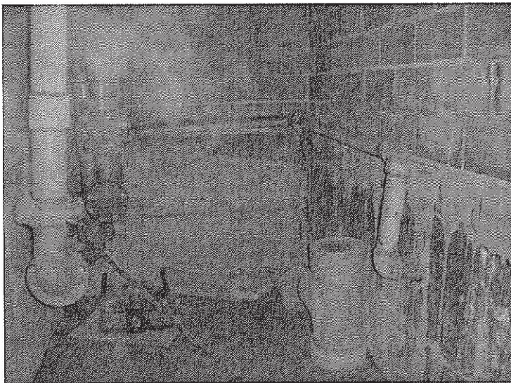
ACM Flange Gaskets in Gas Meter Room
