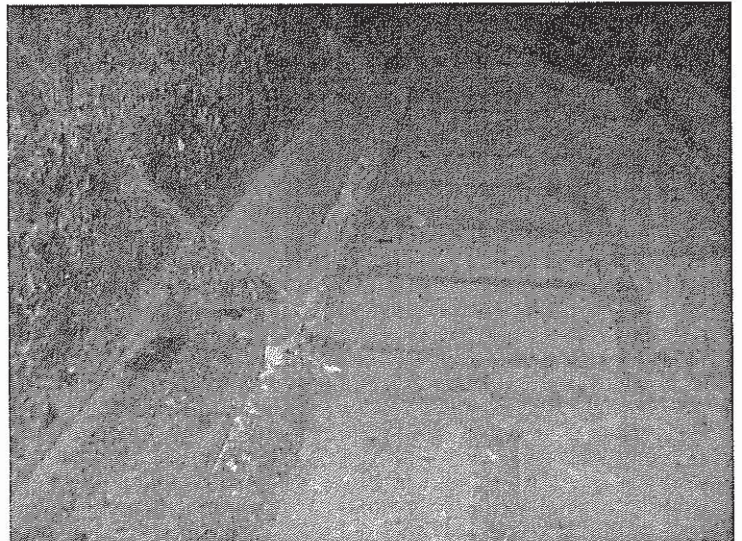
ACM Boiler Insulation at Seam of Boiler
