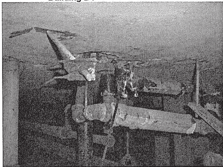
Some ACM Pipe Fitting Still in Place in Crawlspace.
