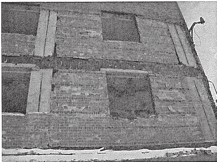
ACM Counterflashing Tar Still in Place on Support Piers
