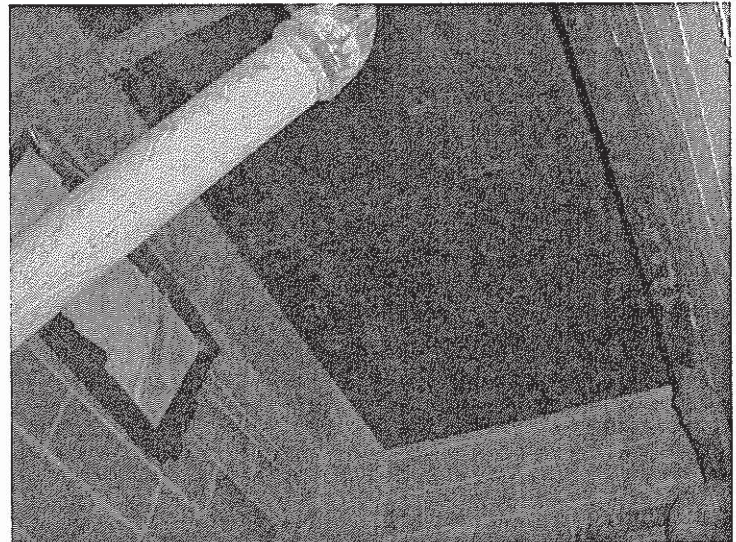
Ceiling Insulation in Place in Gas Meter Room with ACM Glue Holding the Pins to the Ceiling.
