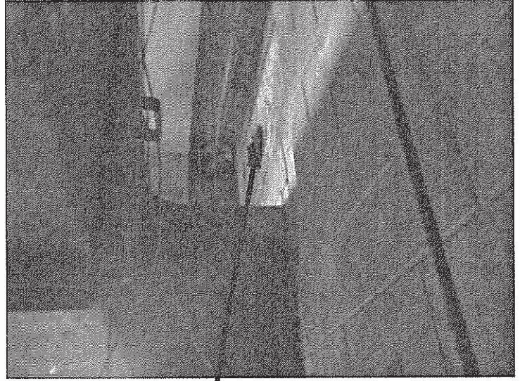
ACM Transite Pipe Still in Wall
