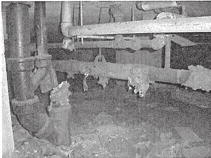
Some ACM Pipe Fitting Still in Place in Crawlspace. Soil Contaminated with ACM Debris
