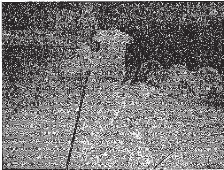
Crawlspace Soil Contaminated with ACM Floor Tile Debris. ACM Flange Gaskets Still in Crawlspace
