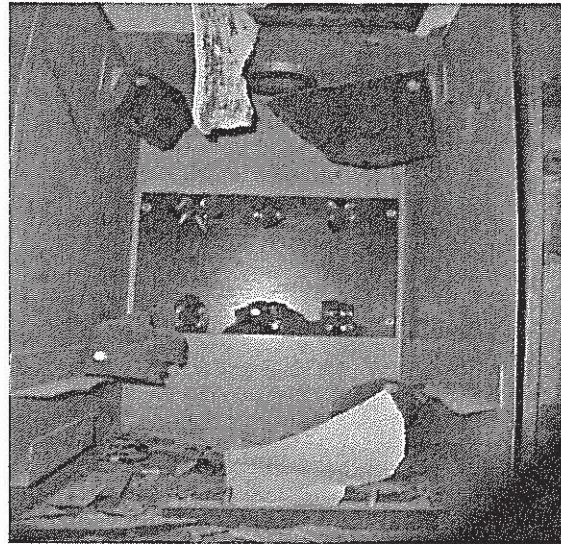
Transformer Room Cabinet with ACM Transite, Bake-Lite and Electrical Paper Debris.
