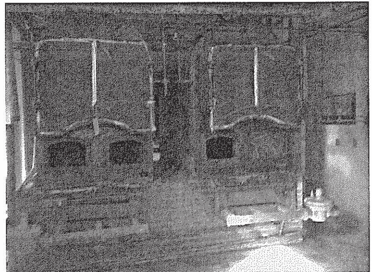
Boiler with Suspect ACM Located Inside, ACM Boiler Insulation at Seam of Boiler and ACM Boiler Gasket on the Doors
