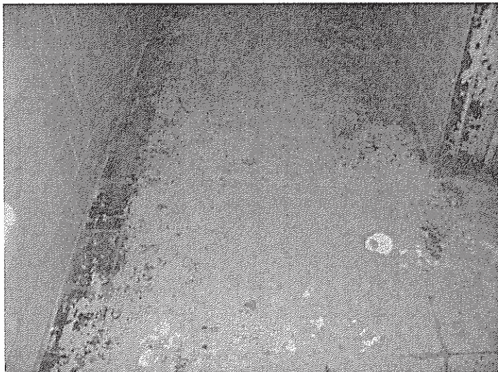
ACM Floor Tile Debris and Mastic Inside Building
