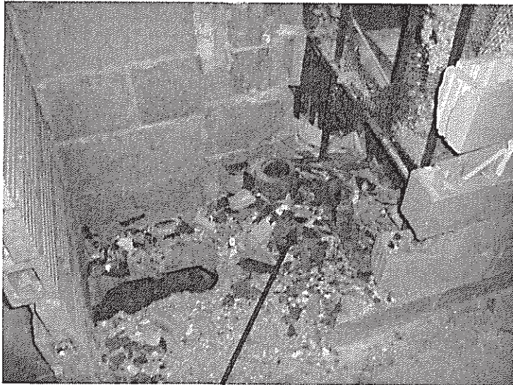
ACM Floor Tile Debris Around Hole to Crawlspace
