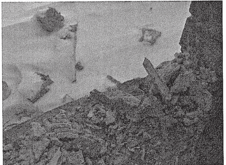
ACM Window Caulk Debris Inside Window Openings.
