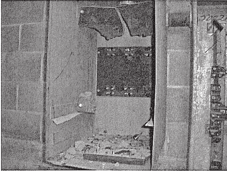
ACM Transite and Bake-Lite Debris in Cabinet in Transformer Room
