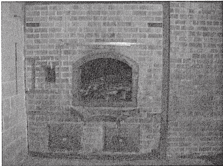
Incinerator with Suspect ACM Located Inside
