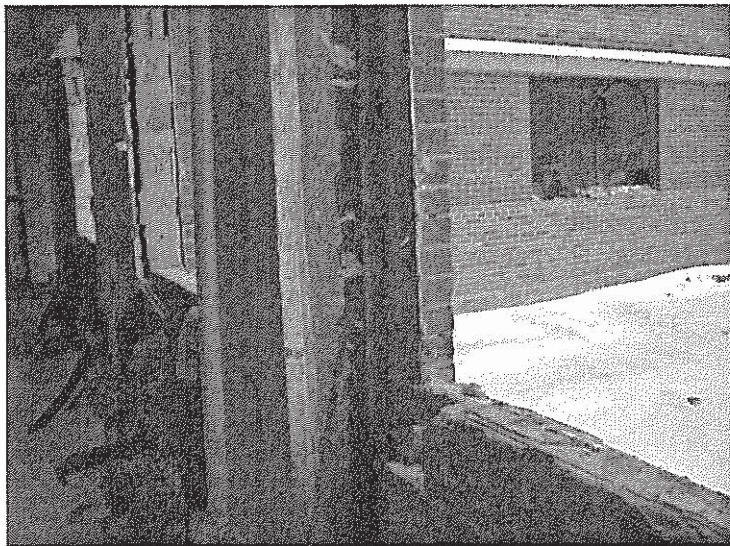
ACM Tar Counterflashing at Interior Support Piers and ACM Window Caulk Still in Place
