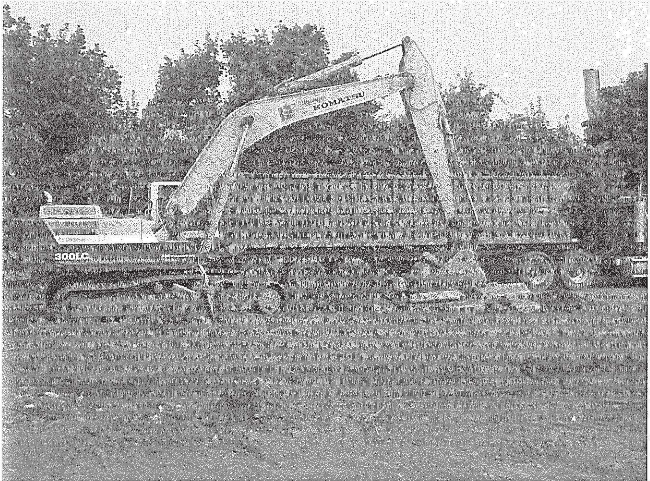
Curb removal North of Building A-1
