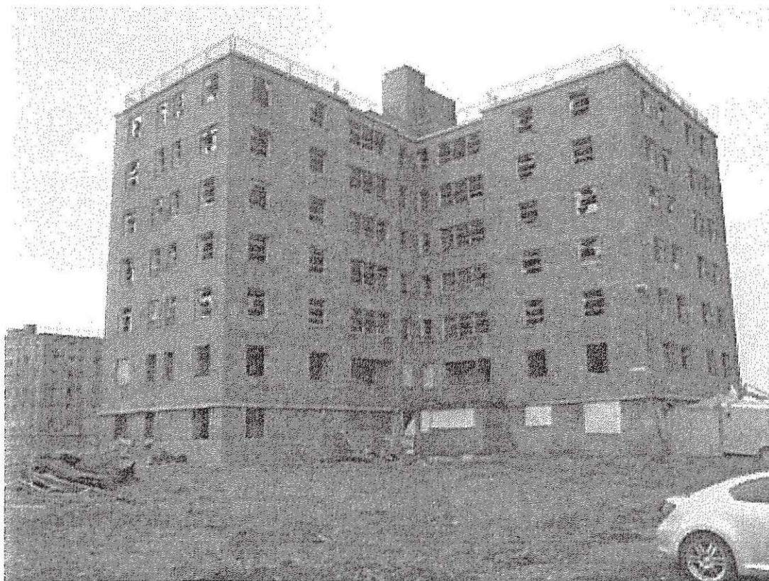
Building B-2, abatement progressing - 1 st & 2 nd floor window frames removed
