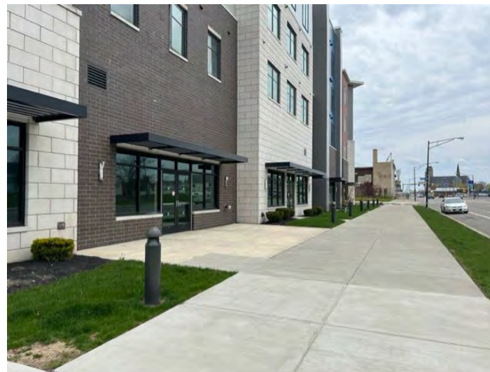
22. South of 490 Broadway looking east
