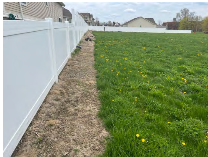
30. View from northwest corner of 233 Mortimer, looking northeast
