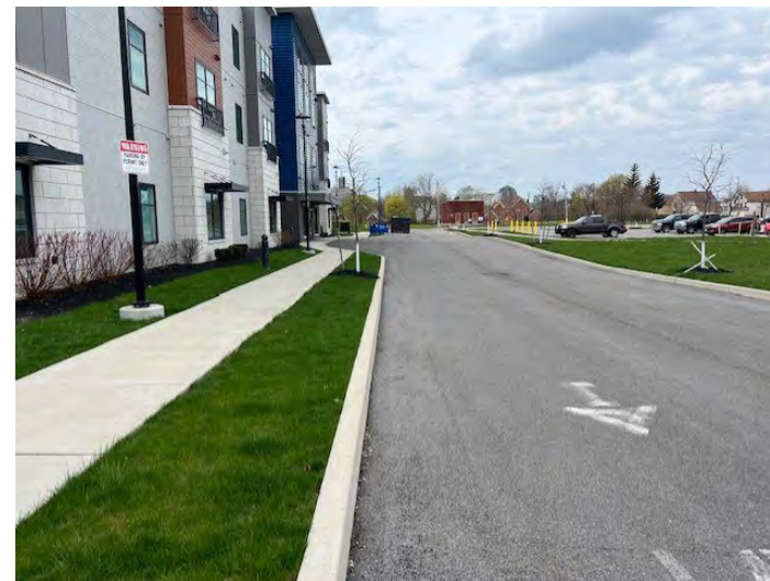
16. Roadway north of building on 490 Broadway looking west
