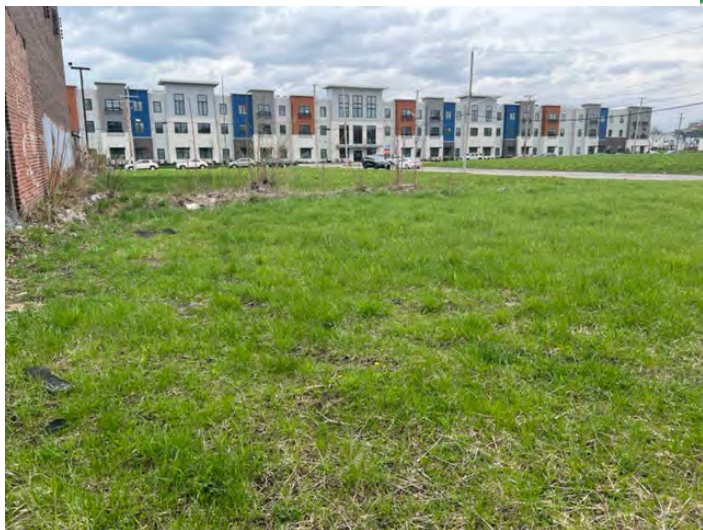
39. View of 498 Broadway looking south
