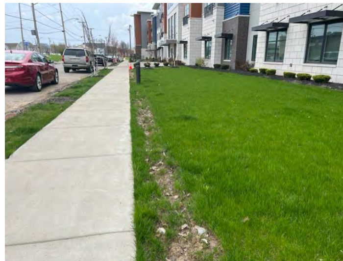
18. View of 490 Broadway continuing south along the building
