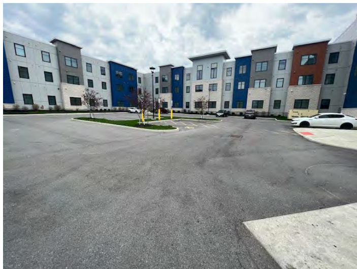
23. View of south parking area of 490 Broadway, looking northeast
