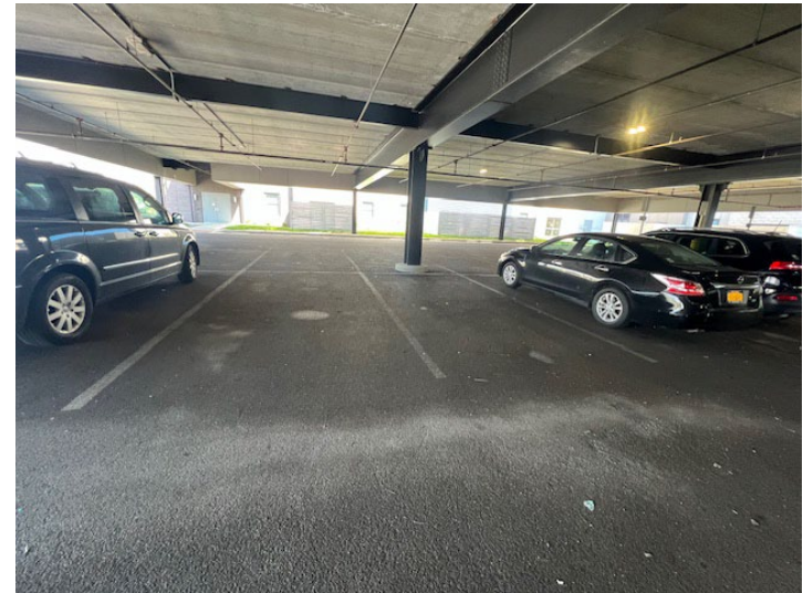
12. Parking area beneath northwestern portion of building, facing east.
