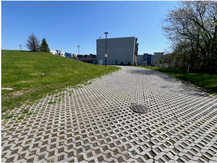
13. Western entrance along Spring Street, facing east.
