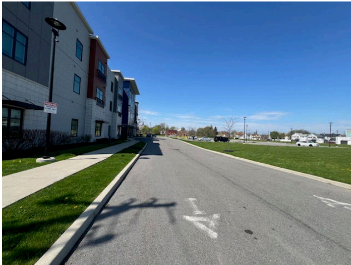
7. Access road traversing the northern entrance, facing west.
