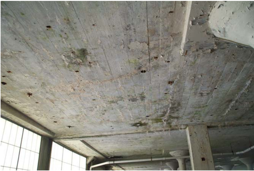
Underside of deck in Bldg. 3, note efflorescence, stalactites, multiple cracks
