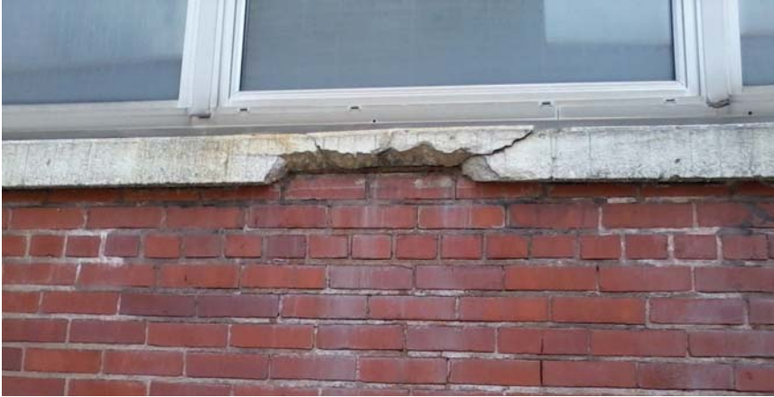
Typical spalling/broken window sill
