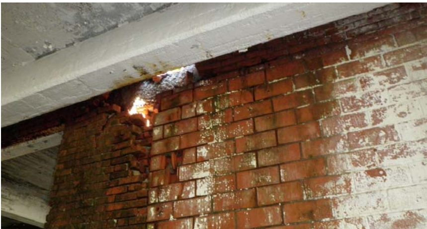
Roof penetrated as a result of collapsed masonry parapet in photo above, note ongoing deterioration of masonry wall
