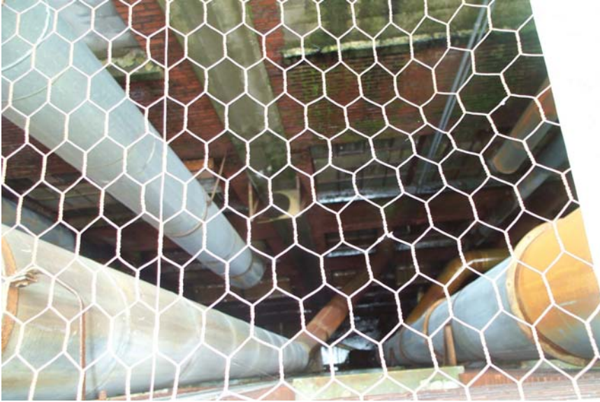
Looking down a light Well in Bldg. 8, masonry is wet and deteriorating due to continuous presence of water
