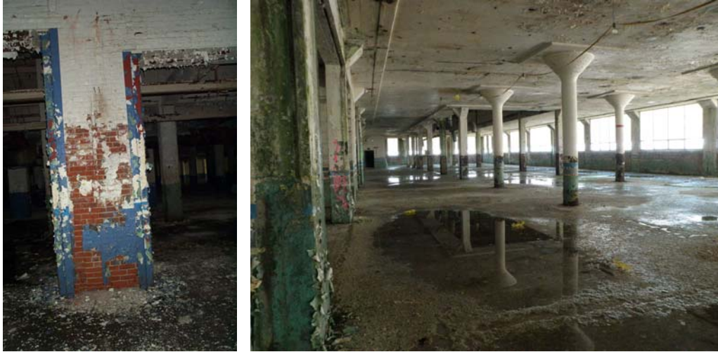
Various paint colors and types that are chipping throughout the building.
