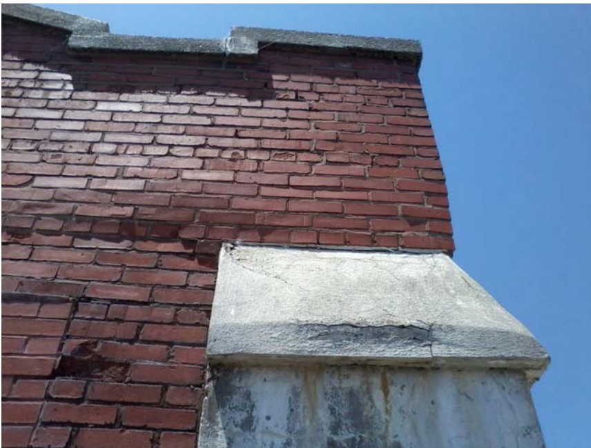
Warped masonry at top of column illustrated in Previous Photo
