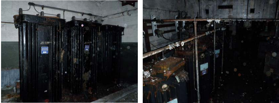
Remaining transformers and oil storage located in the basement.
