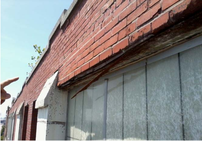
Typical failing lintel over window
