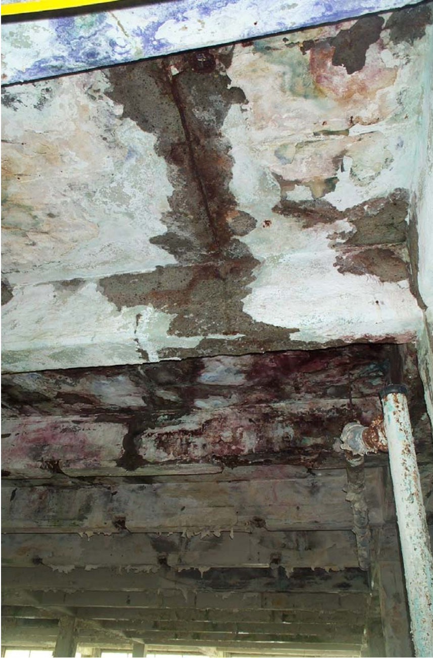
Underside of floor deck, note heavy scaling and exposed reinforcement, localized condition
