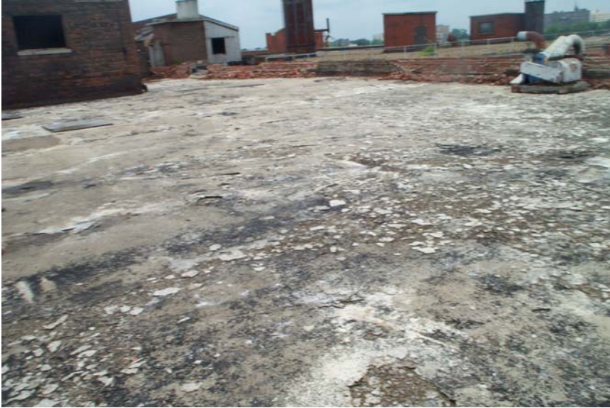
Typical condition of roof in areas where membrane has been removed, heavy freeze/thaw scaling and spalling
