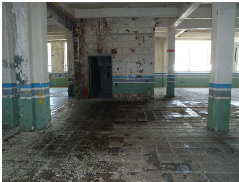
Second floor sheet flooring material which is potentially asbestos containing.
