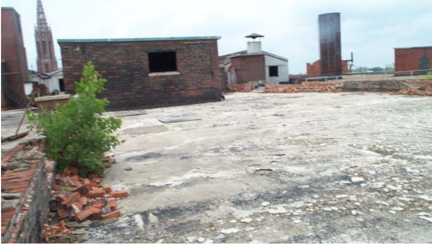
Condition of masonry at roof level
