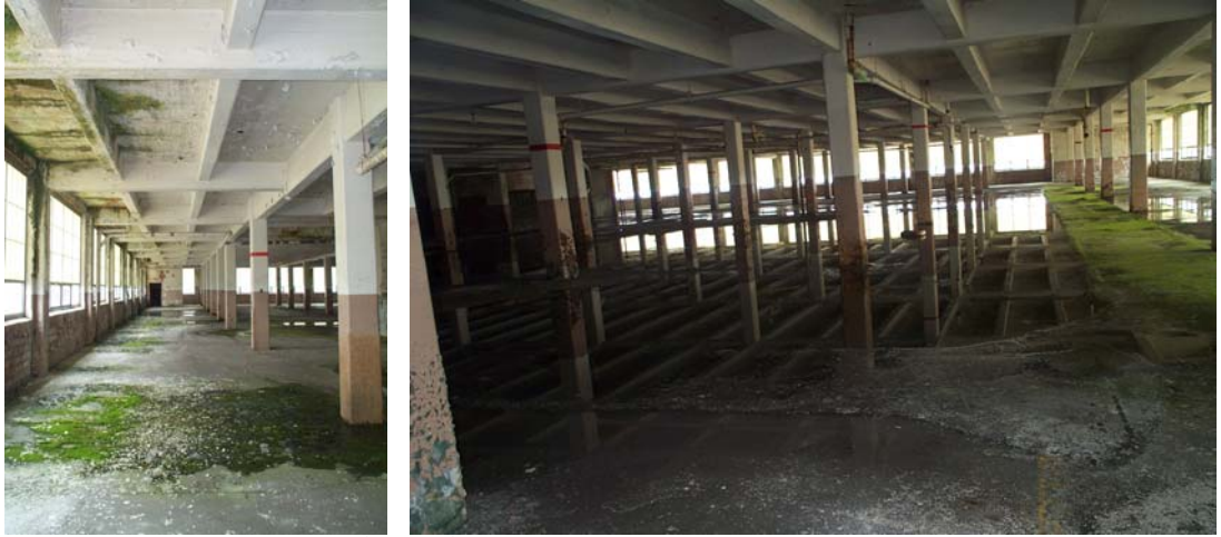
Mold and moss growth on the 6 th and 4 th floors respectively.
