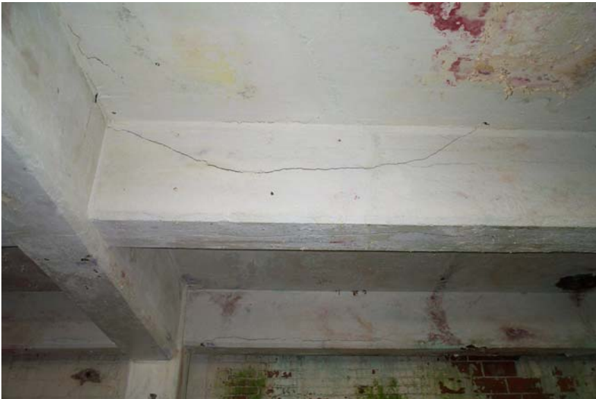
Cracked beam encasement in Bldg. 8, second floor, localized condition
