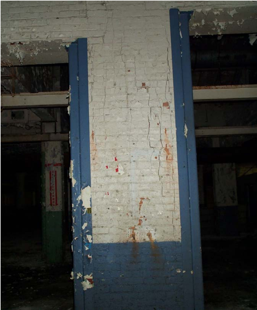
Failing column section in lower level of Bldg. 1, note multiple vertical cracks in column face
