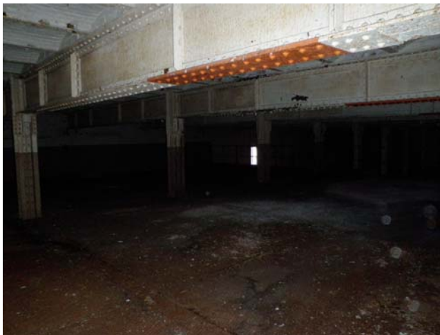
The former chemical storage room (Building 1) with heavy red staining on the floor.
