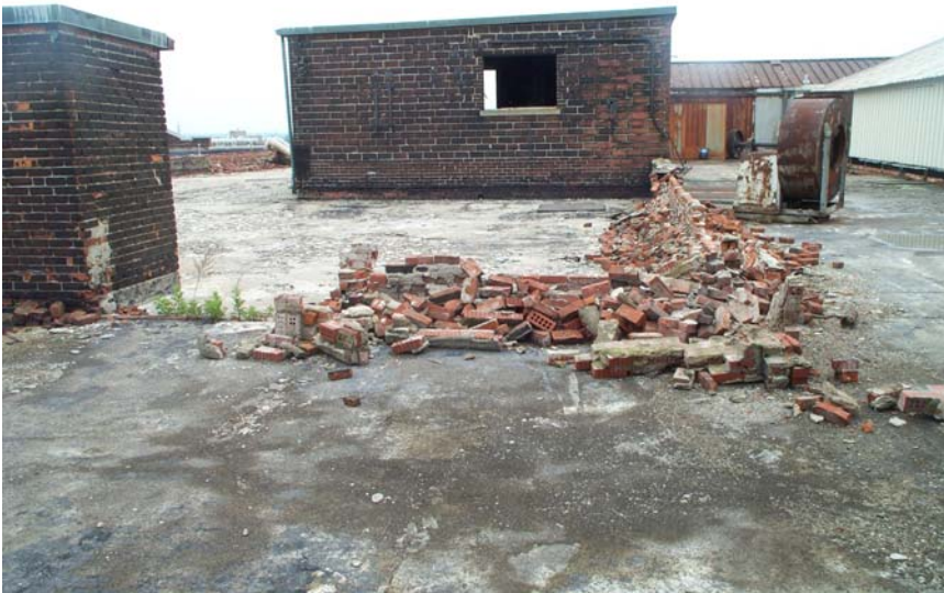
Collapsed parapet at SW corner of Bldg. 1
