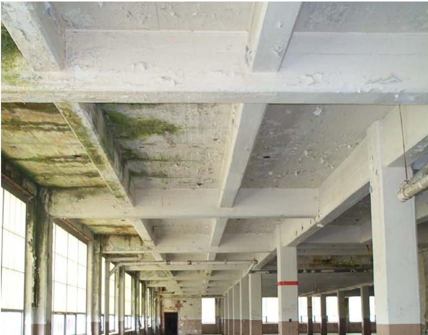
Underside of floor deck, Bldg. 8, note variation of condition from building face inward
