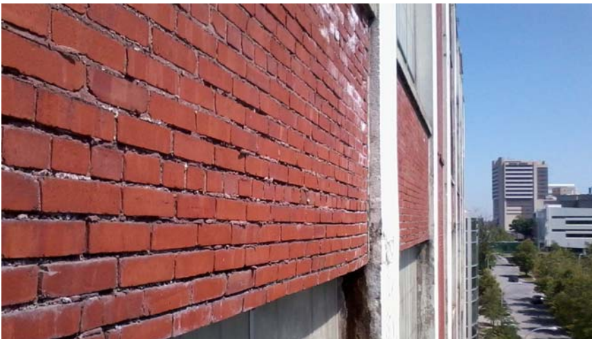
Typical condition of masonry on upper areas of building facade
