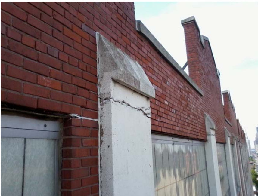
Typical crack in column encasement concrete on building facade
