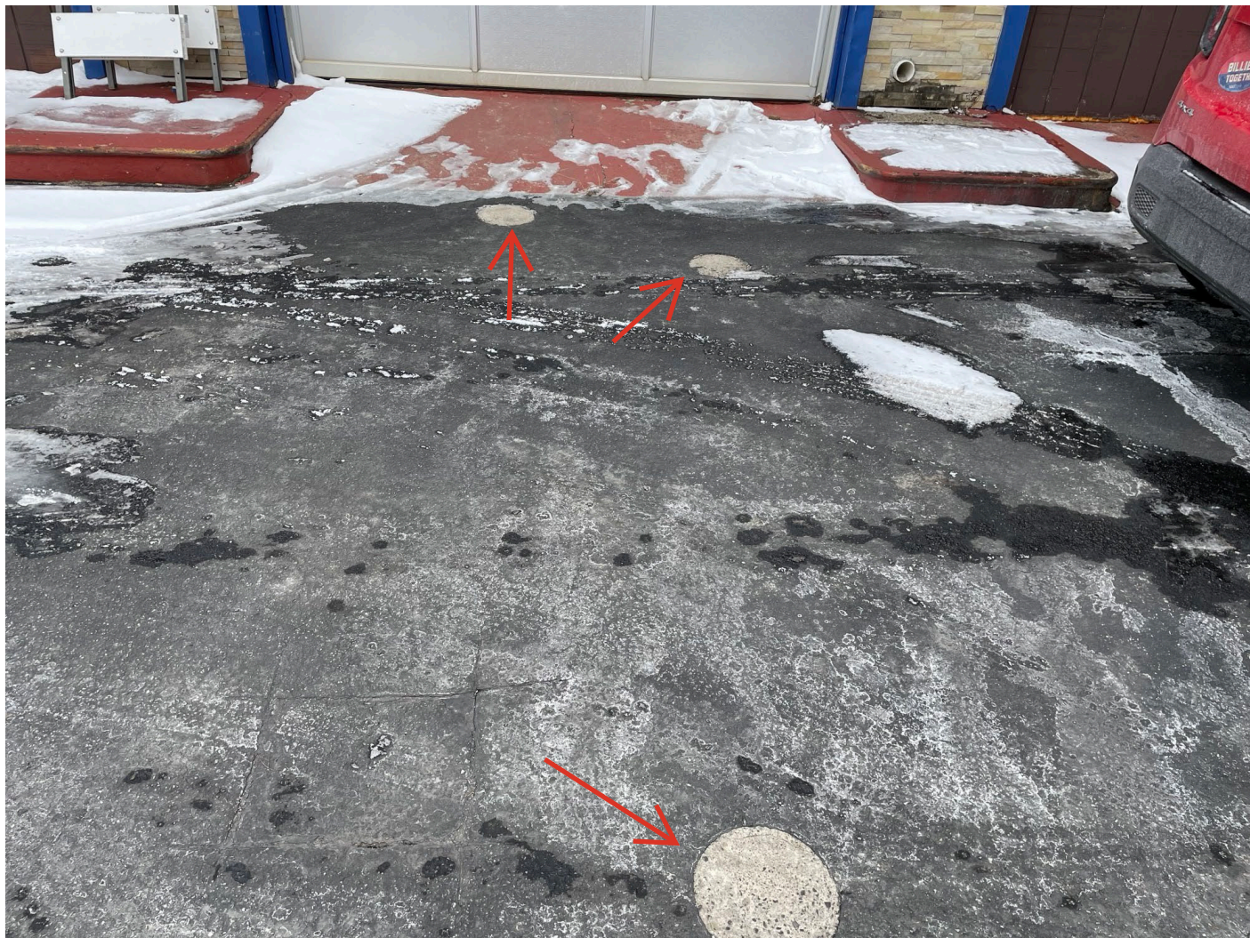
Former Sunoco spill site conditions/probable decommissioned monitoring wells.
