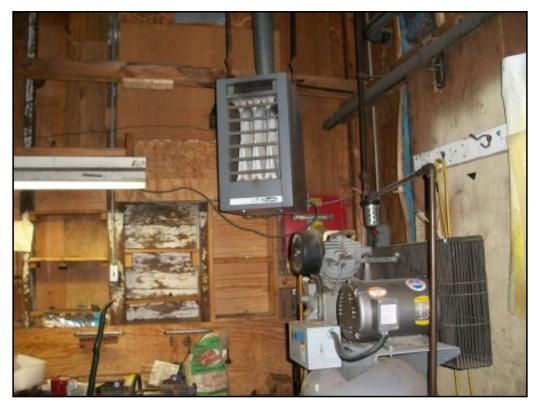
View of natural-gas fired ceiling mounted heating unit in historic maintenance shop.
