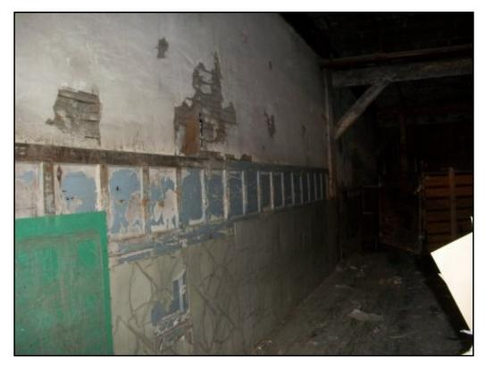
View of damaged suspect ACM plaster.
