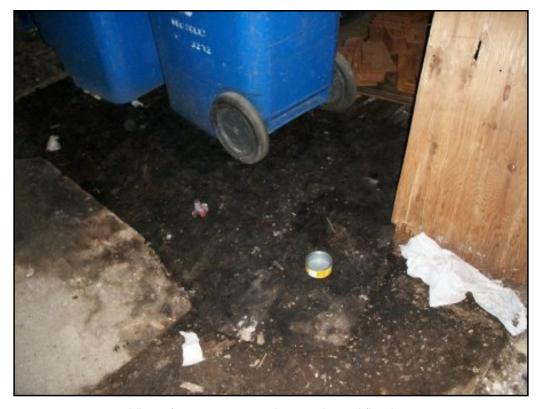
View of apparent water damaged wood flooring.
