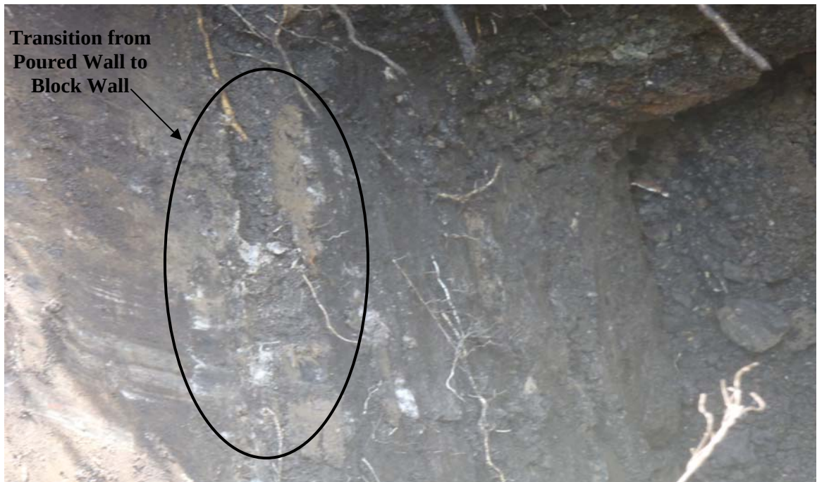
Photograph 8 –Test Pit TP-4 – Formed and Poured Foundation Wall Placed over Previous Stone Block
