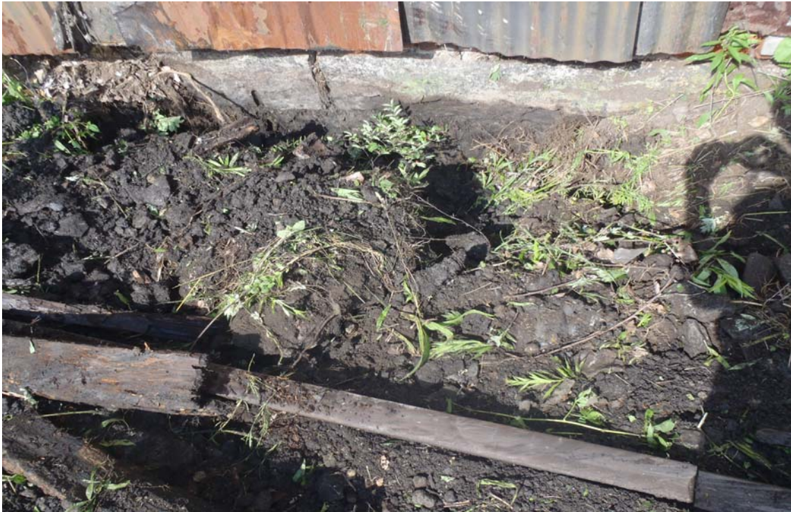
Photograph 3 –Test Pit TP-2 – Surface Fill Soils – Top Portion of Stone Block Foundation Wall
