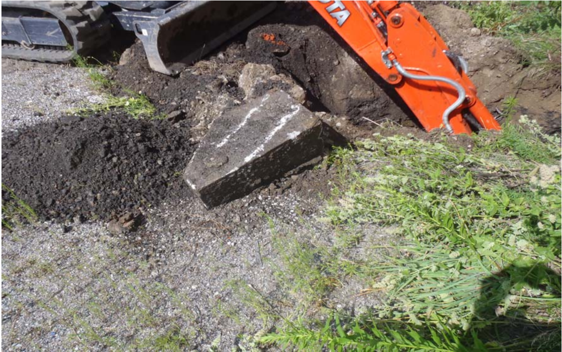
Photograph 9 –Test Pit TP-4 – Stone Block Removed from Test Pit
