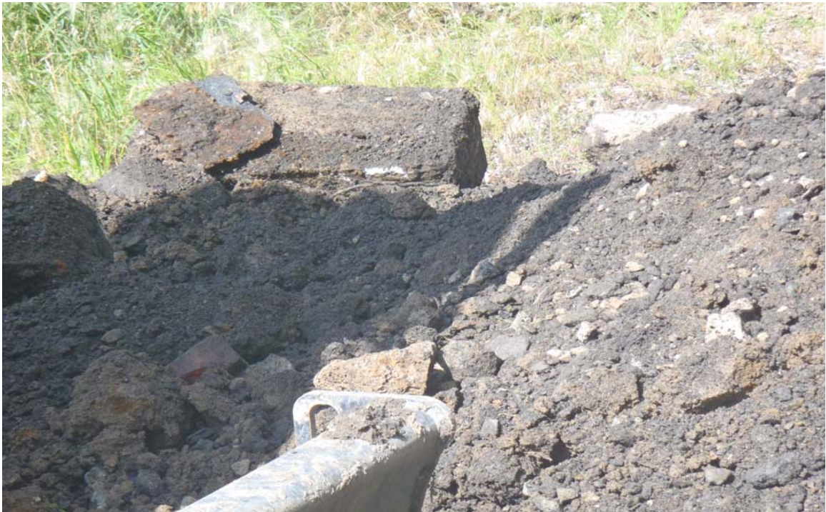
Photograph 10 –Test Pit TP-4 – Typical Fill and Stone Block Removed from Test Pit(s)
