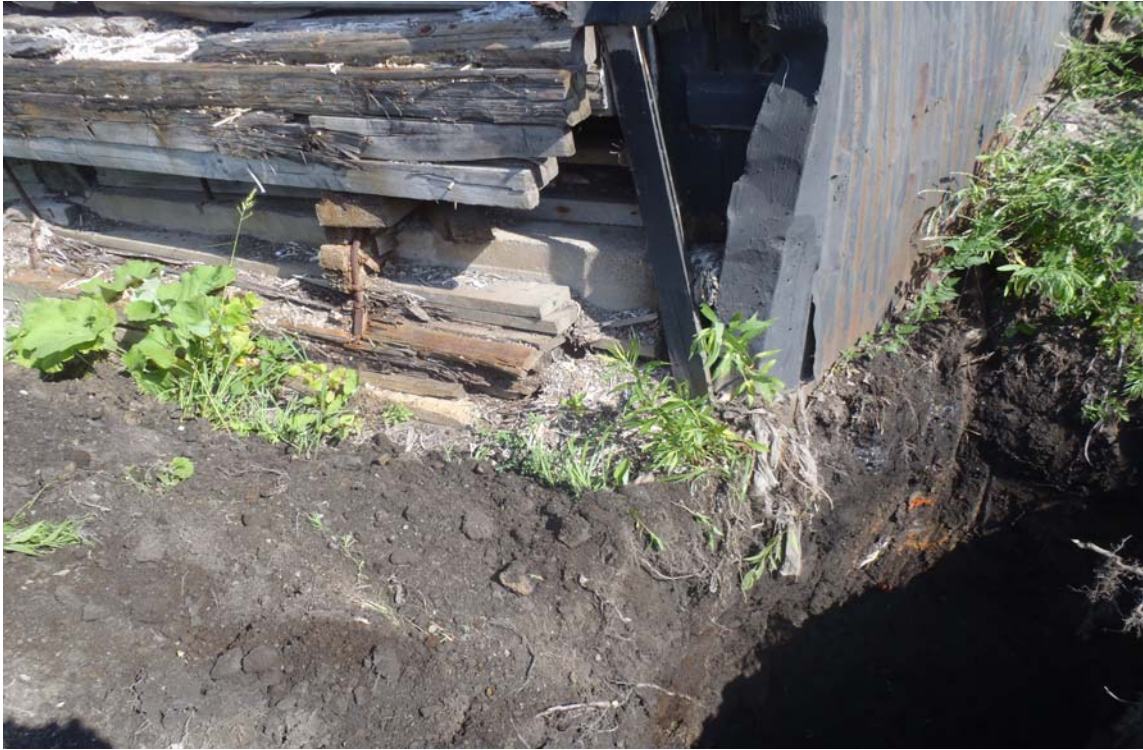
Photograph 5 –Test Pit TP-3 – Northeast Corner of Building
