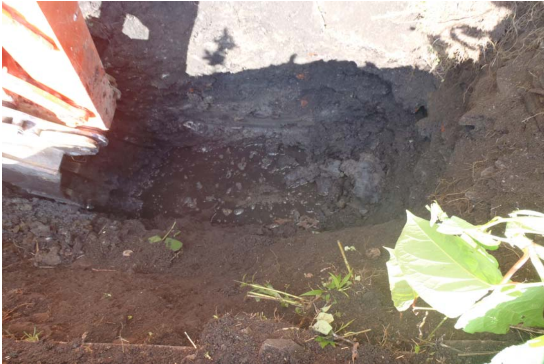
Photograph 1 –Test Pit TP-1 – Stone Block Foundation Wall Exposed – Difficult to observe due to black, organic clayey silt fill.
