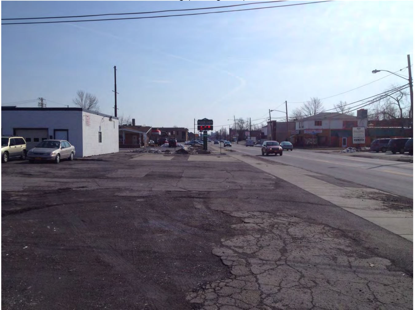
Photo 23: View of former pump islands southeast of the former Western Building and south of the Eastern Building (looking east)
