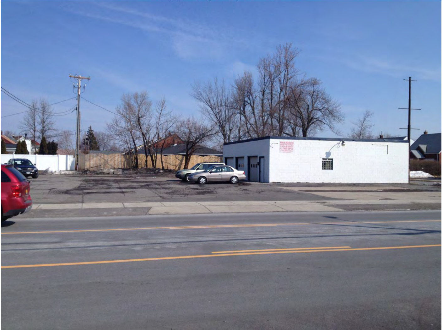
Photo 1: View of the Eastern Building (looking north)
