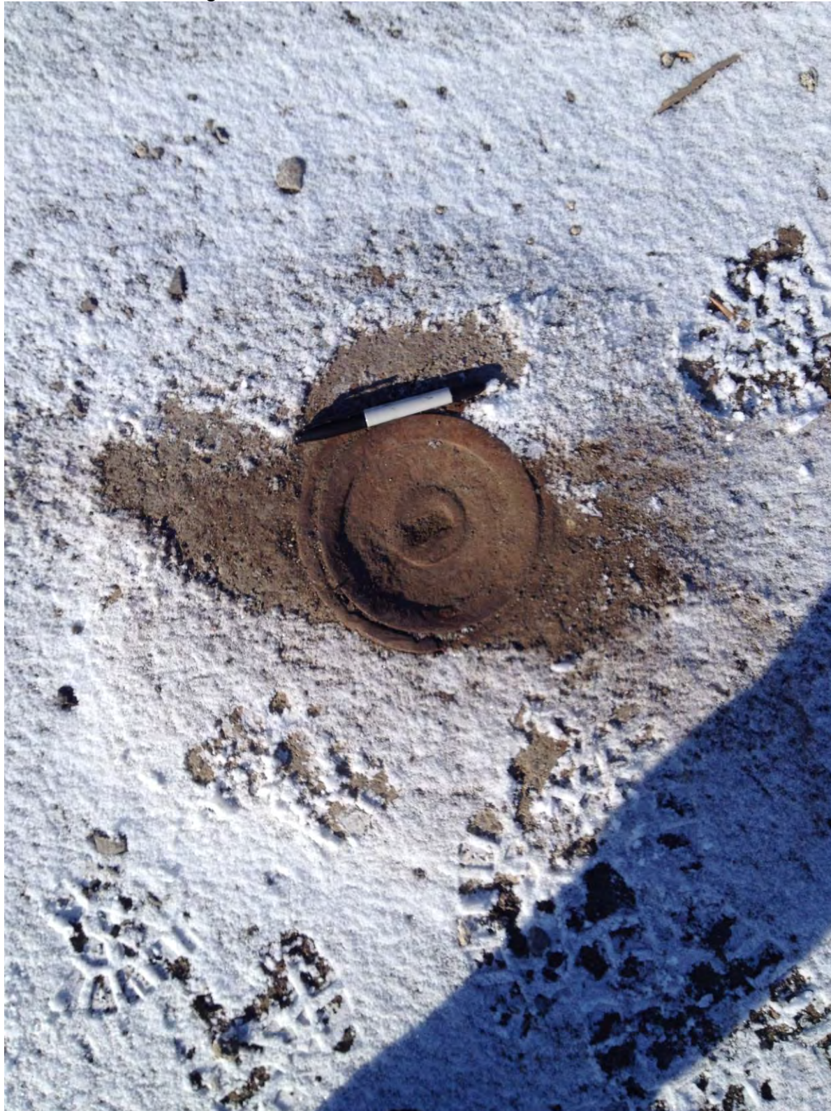
Photo 14: Another view of the fill port on the southeastern edge of the former Western Building
