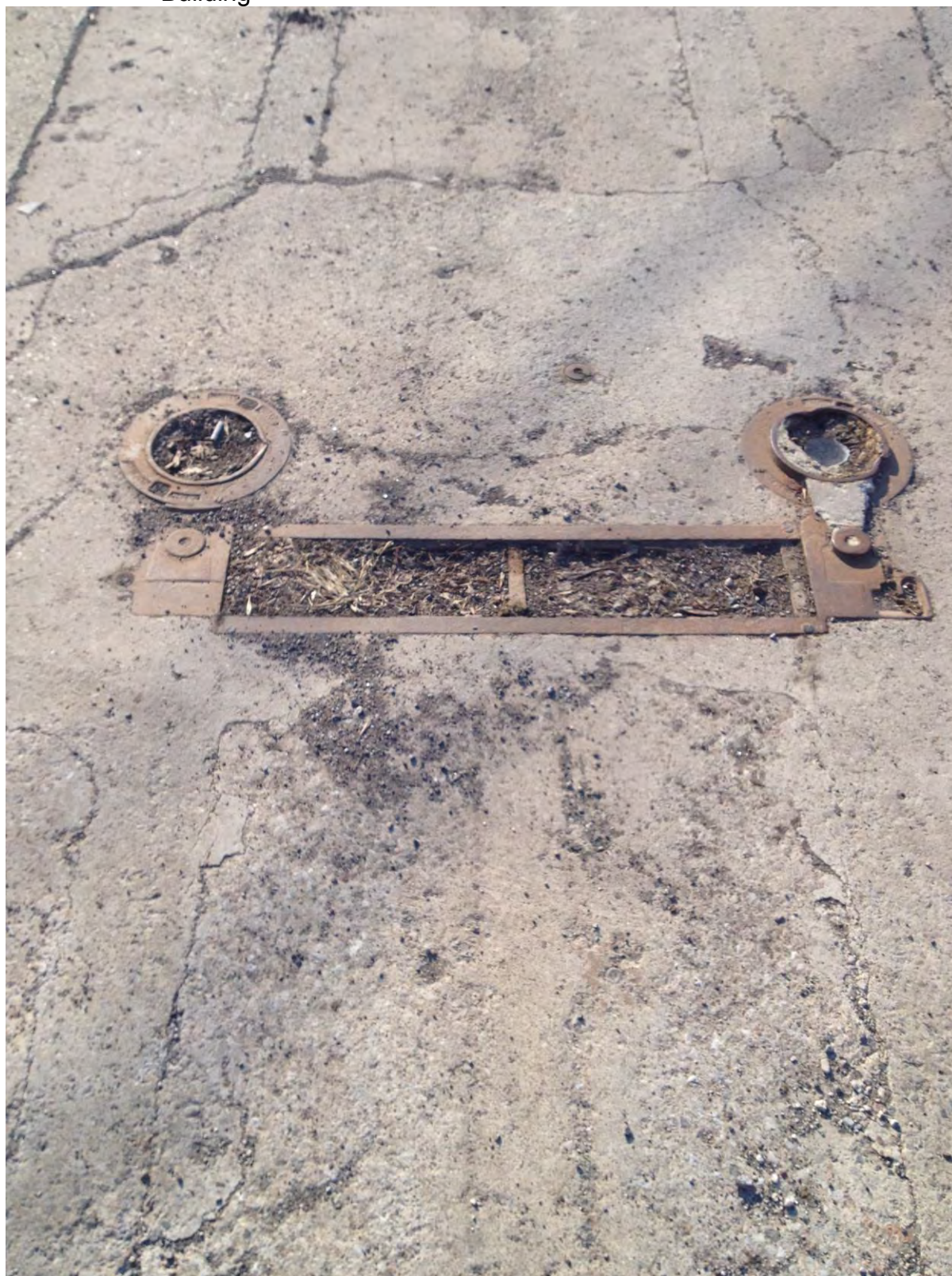
Photo 20: View of a historic in-ground hydraulic lift in the footprint of the former Western Building
