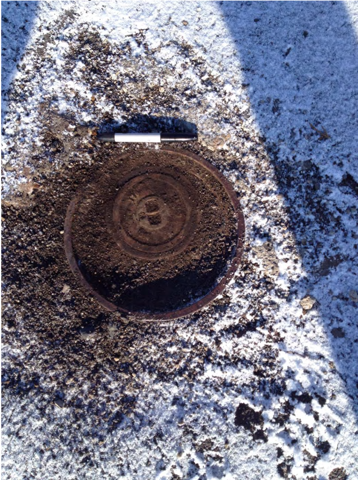
Photo 10: Another view of the fill port on the northwestern edge of the former Western Building
