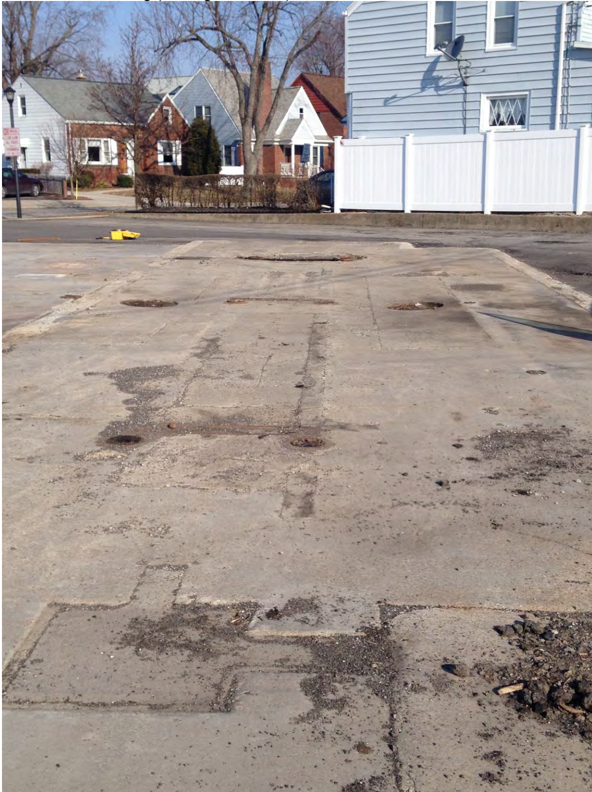
Photo 17: View of 3 historic in-ground hydraulic lifts in the footprint of the former Western Building (looking northwest)
