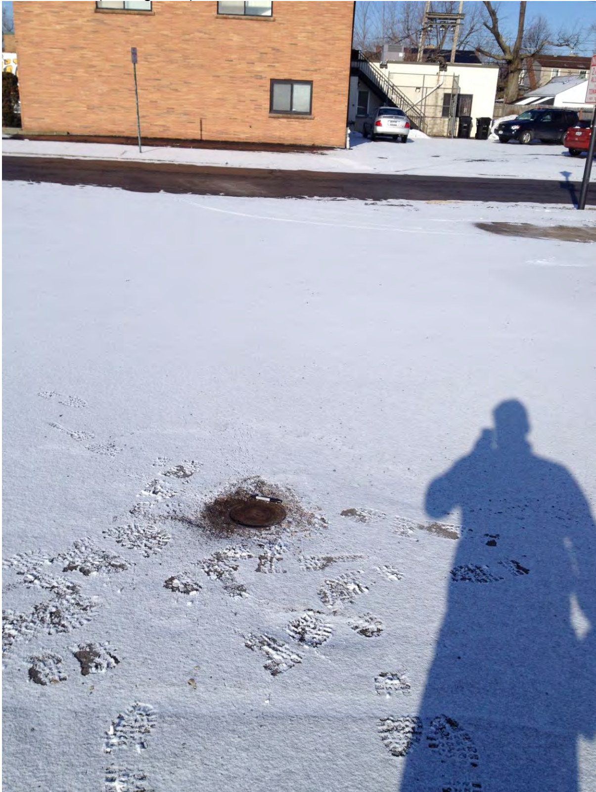
Photo 9: View of a fill port on the northwestern edge of the former Western Building (looking west)
