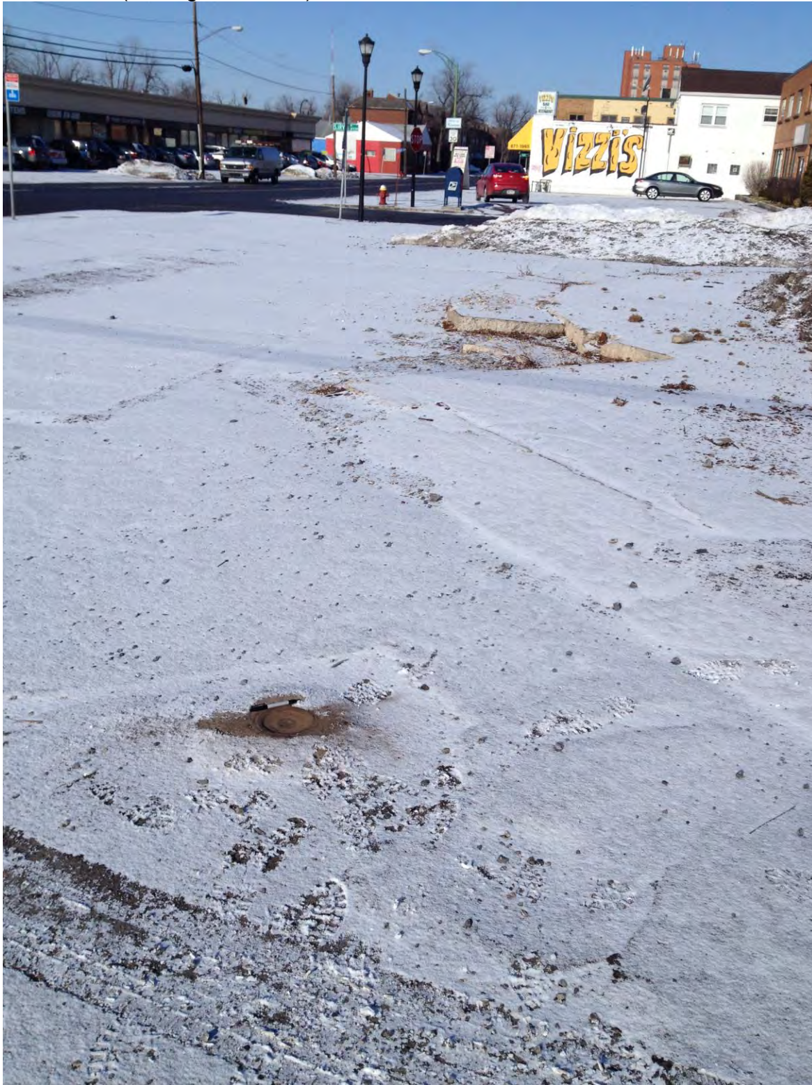
Photo 13: View of a fill port on the southeastern edge of the former Western Building (looking southwest)
