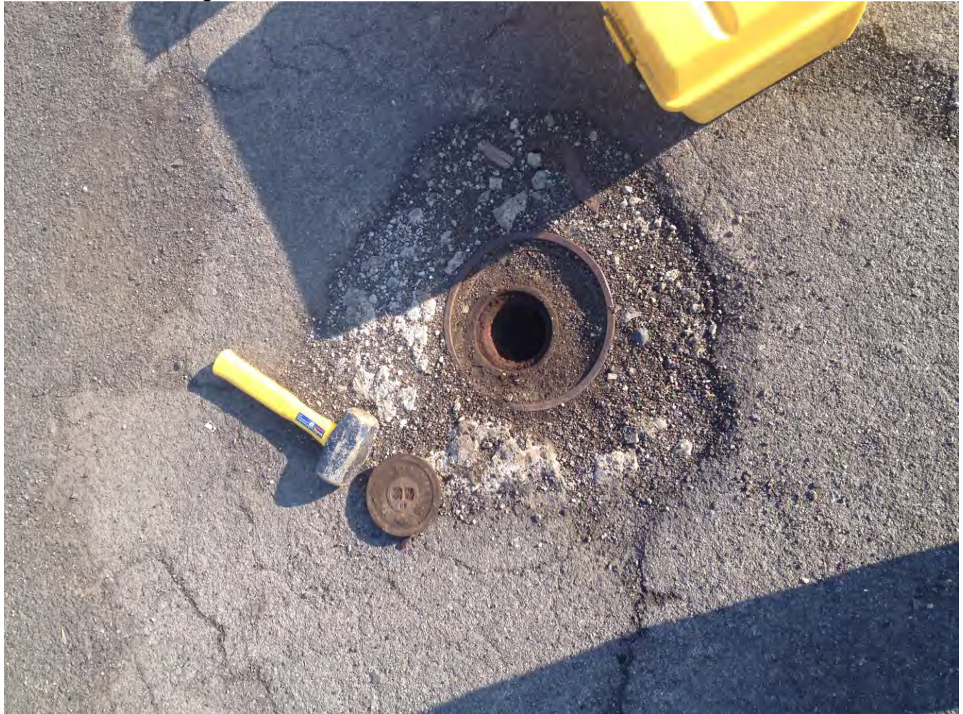
Photo 11: View of the opened fill port on the northwestern edge of the former Western Building
