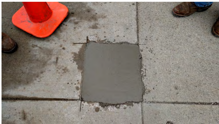
MWB decommissioned and capped with concrete 12/21/15.
