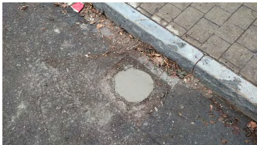
MWA decommissioned and capped with concrete 12/21/15.
