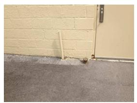
Vent pipe and fill port for heating oil UST on west side of Building 3
