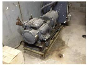
Motor/compressor with staining and drain in old air handling room in basement of Building 4
