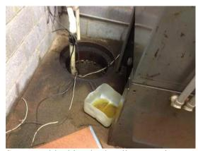
Sump and leaking hydraulic pump in basement of Building 4
