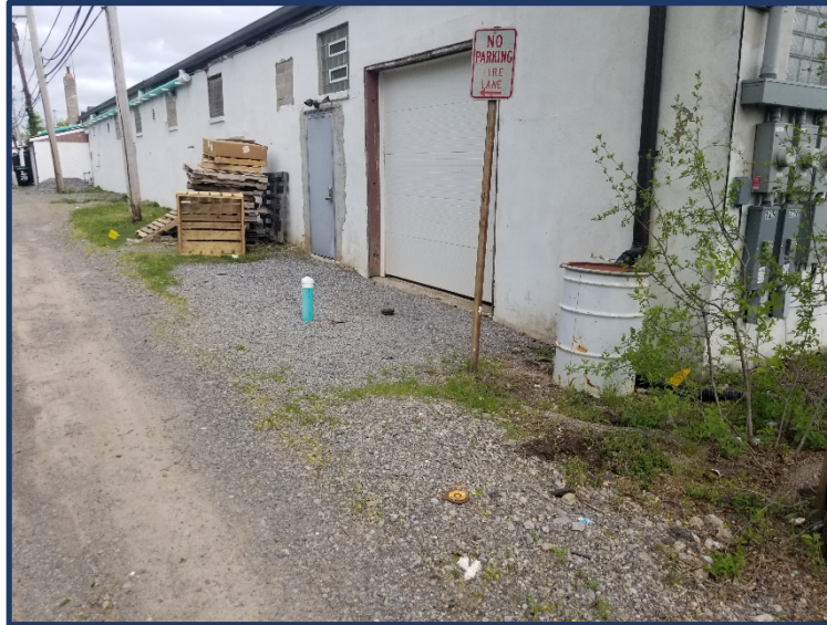
Photo 3 – Soil cover behind building looking west.
