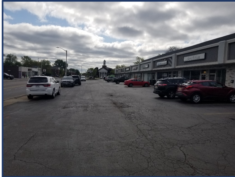
Photo 1 – Front parking lot and sidewalk looking east.
