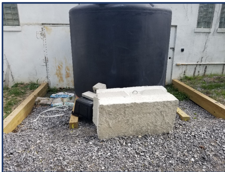
Photo 6 – View of pad underneath water cistern.
