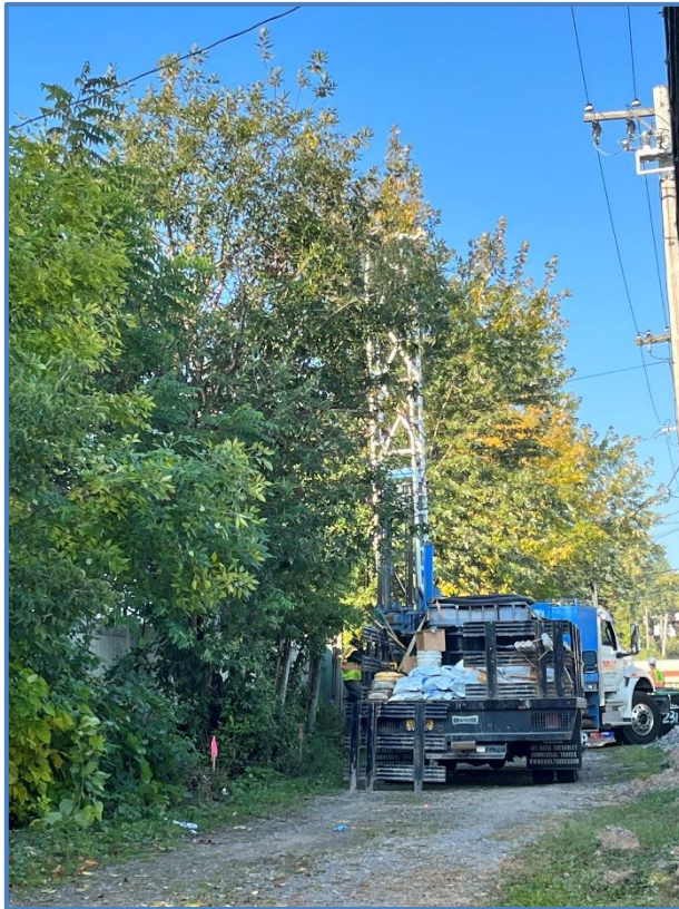
Figure 6-11. Photo showing vegetation at the Highland Plaza Off-Site Area. View looking west. Notice the utility line crossing the service alleyway. Photo taken by Glenn M. May October 3, 2023.
