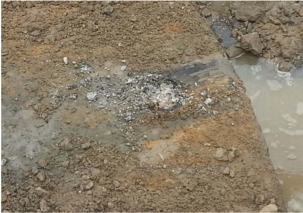
Photo #3 - Close-up of exposed fill port. Note concrete fill.
