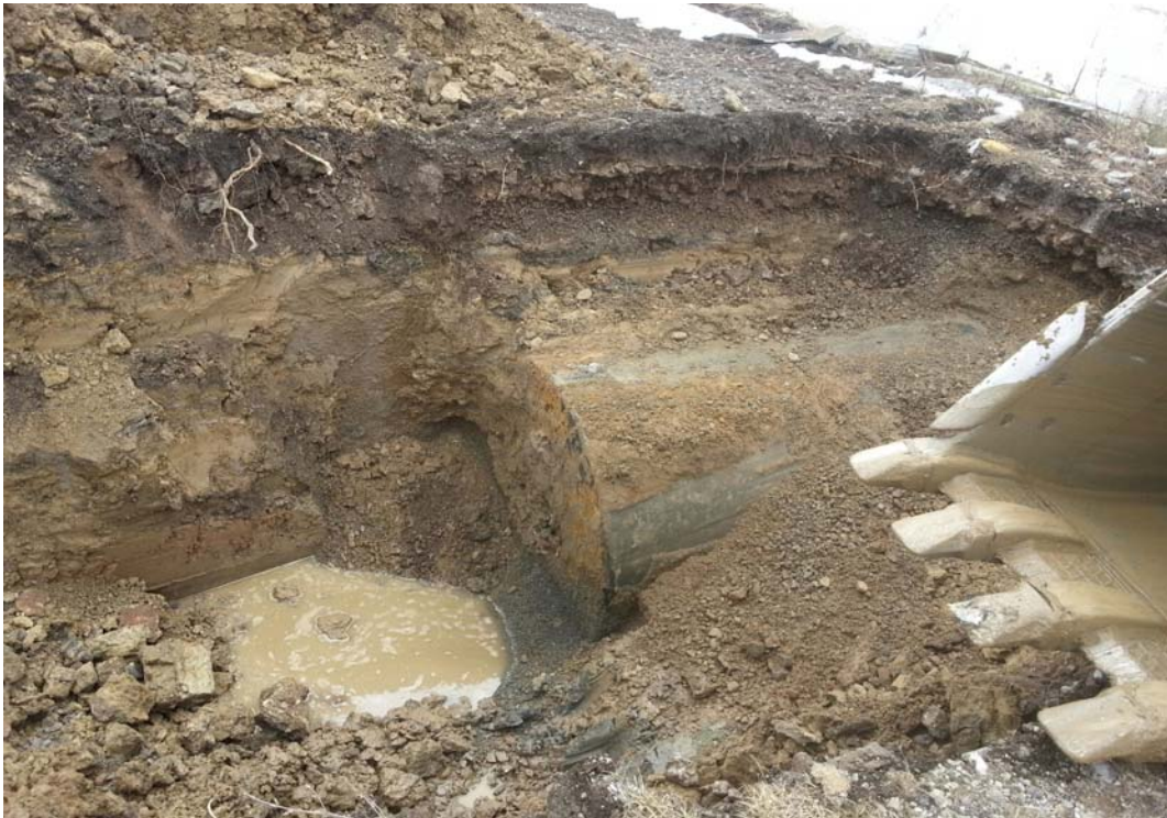
Photo #2 - Abandoned UST in-place
