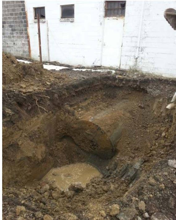
Photo #1 - Abandoned UST in-place
