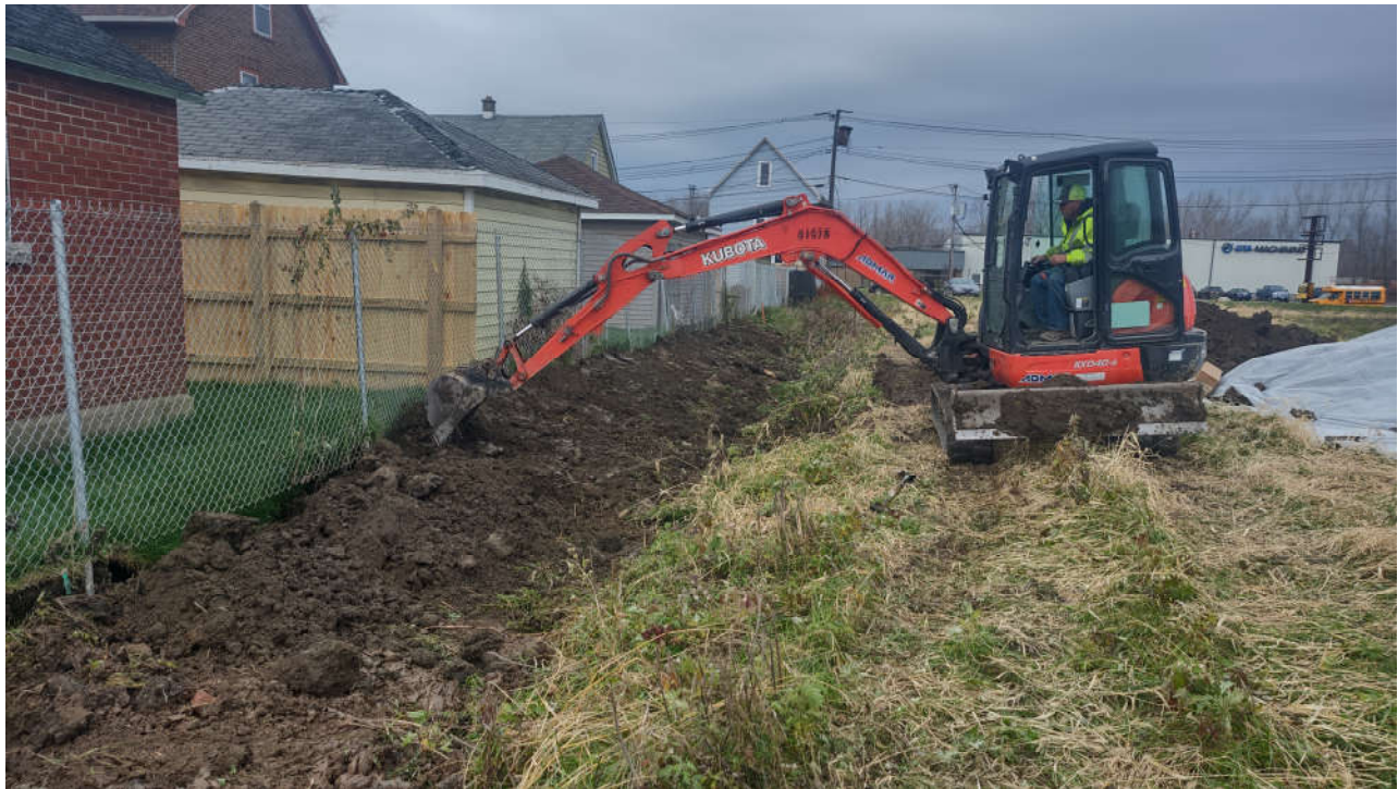
Photo #12: Re-construction of Peru property line excavation
