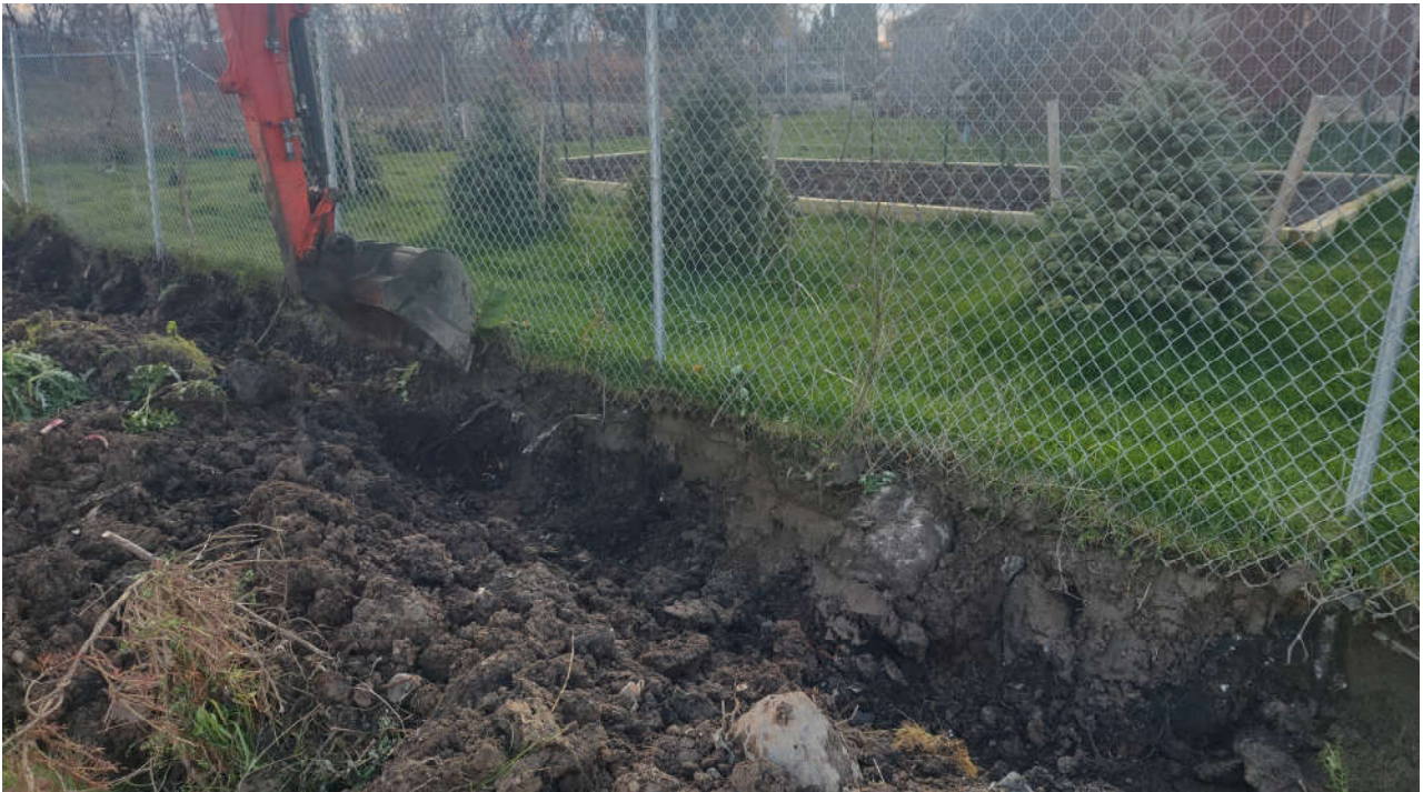
Photo #9: Excavation in progress at Peru property line excavation
