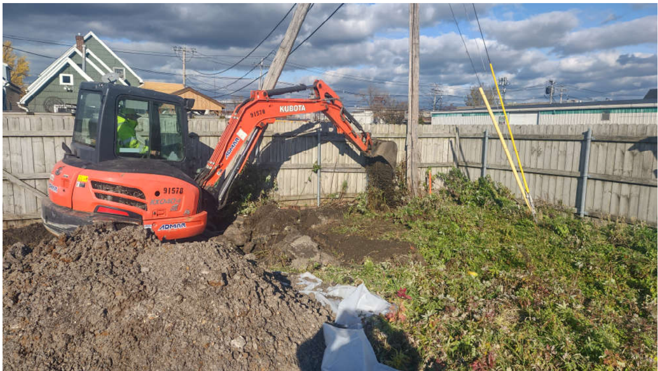
Photo #6: Re-construction of Dingens property line excavation
