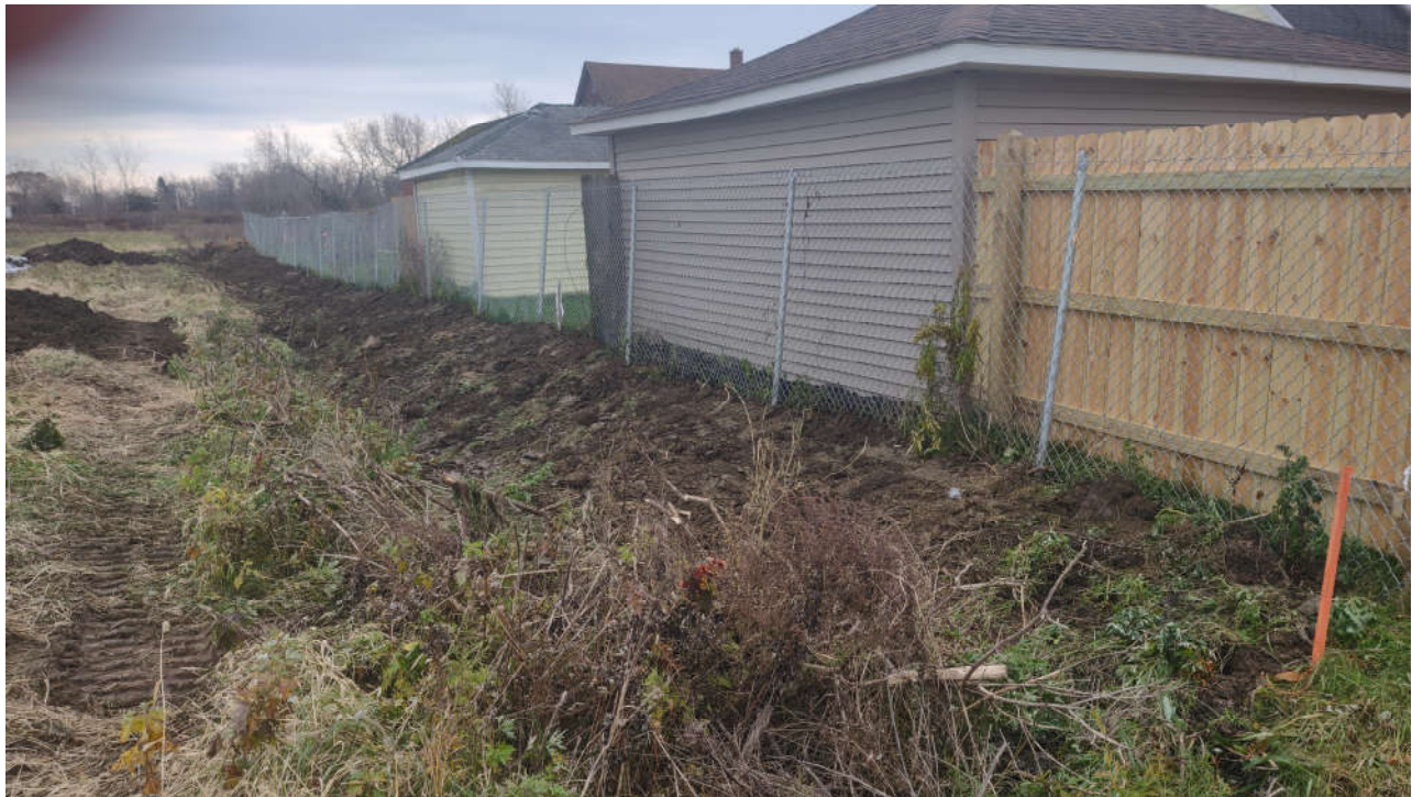
Photo #14: Re-construction of Peru property line excavation
