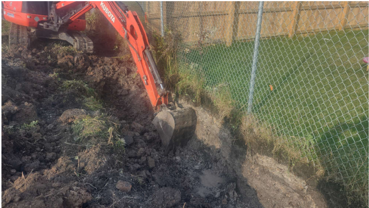
Photo #2: Excavation in progress at Dingens property line
