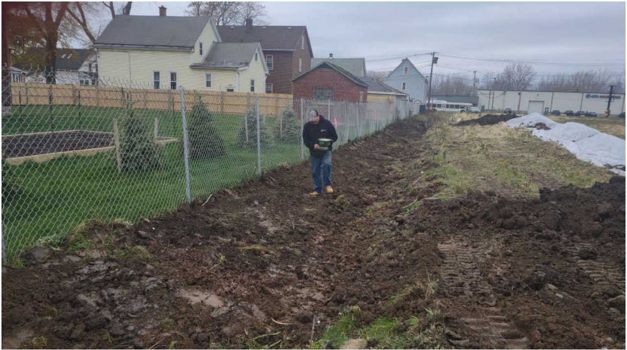
Photo #13: Re-seeding of Peru property line excavation
