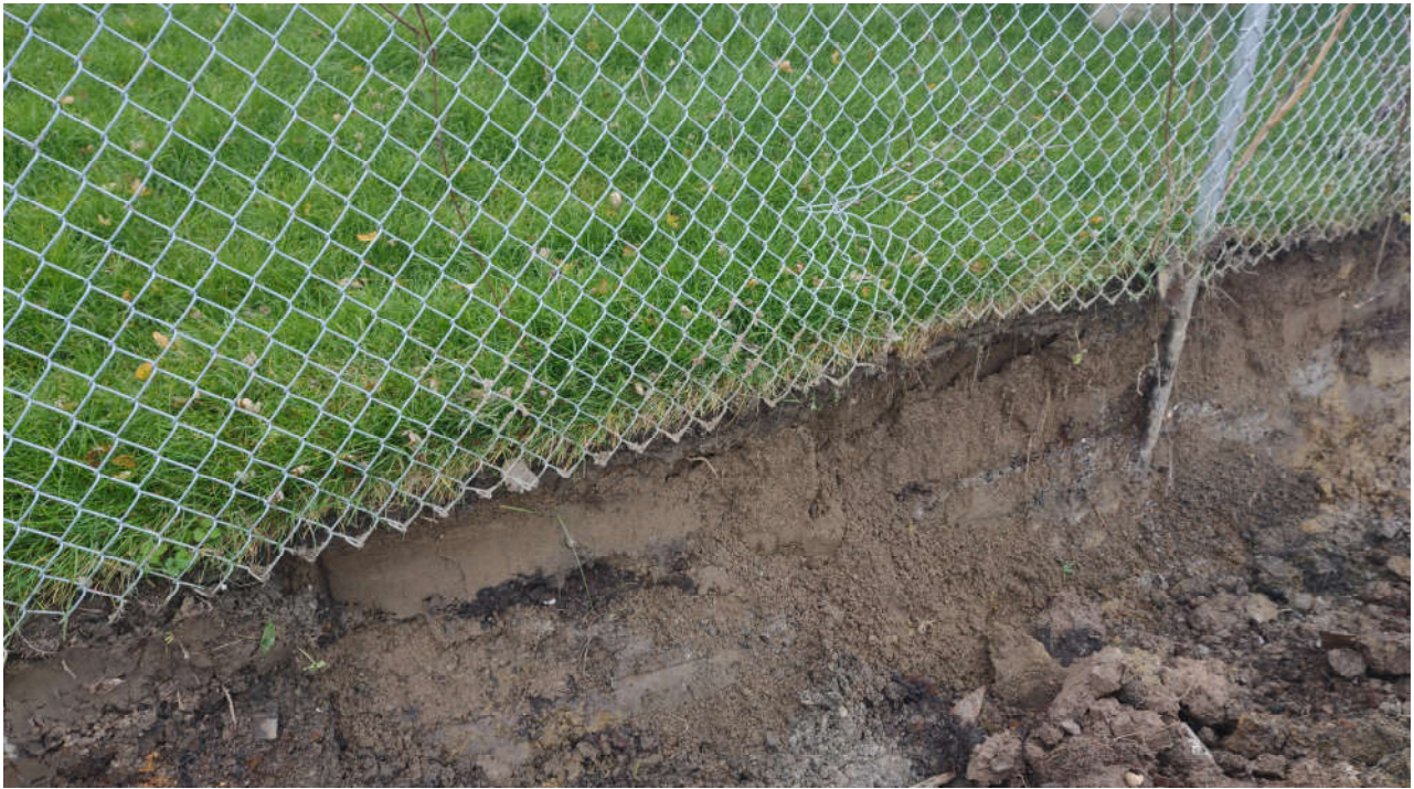
Photo #1: Excavation in progress at Dingens property line
