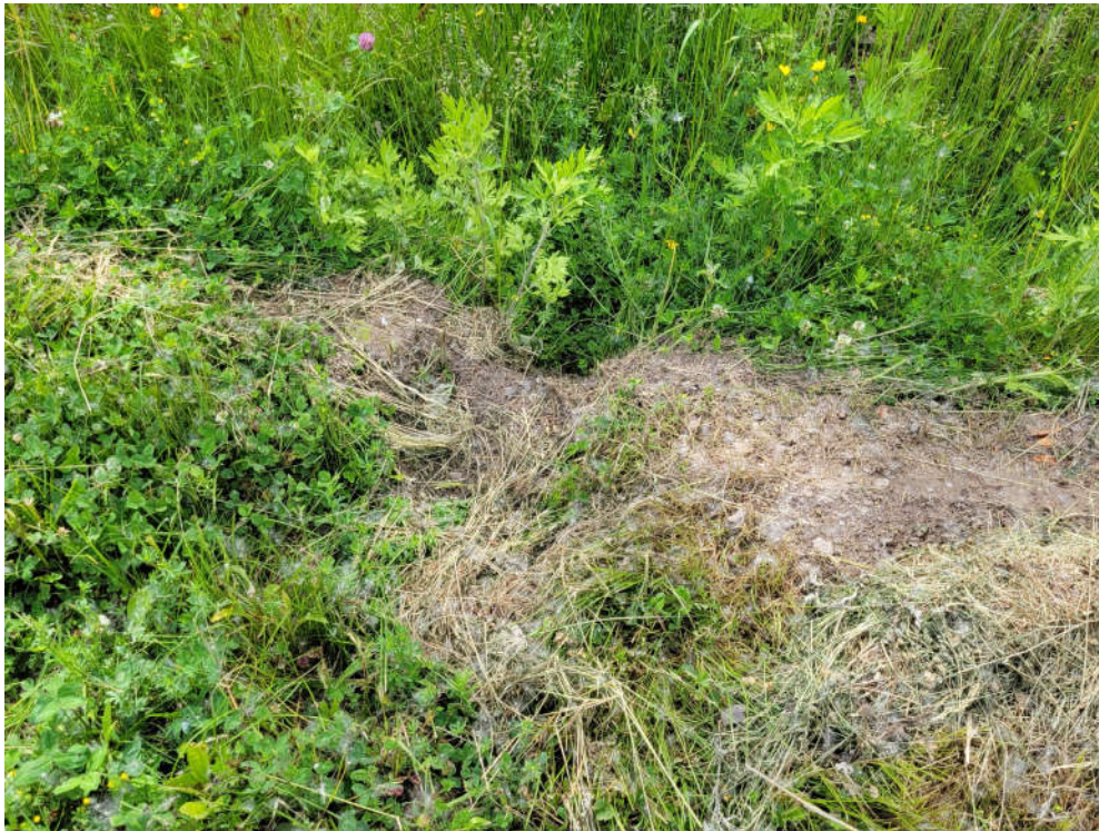
Photo #6: Additional erosion rill.
