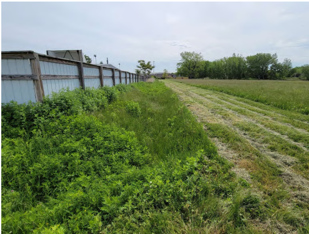
Photo #2: North drainage ditch with vegetation. Fencing remains in good condition.
