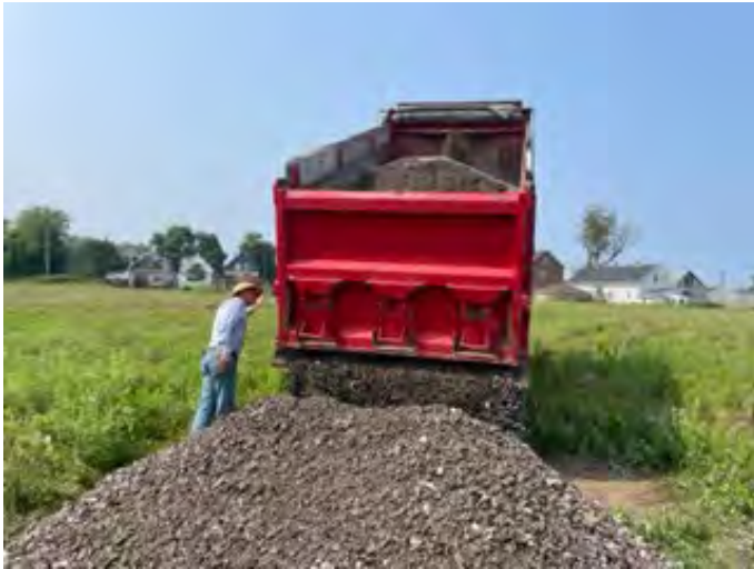
9. Stone being dumped into test pits by dump truck
