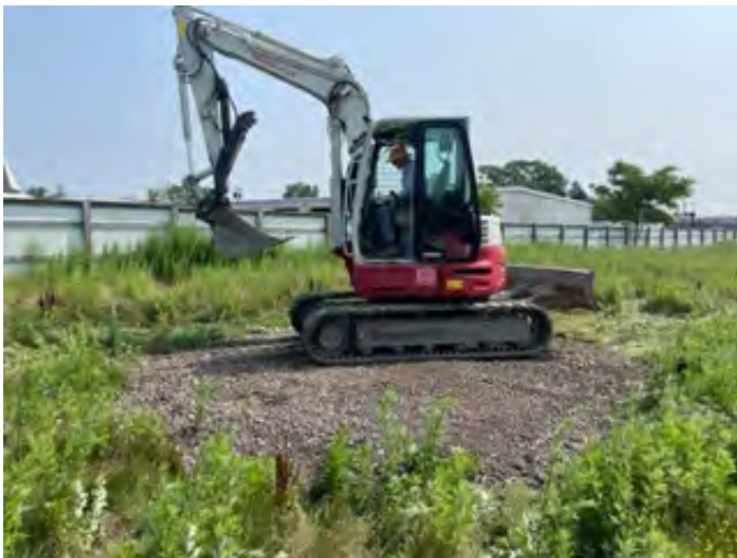
11. Stone being compacted by mini-excavator
