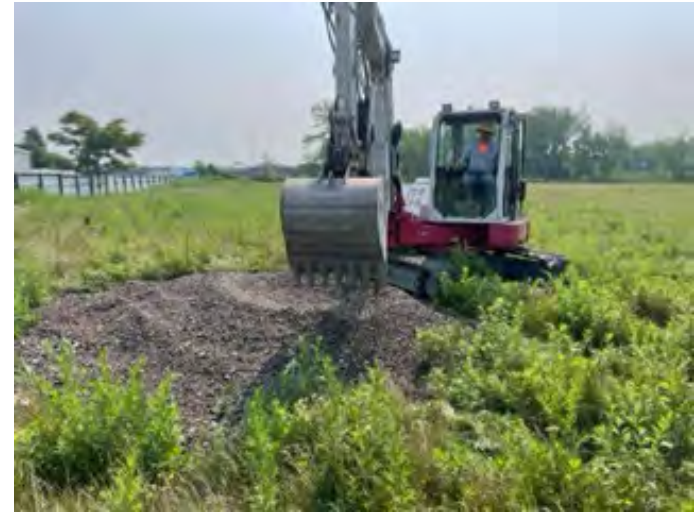
10. Stone being leveled by mini-excavator
