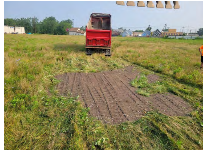
4. Completed backfill of Test Pit 1
