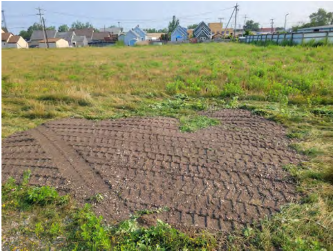
5. Completed backfill of Test Pit 3
