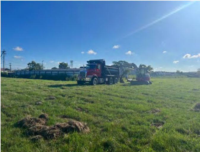
1. View of dump truck holding stone and mini-excavator used to transport and compact stone facing northeast
