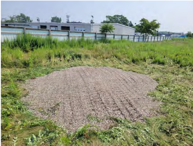
1. Completed backfill of Test Pit 2
