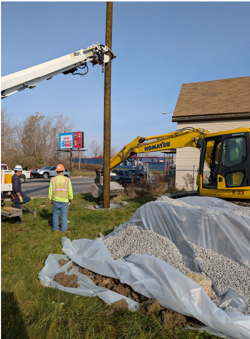
Placing stone base for foundation
