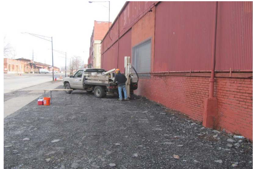
8. Location of borehole 3 facing north
