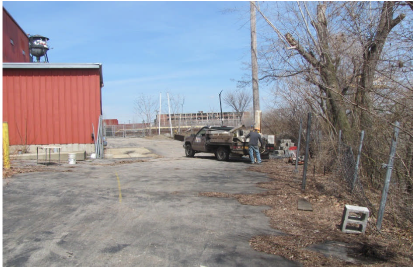
23. Location of BH-8 facing north
