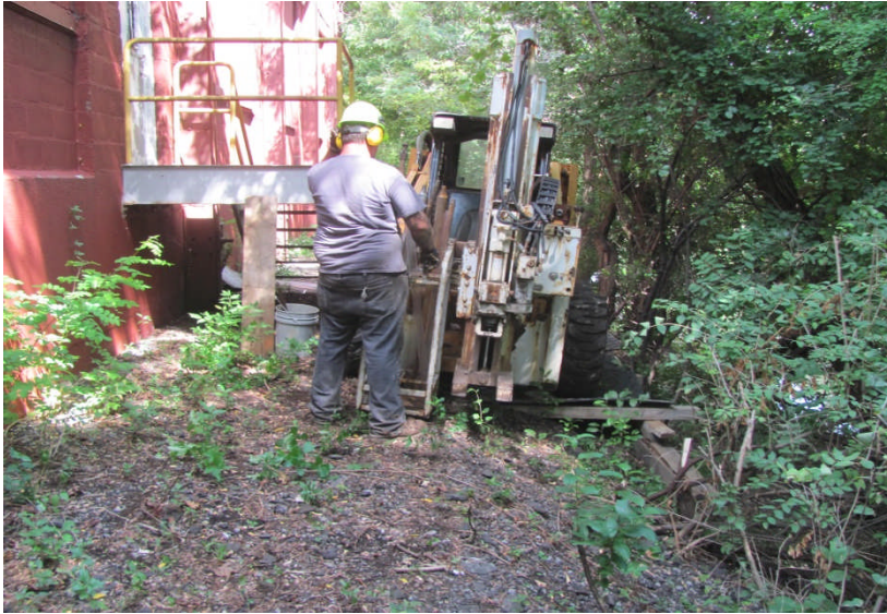
41. Location borehole BH5-4s; 49 feet south of Phase 2 borehole BH-5 facing north
