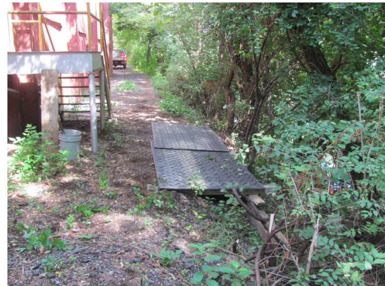
40. Bridge to get around stairs
