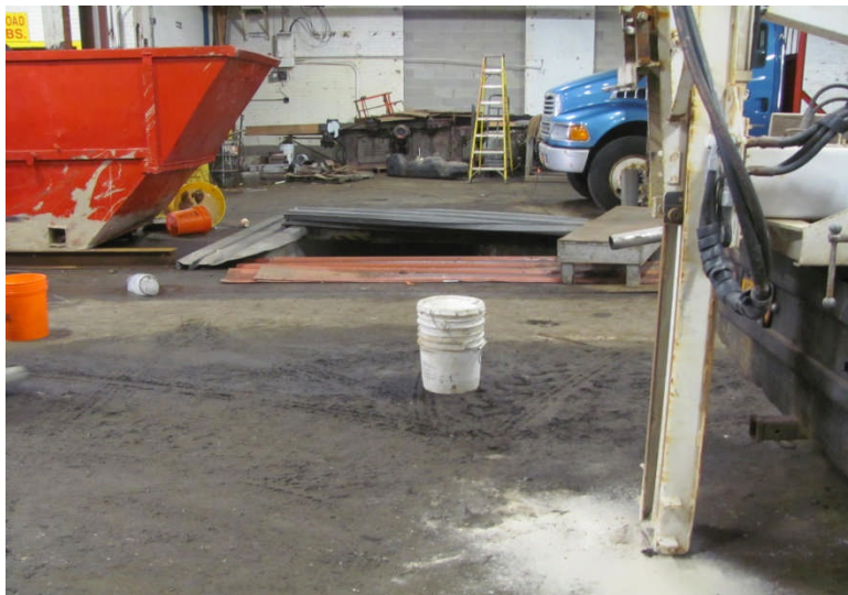
31. Location of BH-10 adjacent to pit area in High Bay area of building
