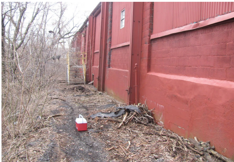
15. Location of BH-5 at cooler; facing south
