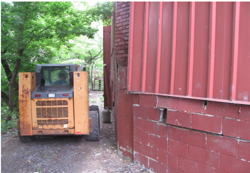
43. Location of borehole BH5-1n facing south
