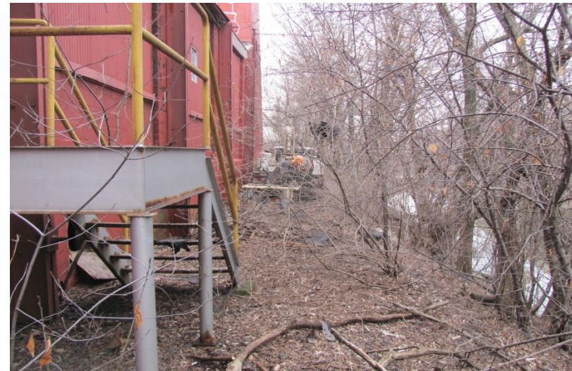
12. Location of Borehole BH-5 facing north
