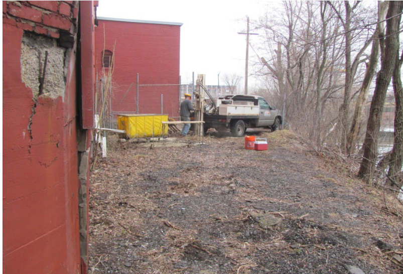
17. Location of BH-6 facing north
