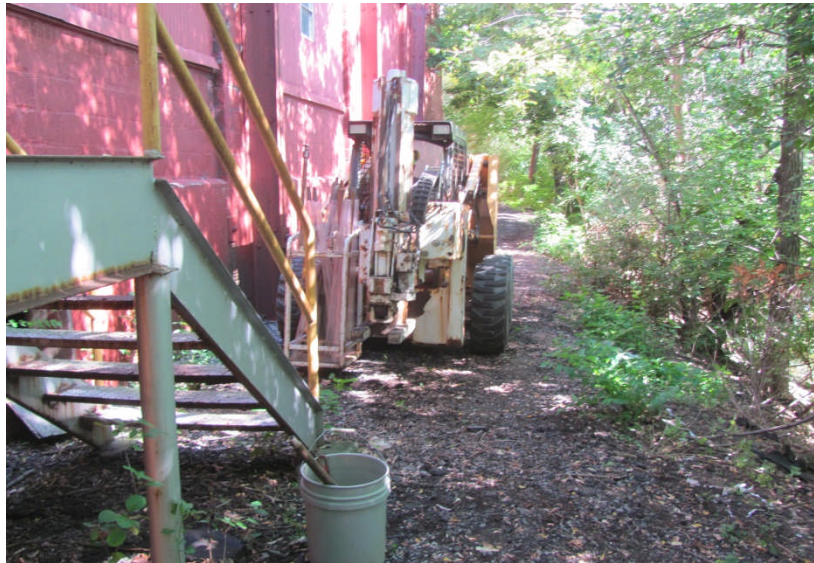
37. Location of borehole BH5-3s facing north; 30 feet south of Phase 2 BH-5
