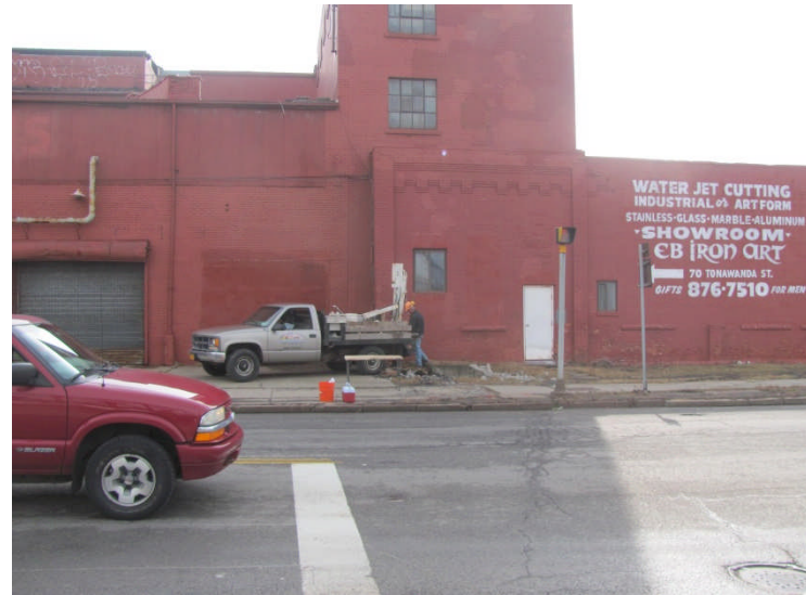
4. Location of borehole BH-2 facing east
