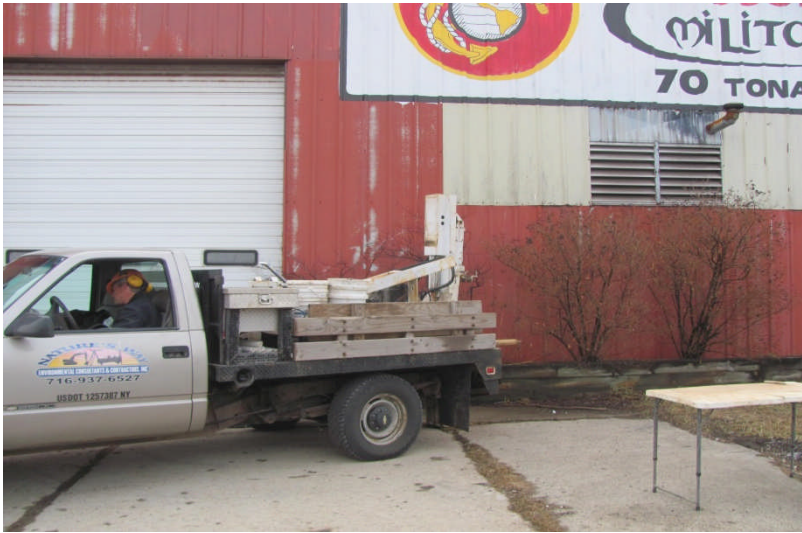
1 location of borehole BH-1 facing east
