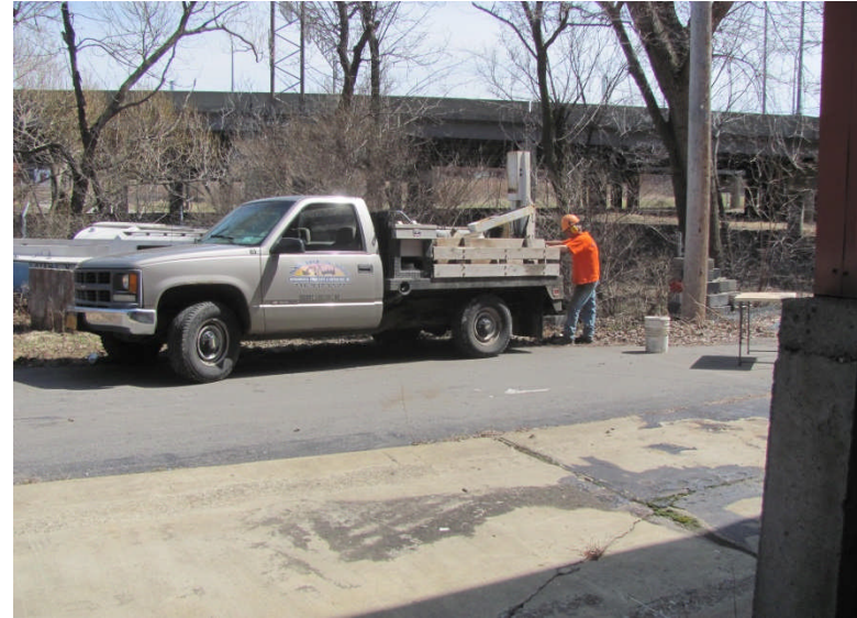
26. Location of BH-9 facing east
