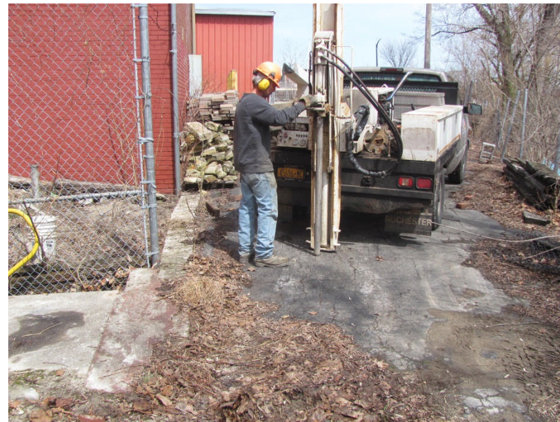
20. Location of borehole 7 facing north
