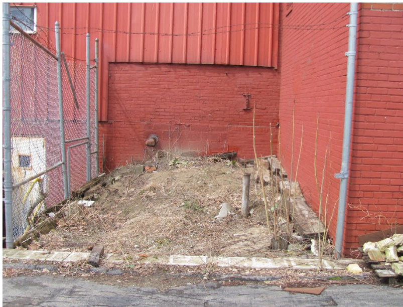
19. Pipe stick-up; west side of building
