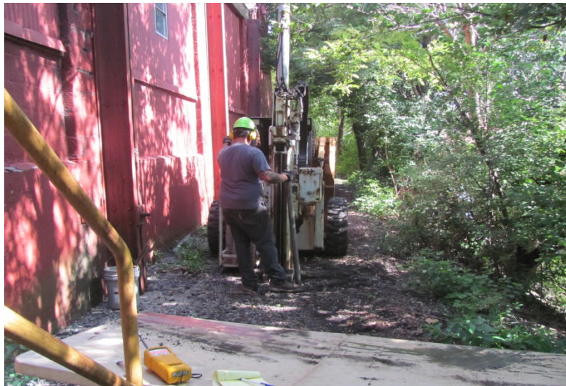
35. Location of BH5-2s; 20 feet south of Phase 2 BH-5 facing north
