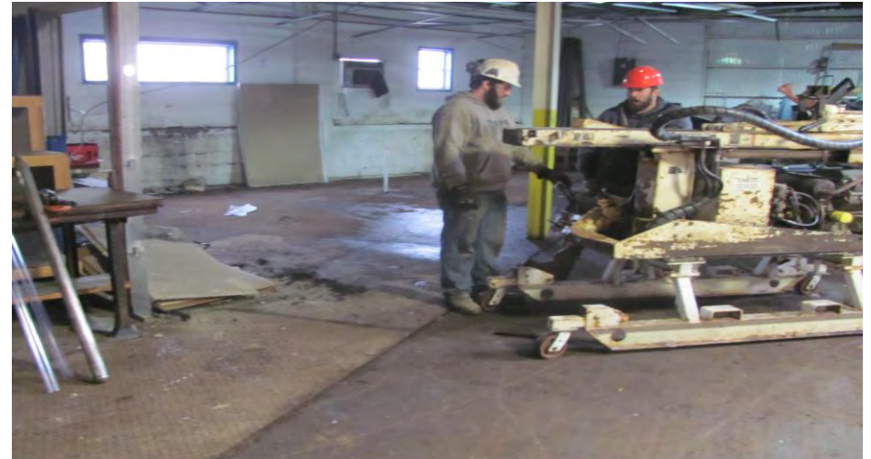
20. Location of Borehole SBH-8 facing southeast
