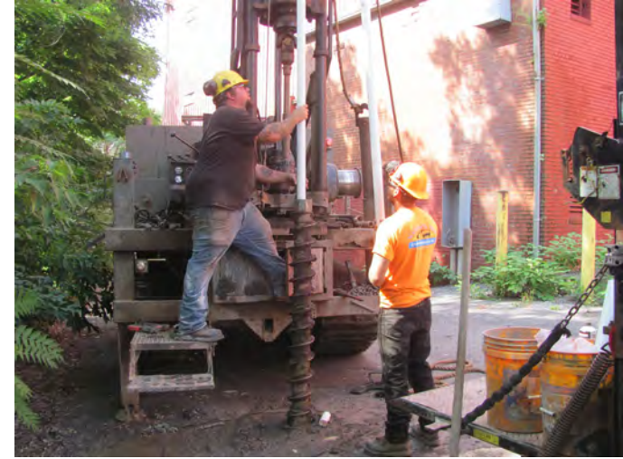
38. 31-MW-4 well installation adjacent creek on east side of property.
