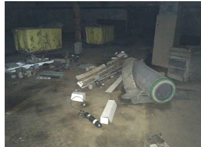
32. SS-05 sample location, middle of basement.
