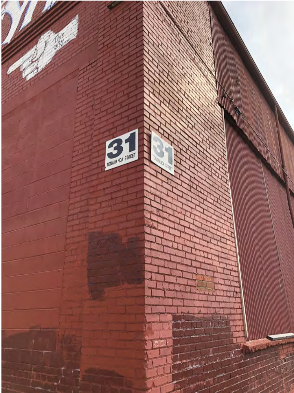
Exterior View of Building
