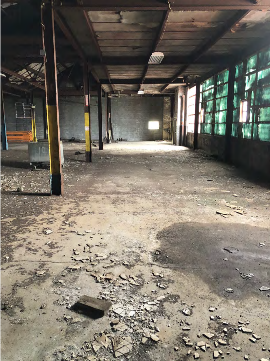
View of Building Interior
