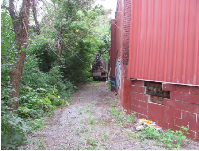
37. 31-MW-3 Well install location, adjacent creek, southeast edge of property.
