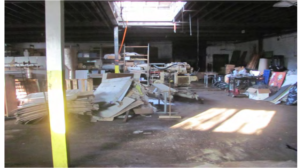
2. View of location of SBH-1 from east facing west
