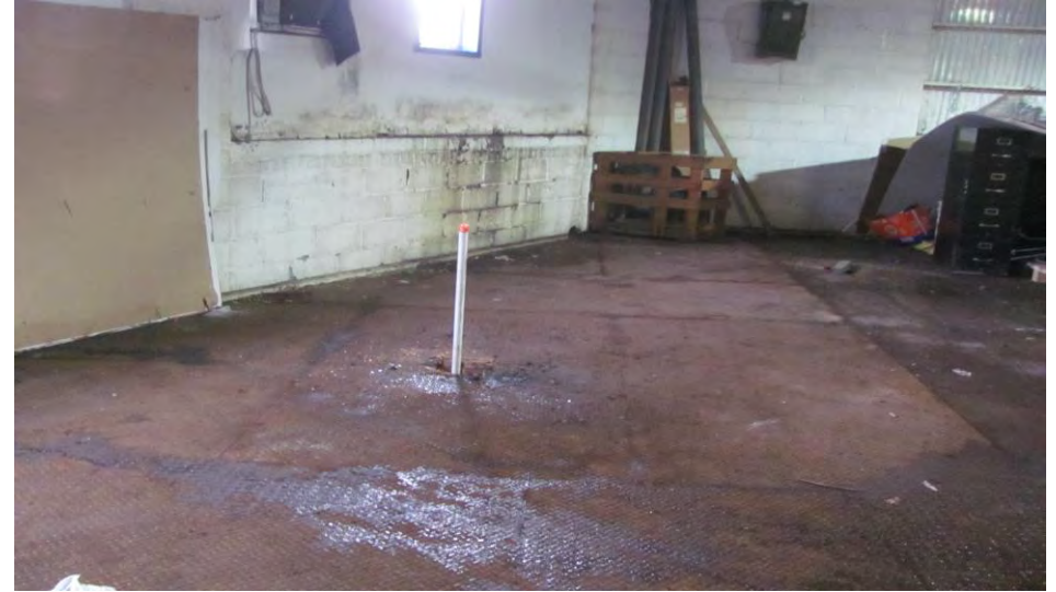
22. Well installed in SBH-3
