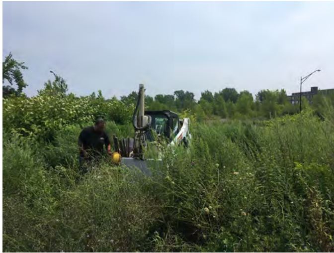
5. BH-3 soil boring location, looking east.
