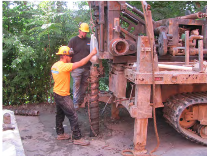
39. 31-MW-4 well installation. No. 0 sand used for filter pack.
