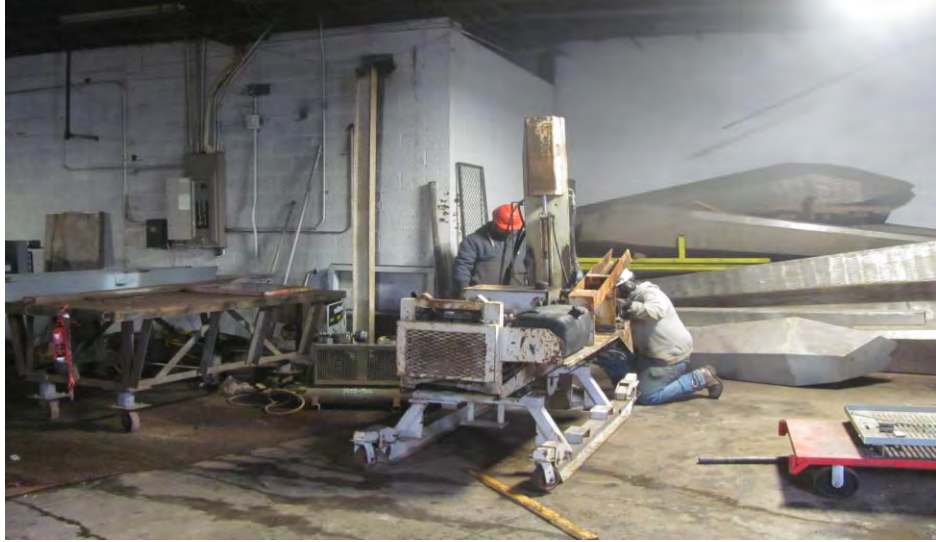
17. Location of SBH-6 facing north
