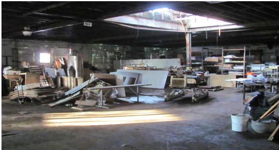
3. Location of SBH-1 from east facing southwest
