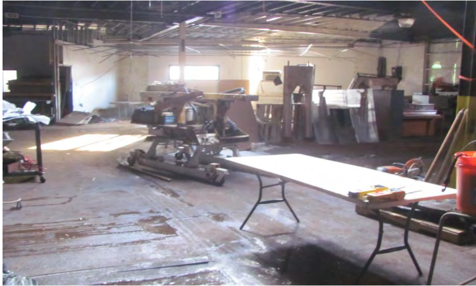
1. Borehole SBH-1 location; from west end facing east
