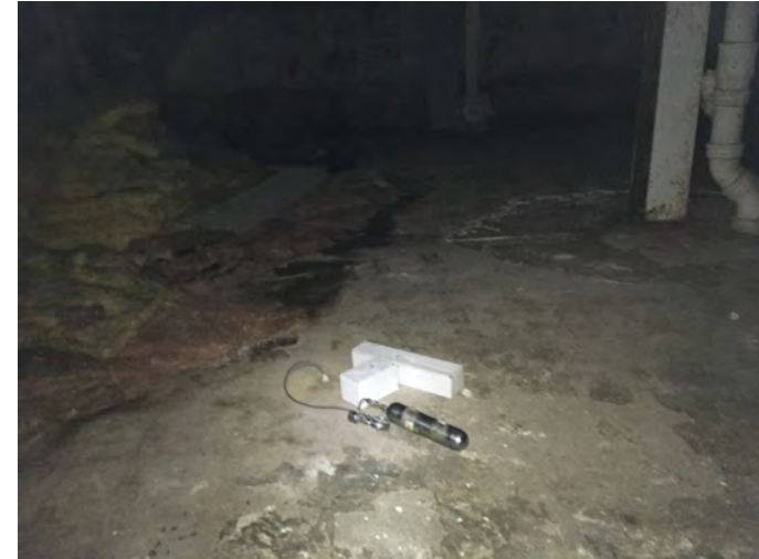
30. SS-04 sample location, northern end of basement.
