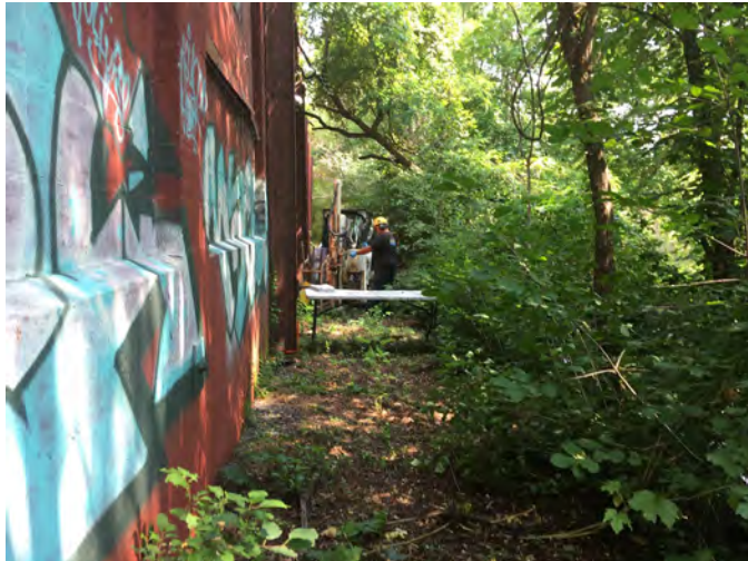
19. BH-1 boring location, looking northeast.
