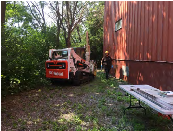
17. BH-2 boring location, looking south.
