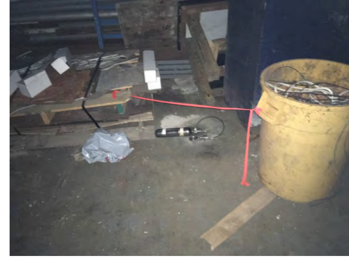
26. SS-02 sample location, middle of high bay slab on grade.
