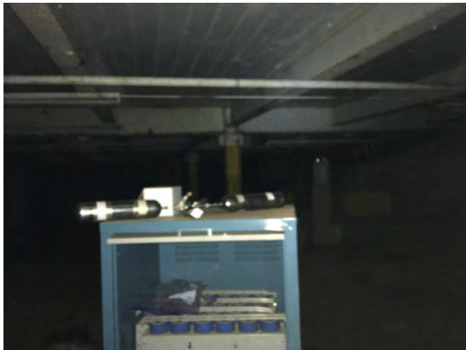
31. IA-04 sample location, northern end of basement.
