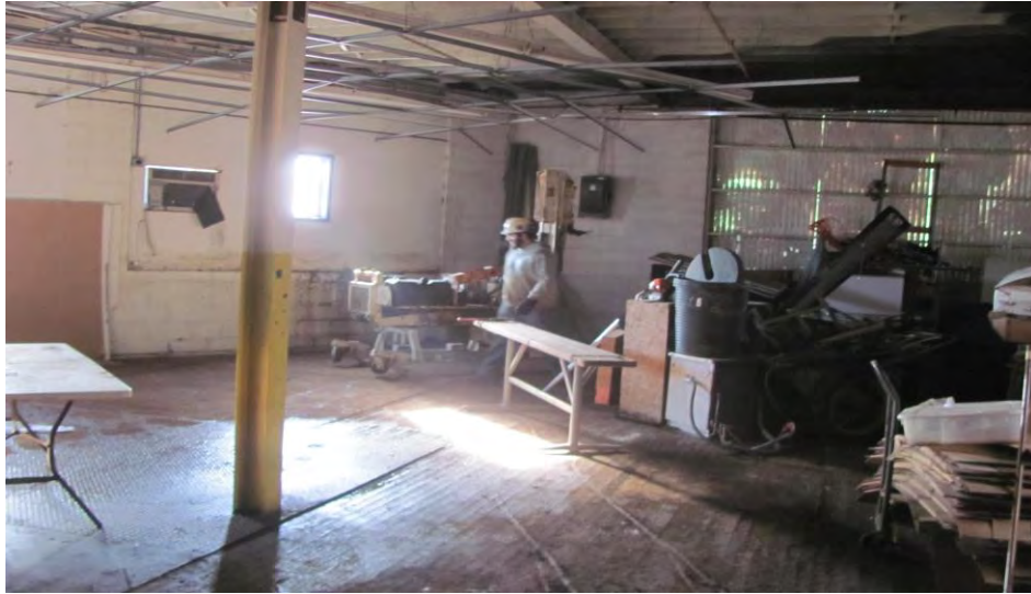
5. Location of SBH-2 facing southeast – in southeast corner of building
