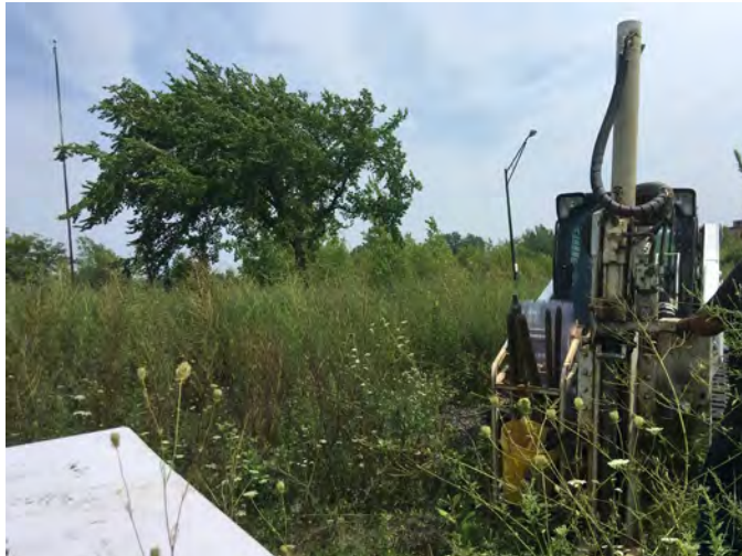
7. BH-4 soil boring location, looking east.
