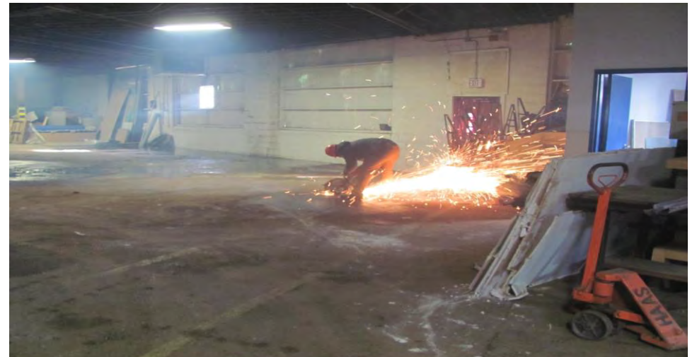
8. View of cutting metal for SBH-5
