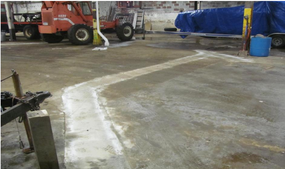
7. SSDS completed trench and vertical piping
