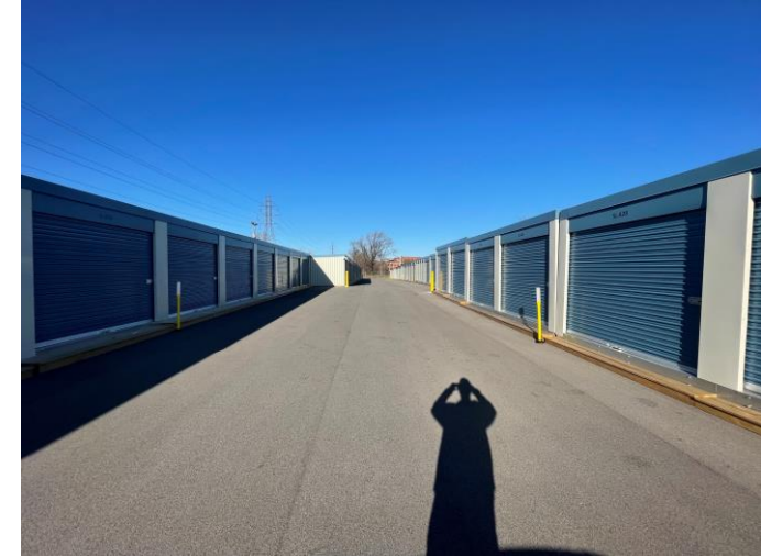
Facing south from middle of driveway that leads through the self storage units.
