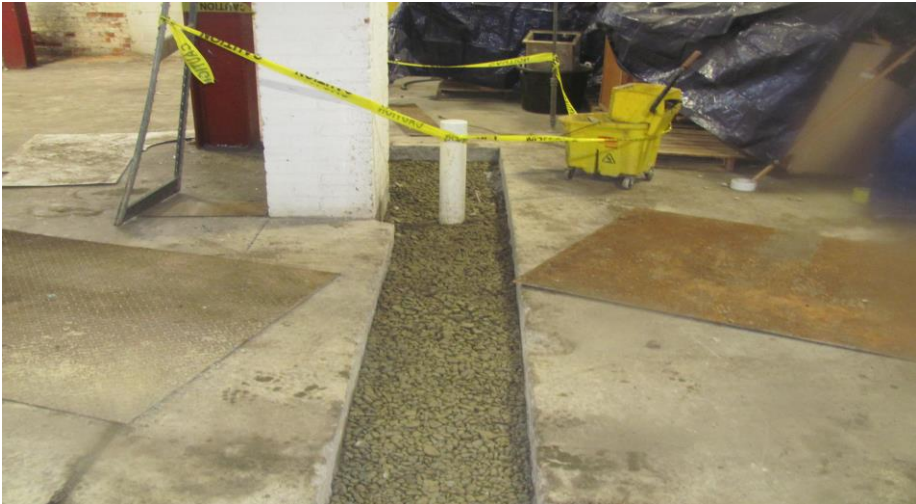
3. Installation of SSDS in High-Bay area
