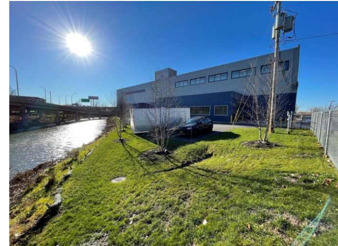
Facing southwest looking at soil and grass cover system located east of the building at 31 Tonawanda.
