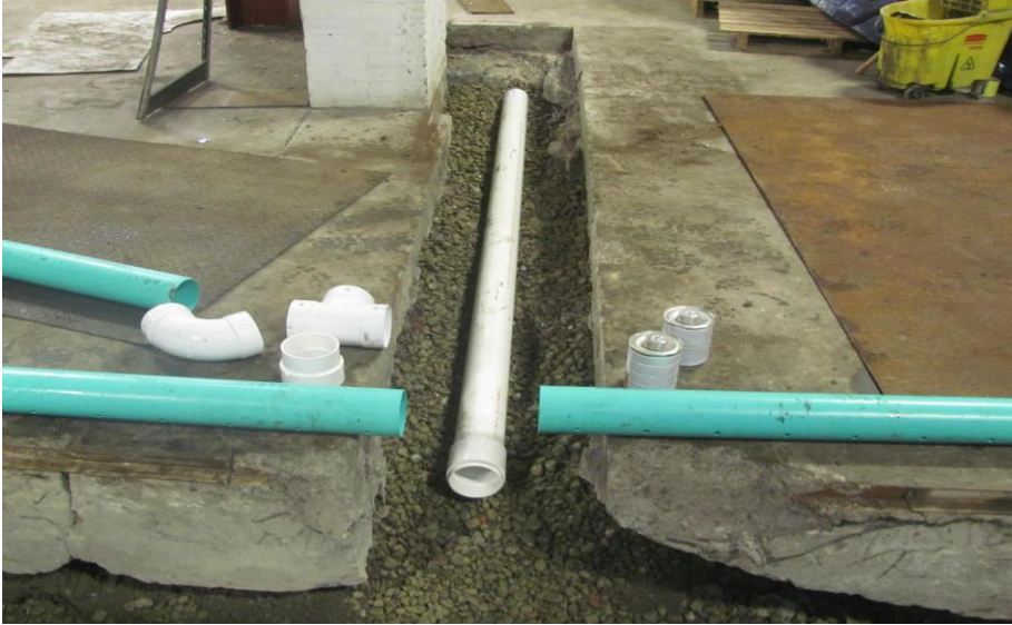
5. Installation of SSDS in High-Bay area
