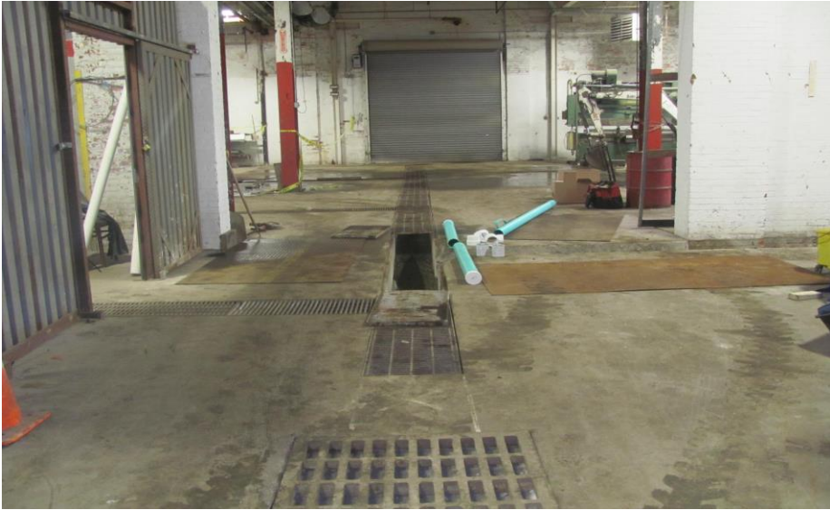
1. Installing SSDS in High-Bay area of building
