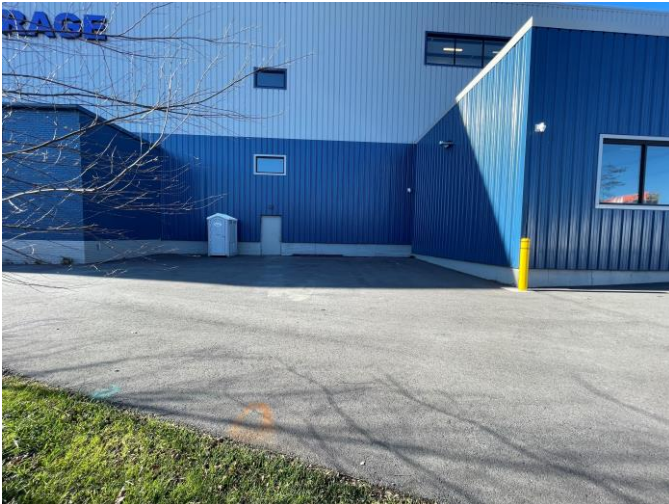
Facing west looking at asphalt cover system located east of the building at 31 Tonawanda.
