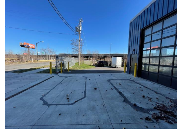
Facing east looking at cover system next to loading dock at 31 Tonawanda.
