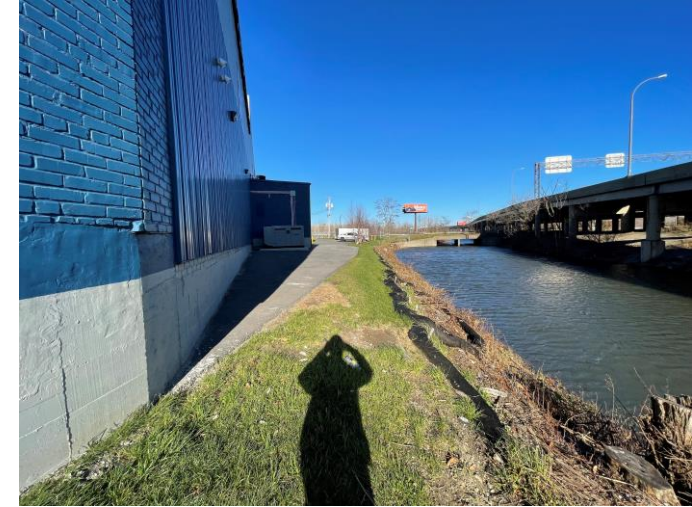
Facing north looking at soil and grass cover system located east of the building at 31 Tonawanda.
