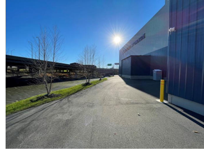
Facing south looking at asphalt cover system located east of the building at 31 Tonawanda.
