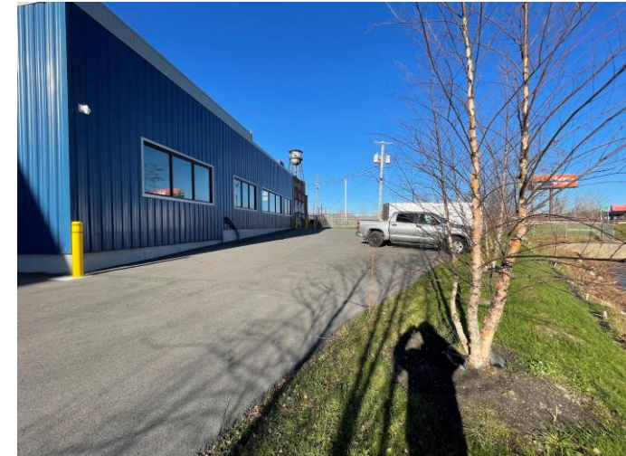
Facing north looking at soil and asphalt cover system located east of the building at 31 Tonawanda.
