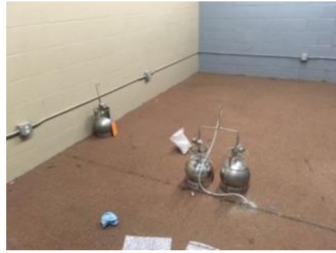
Image 7: Sub-slab Summa Canisters Sample Location: Room #10
