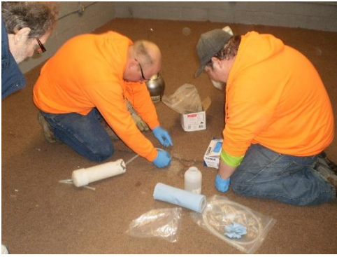
Image 6: Installation of Sub-slab Summa Canisters Sample Location: Room #10
