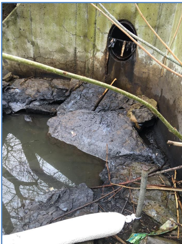
Figure 4-9. Photo showing the oily residue that coats the rocks at the Niagara Street pumphouse discharge area. Photo taken on May 3, 2019 by unknown.
