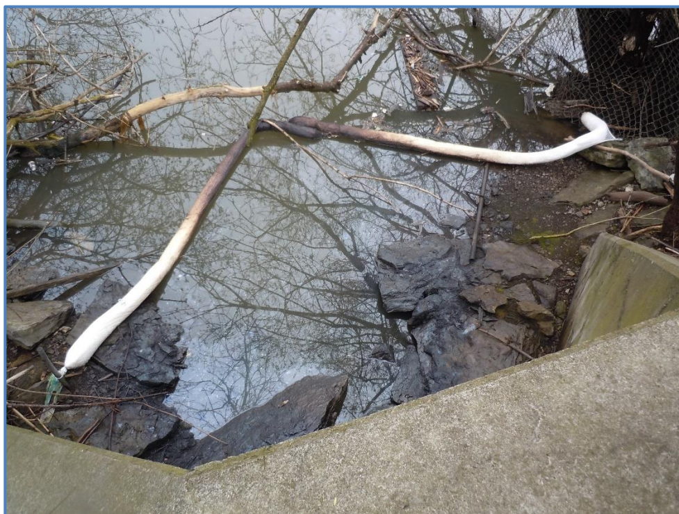
Figure 4-10. Photo showing the oil booms placed at the Niagara Street pumphouse discharge area to absorb any NAPL pumped into the creek. Photo taken on May 3, 2019 by unknown.
