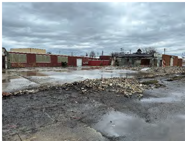
Photo 2: Remaining 1746 Dale Road building (right) and 24 Anderson Road building (background); looking northeast.
