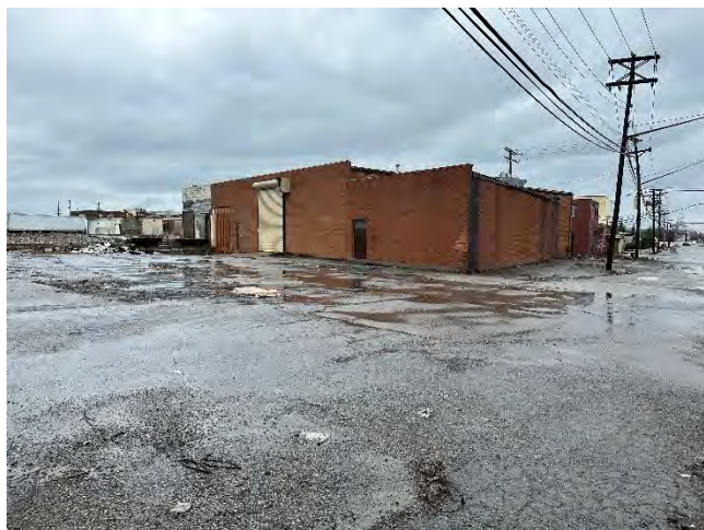
Photo 1: Remaining 1746 Dale Road building to be demolished, looking northwest.
