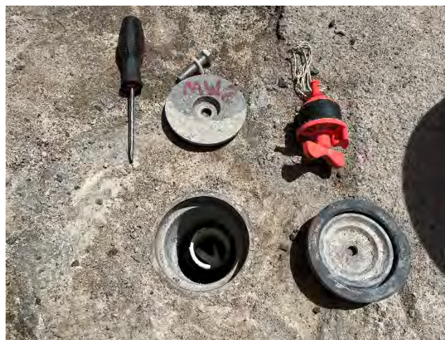
Photo 8: Newly installed Remedial Investigation groundwater monitoring well MW-2.
