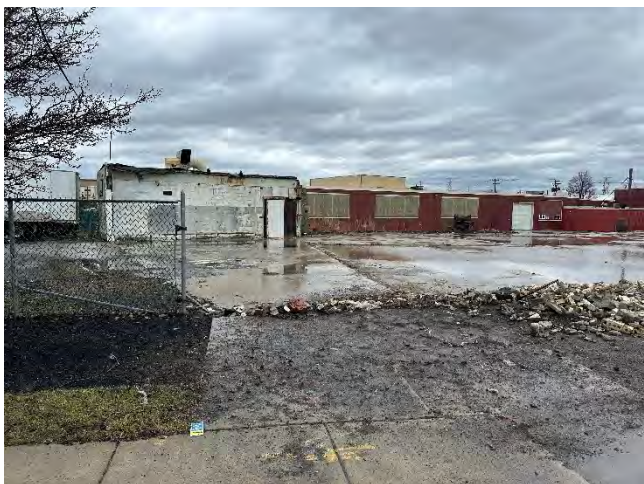
Photo 3: 1746 Dale Road Metal Prep Building (left) and 24 Anderson Road Building (background); looking north).
