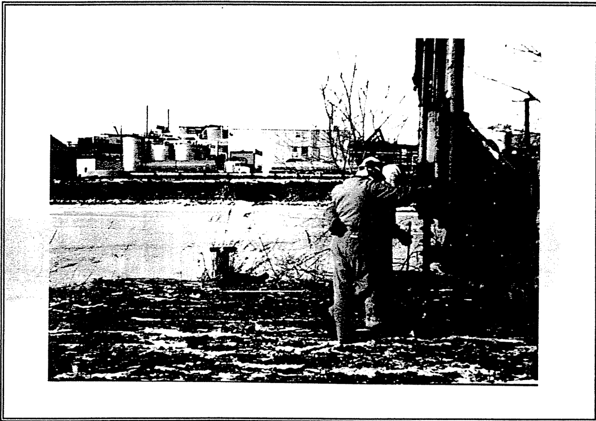
DESCRIPTION: Borehole B-12
