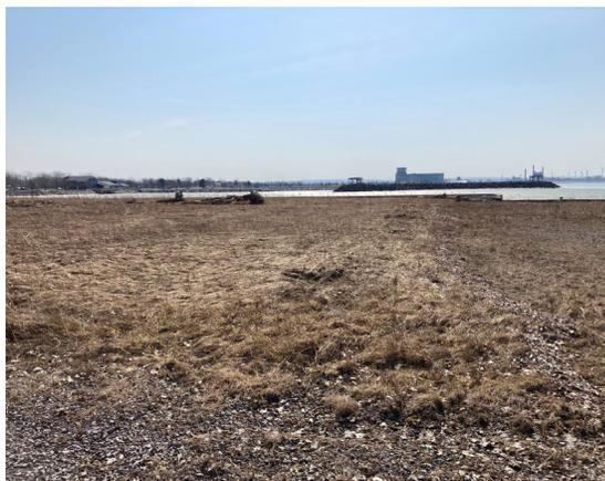
Photo 1: Cover system in the southeastern portion of the Site. Erosion rill repaired with large over-sized stone in 2020 to allow surface water runoff is still intact, looking south.
